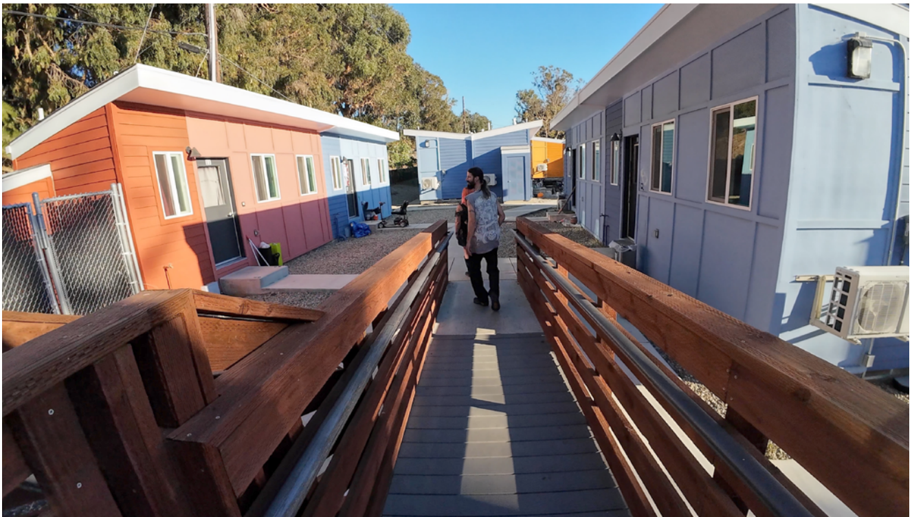
Fairmont Navigation Center, San Leandro
