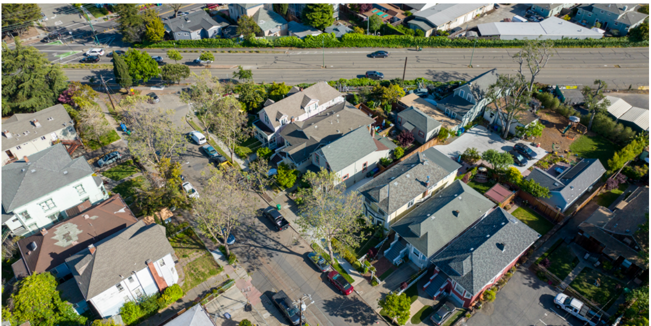
Residential neighborhood, Alameda County
