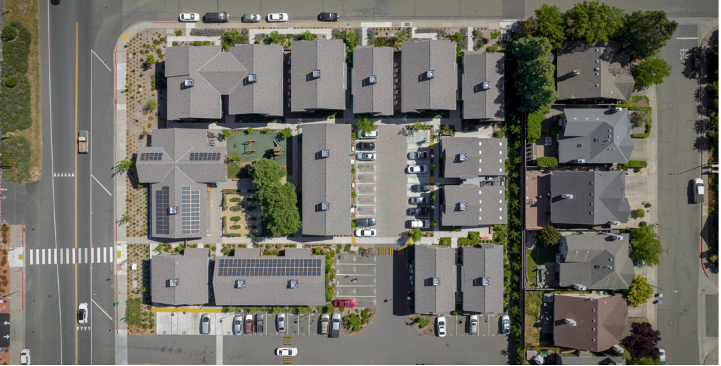
Residential housing, Sonoma County Photo: Karl Nielsen
