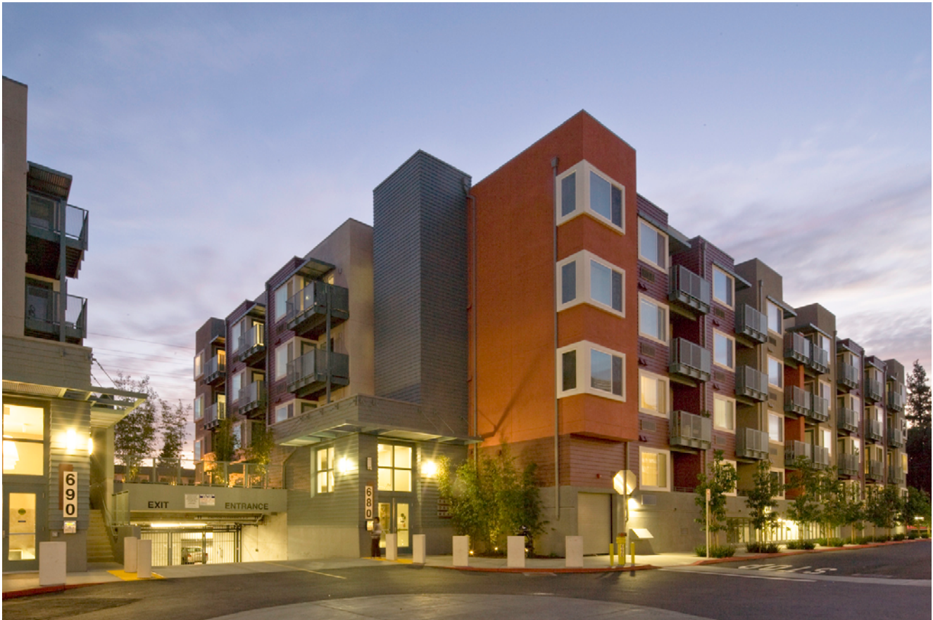
Fair Oaks Plaza apartments, Santa Clara County
