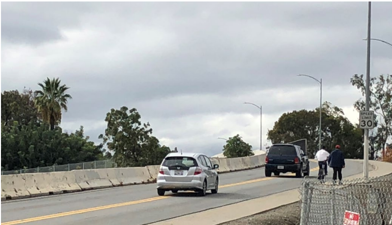
Taylor Street Overcrossing
