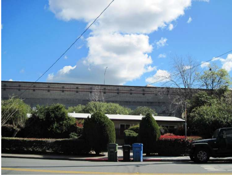
Figure 2.1.9-7. Key View 3 Photograph of Existing Conditions (July 6, 2021)
