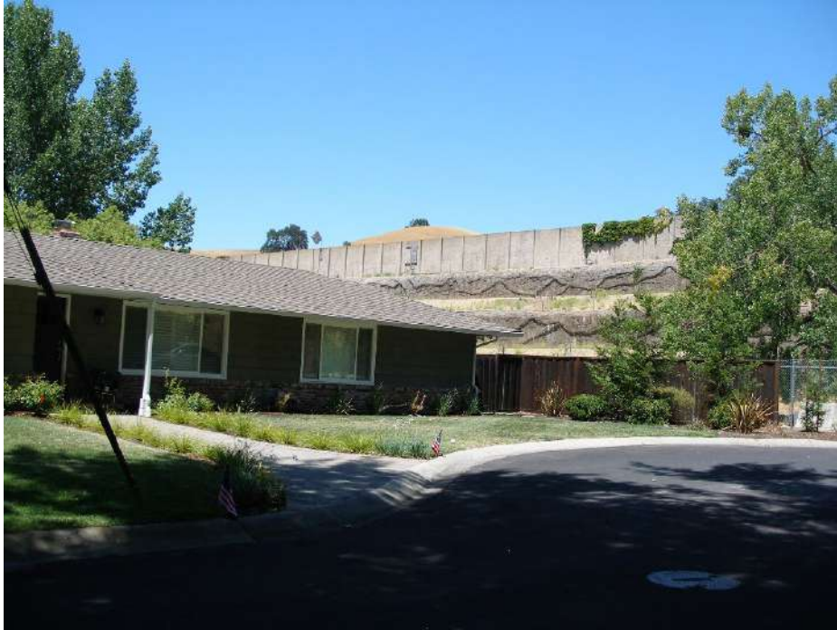
Figure 2.1.9-3. Key View 1 Photograph of Existing Conditions (July 6, 2021)
