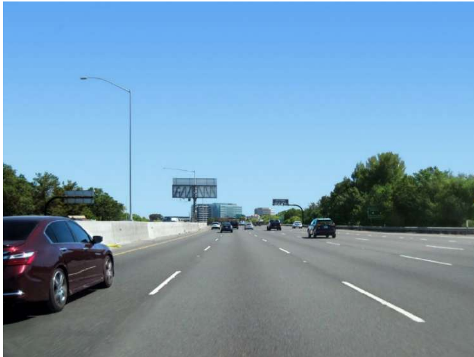
Figure 2.1.9-9. Key View 4 Photograph of Existing Conditions (July 6, 2021)
