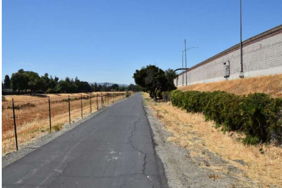
Figure 2.1.9-15. Key View 7 Photograph of Existing Conditions (July 6, 2021)
