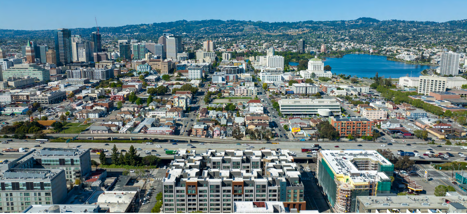
New housing, Oakland Photo: Karl Nielsen
