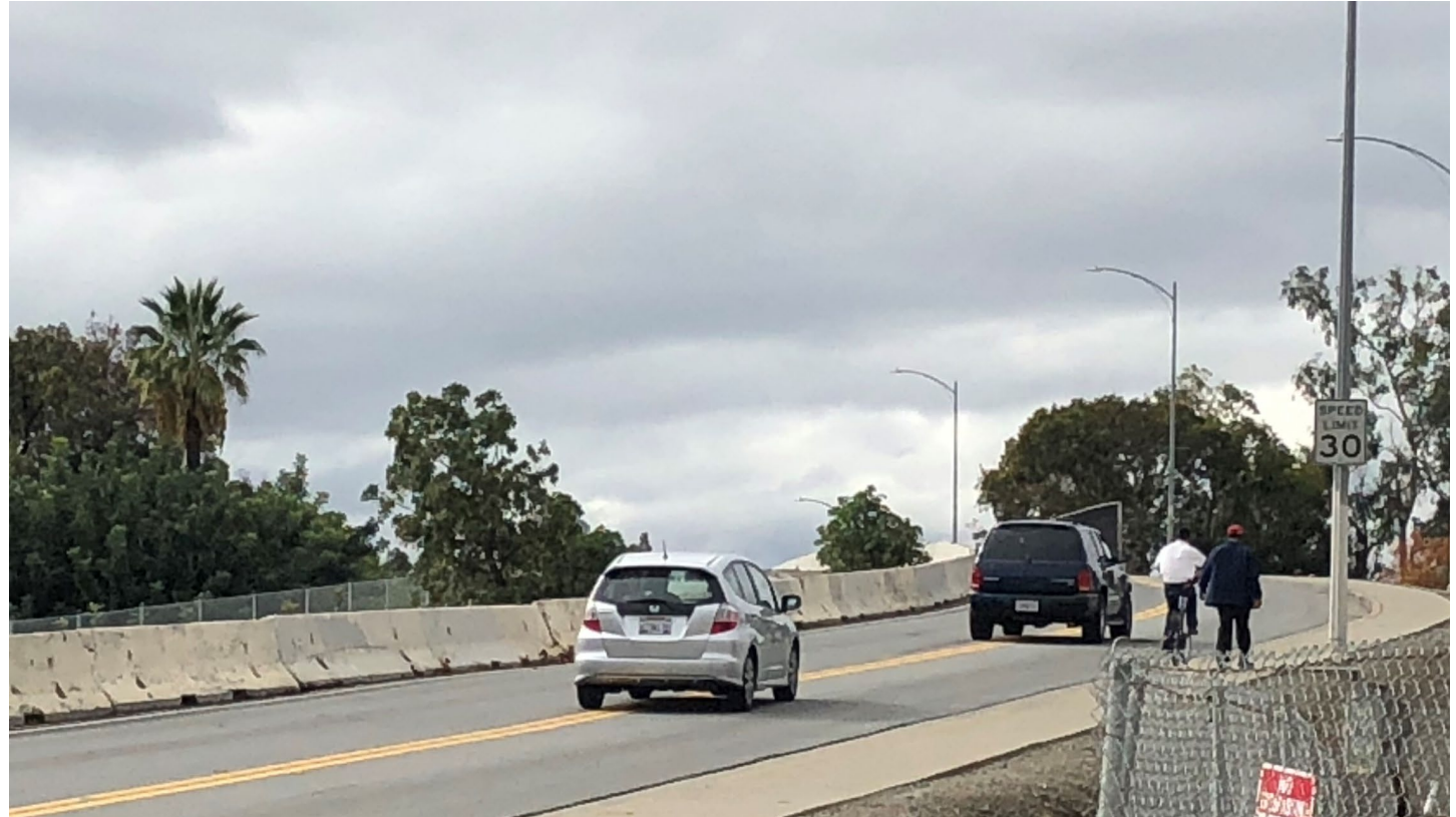
Taylor Street Overcrossing
