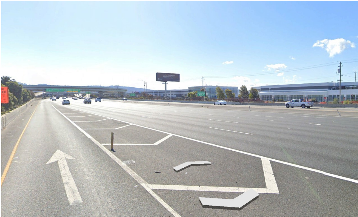
Photo 1. Looking southeast toward the Link project area from the Bay Bridge Toll Plaza. Source: Google Earth
