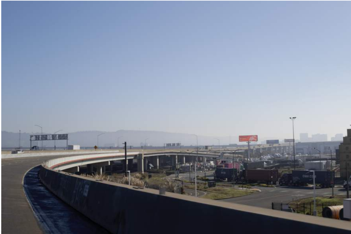
Existing Conditions. View eastward from I-80.
