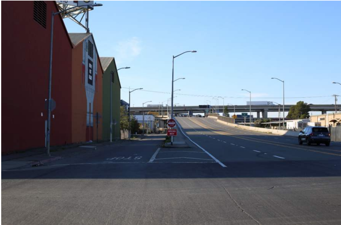
Existing Conditions. View of warehouse on West Grand Avenue alley.
