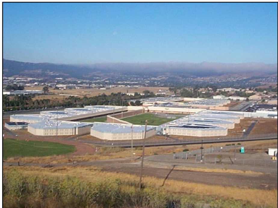
Solar Installation at the Santa Rita Jail consists of nearly 3 acres of Power-Light's roof top PV tiles.
