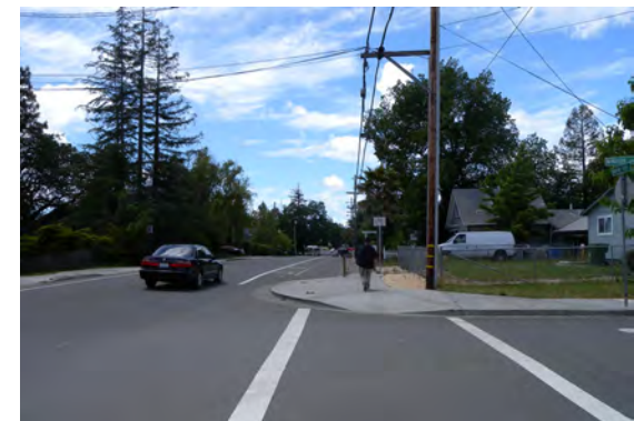
The Town currently requires utilities to be undergrounded as part of a subdivision project. Undergrounding has occurred in the Downtown core (top), but not in all of the surrounding neighborhoods (middle and bottom).
