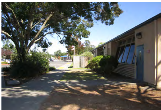
Windsor High School (top and middle) and Windsor Creek Elementary School (bottom) are located within the Planning Area.
