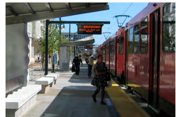
Transit stops should incorporate amenities such as benches, shelter, and next-bus updates.
