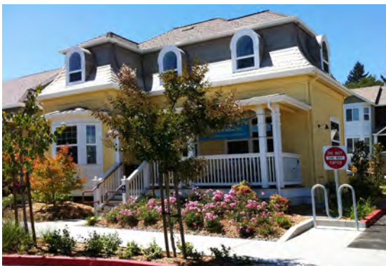
Large retail establishments should be multi-storied (top) and should consider features such as arcades to improve pedestrian friendliness (middle). Residential buildings converted to office should retain their residential character (bottom).
