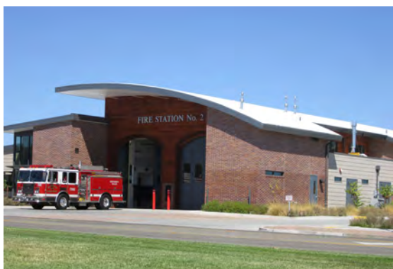
The Police Station (above) is located in the Civic Center and Fire Station #2 (middle and bottom) is located at the southern edge of the Planning Area.
