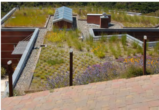
Consider permeable pavers for new paving areas (top), installation of solar panels (middle), and green roofs (bottom).
