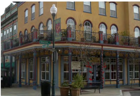
Landscaping should include amenities such as bike racks and benches (top) and climate appropriate and drought-resistant landscaping (middle). Street furniture existing in Downtown Windsor adds to the pedestrian realm and improves walkability (bottom).
