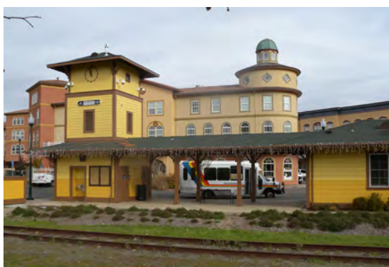
The Windsor Station Area/Downtown Specific Plan extends the Downtown core with a “town green loop” strategy, and aims to promote transit oriented development and a vibrant, walkable, and well-connected Downtown.
