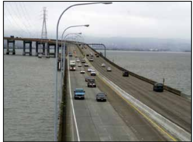
High-Rise Section of San Mateo-Hayward Bridge
