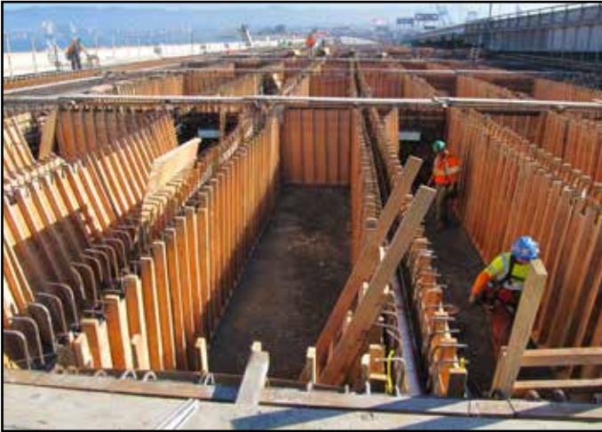
Oakland Touchdown #2 Eastbound Stemwall Formwork
