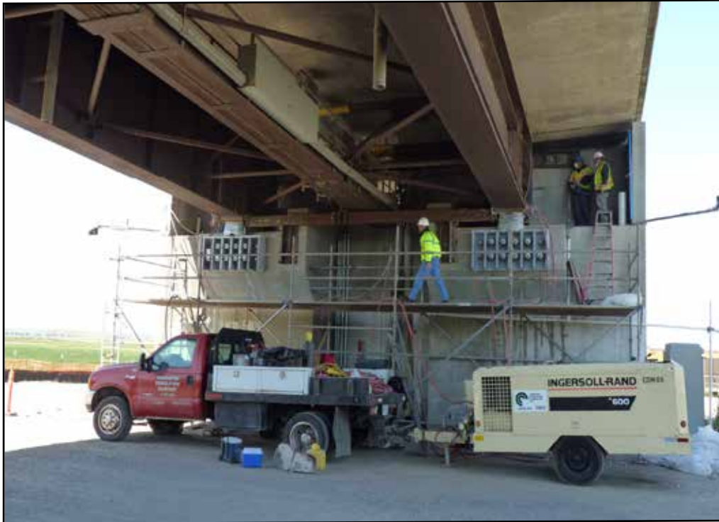
Antioch Bridge - Pier 41 Girders on Temporary Jacks prior to Installation of Isolation Bearings
