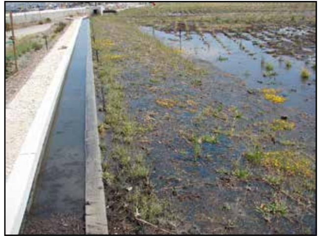
Stormwater Retention Basin
