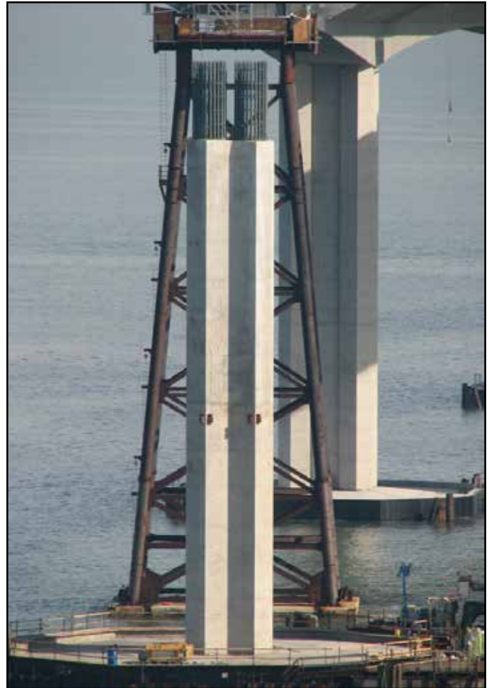
SAS Marine E2 Foundation and the Skyway Westbound Column
