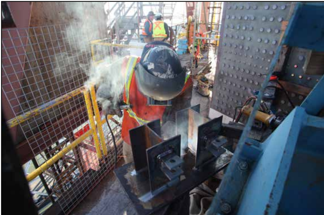
Self-Anchored Suspension Bridge Welding A Pipe Support at the Tower Head
