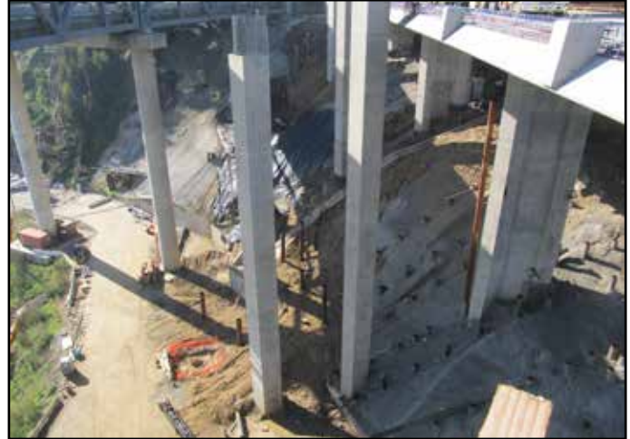
YBITS Structure Eastbound On-Ramp Columns
