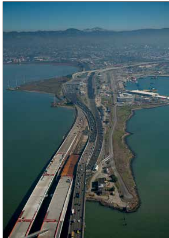
Aerial View of the Eastbound Oakland Touchdown #2 Construction Progress
