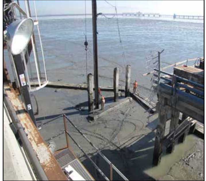
Ravenswood Pier Pile Removal
