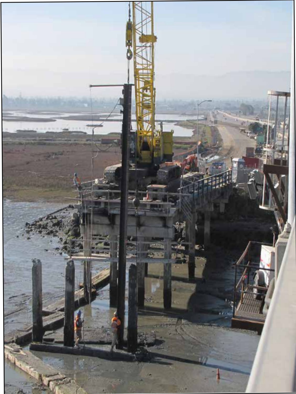
Ravenswood Pier Demolition
