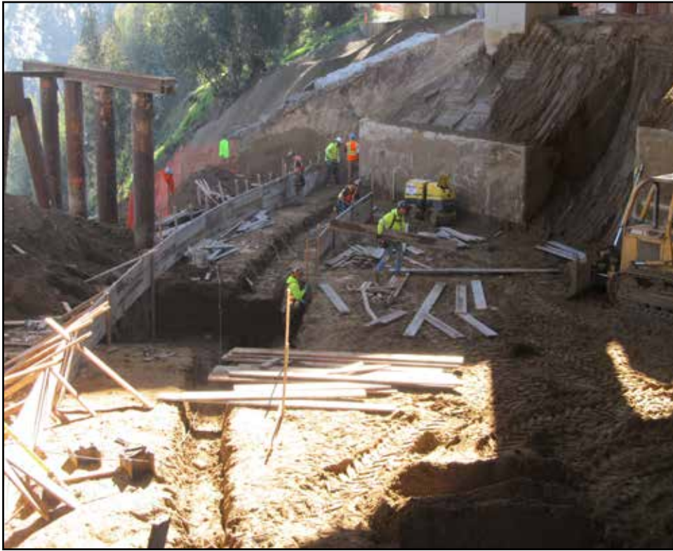
YBITS # 1 Retaining Wall #50
