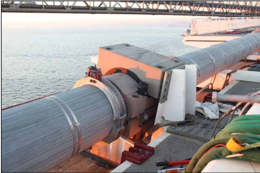
Self-Anchored Suspension Bridge Cable Band Bracket in Place at South Mainspan
