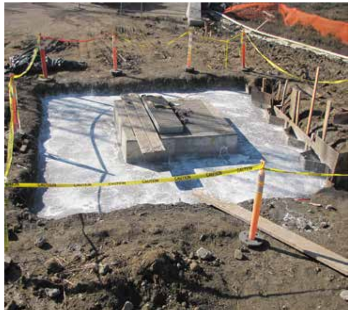
Repair to Settling Junction
