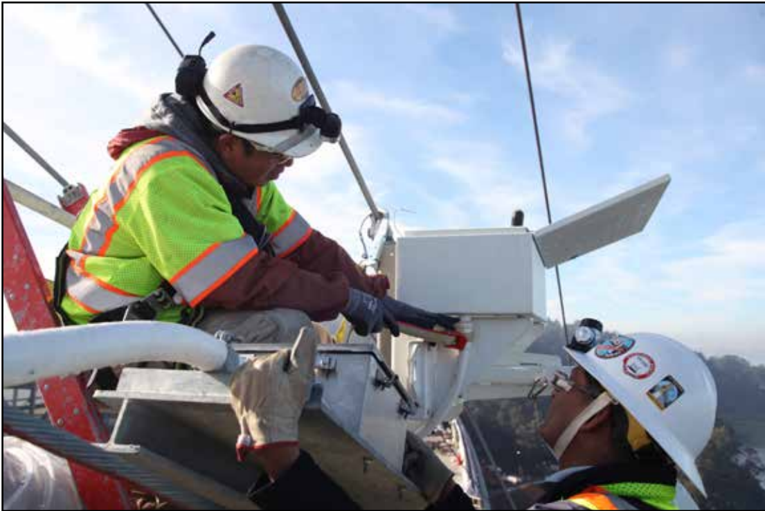
Self-Anchored Suspension Bridge Light Fixtures Installation
