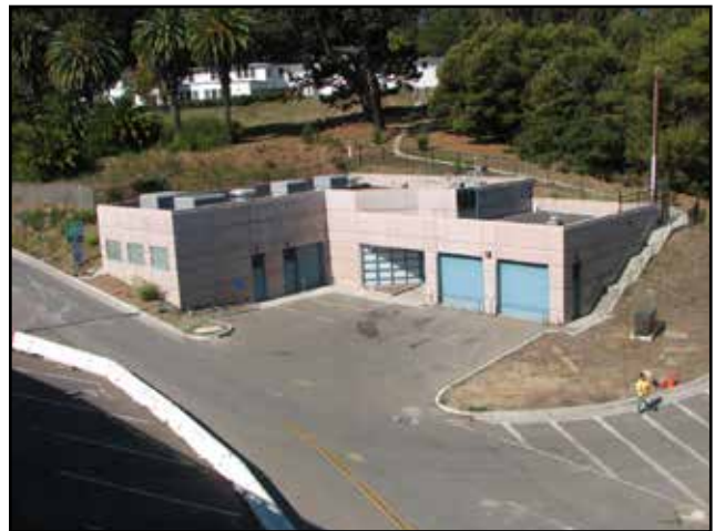
New YBI Electrical Substation
