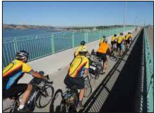
Benicia-Martinez Bridge Bicycle/Pedestrian Path
