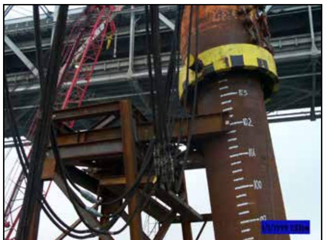
Battered Pile Installation Demonstration
