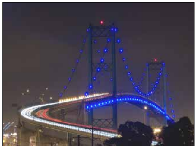
Los Angeles-Vincent Thomas Bridge
