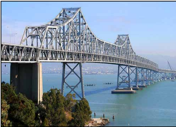
Existing San Francisco-Oakland Bay Bridge Cantilever Section to be Dismantled as Part of the YBITS #2 Contract
