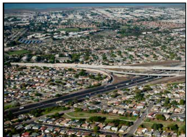
Aerial View of Completed 880/92 Interchange Project
