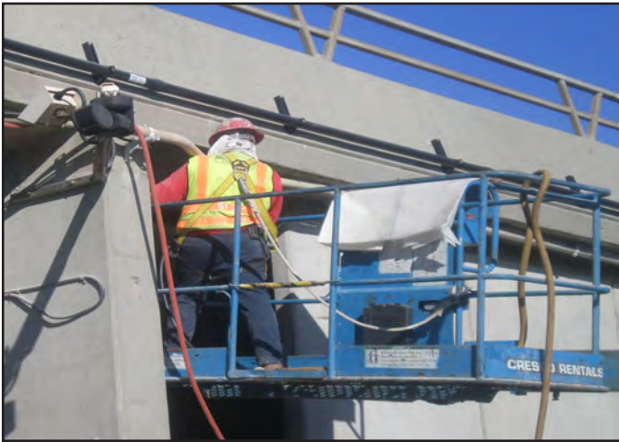
Dumbarton Bridge - Concrete Removal Operation at East Approach Slab
