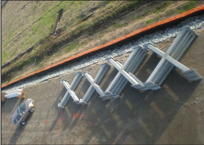
Antioch Bridge - Steel Cross Bracing Delivered to Site
