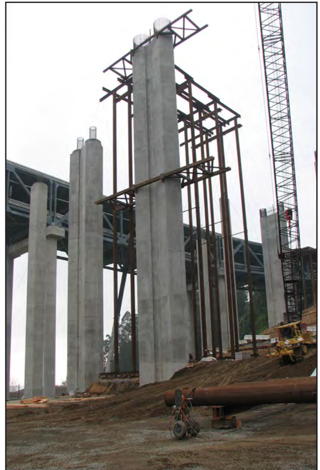
Yerba Buena Island Transition Westbound Falsework
