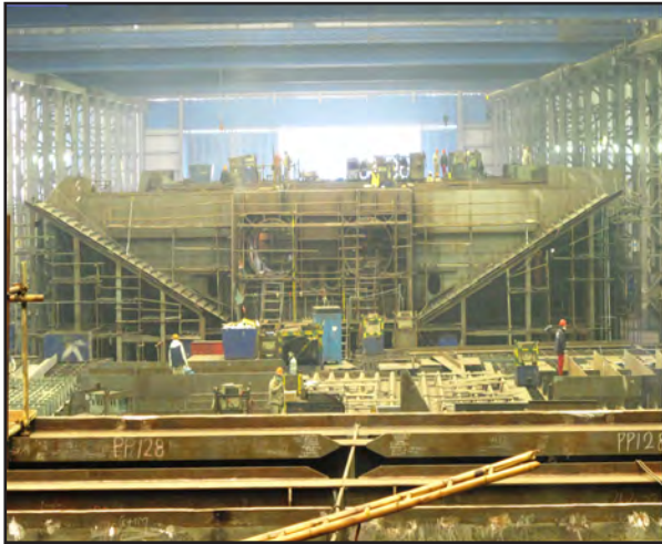
Looking East at 14 East
