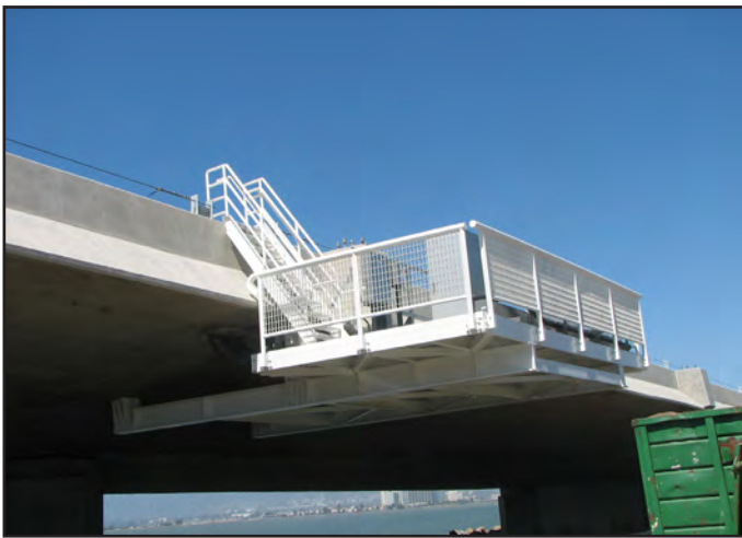
Oakland Touchdown Service Platforms Installed
