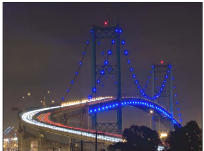
Los Angeles-Vincent Thomas Bridge
