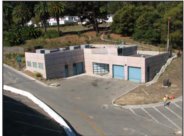
New YBI Electrical Substation
