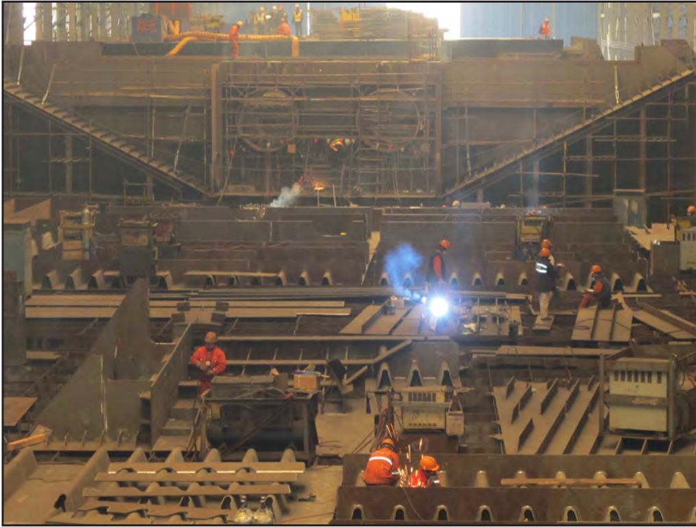
Roadway Box 14 in Sub Assembly
