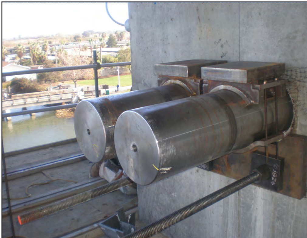
Jacking Pins at Pier 7 Prior to Setting Jacks
