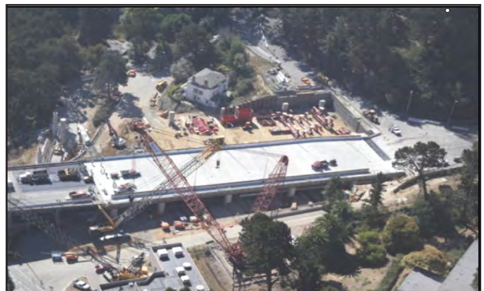
West Tie-In Phase #1 Rolled in on Labor Day 2007
