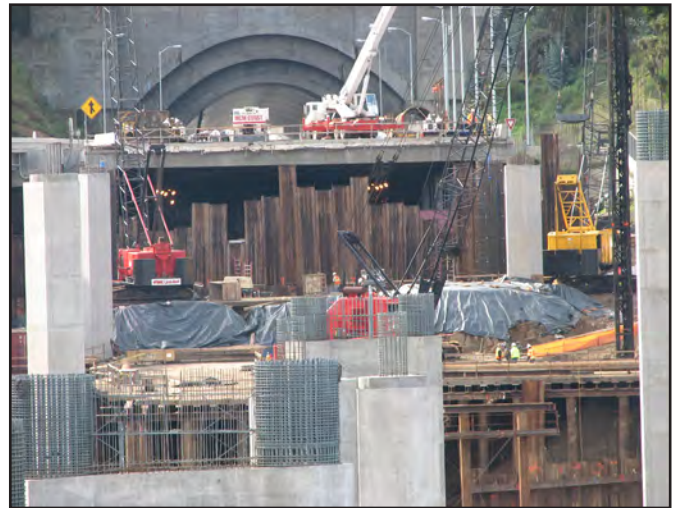
YBITS #1 Access Trestle and Footing Shoring
