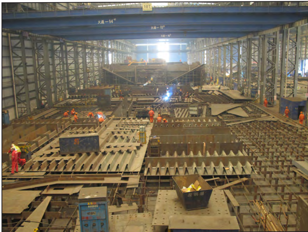
Roadway Boxes 13 and 14 in Fabrication at ZPMC
