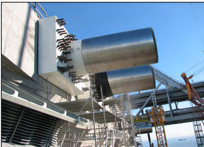
Hinge K Pipe Beams on Pier W2
