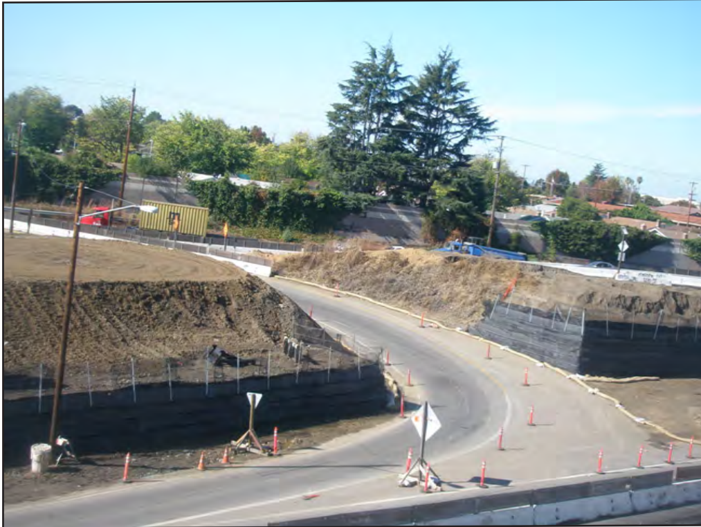
GRE Work in Progress at Southwest Quadrant of the 92/880 Interchange
