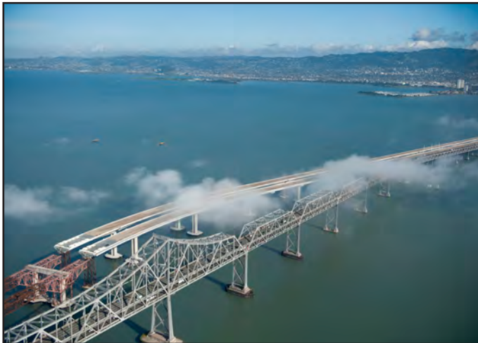
The Existing Bridge on right and Completed Skyway on left Looking East toward Oakland
