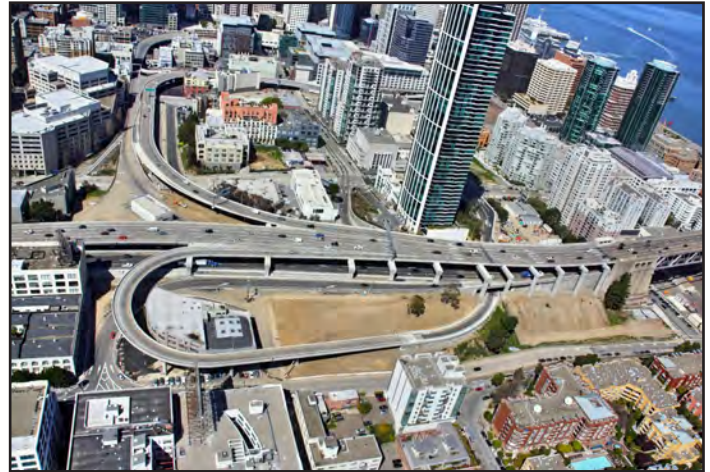
West Approach Overview
