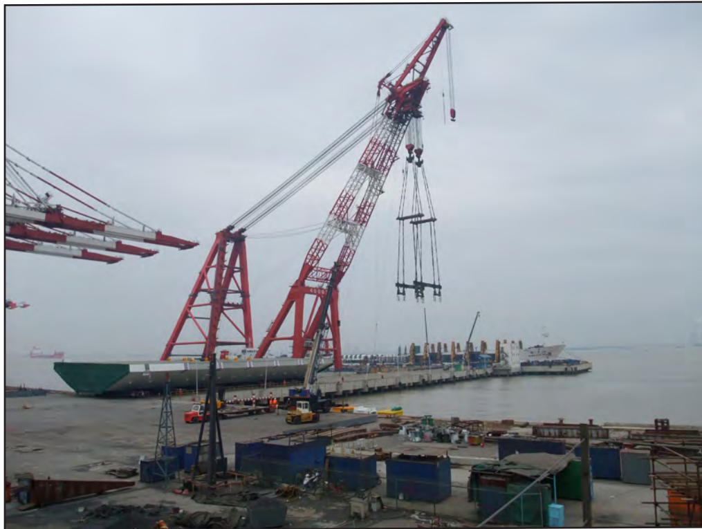
Roadway Boxes Being Prepared for Loading onto the Ship at ZPMC Heavy Duty Dock in China
