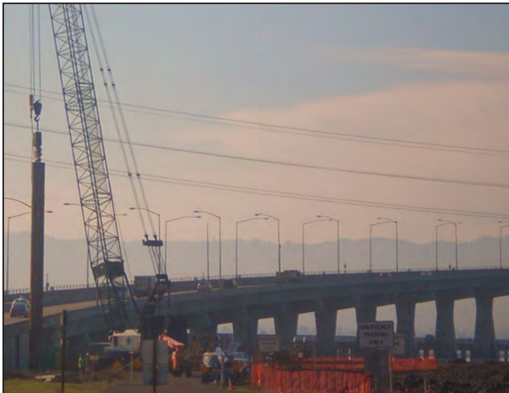
Crane Positioning 48-inch Pile at East Approach Prior to Driving Pile
