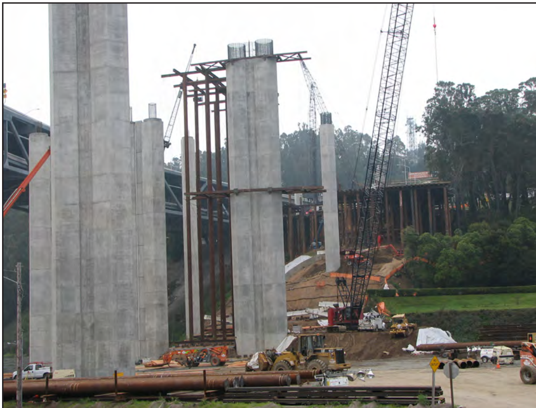
Yerba Buena Island Transition Structures #1 Contract Falsework and Trestle Erection
