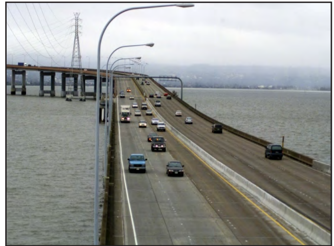
High-Rise Section of San Mateo-Hayward Bridge
