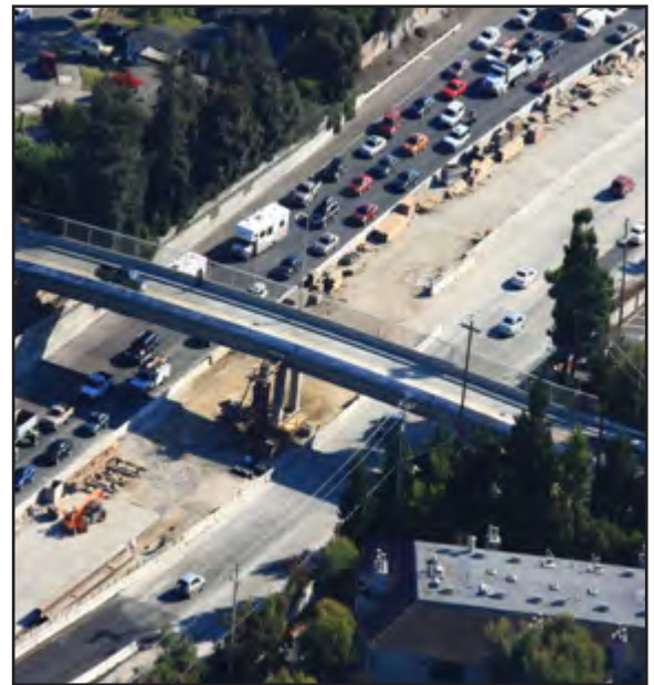
Calaroga Bridge Work in Progress
