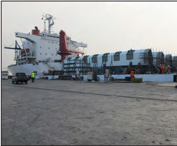
Tower Lift 4 Loaded onto Ship
