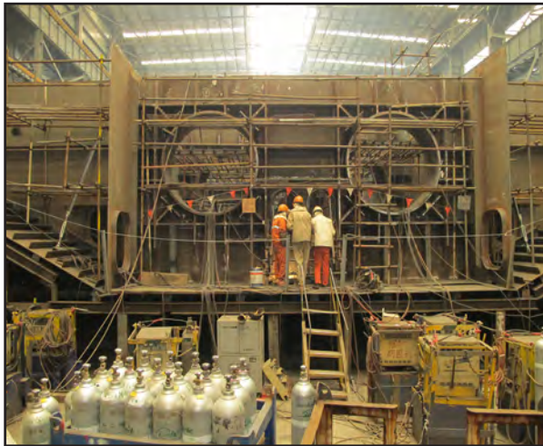
Roadway Box Lift 14
