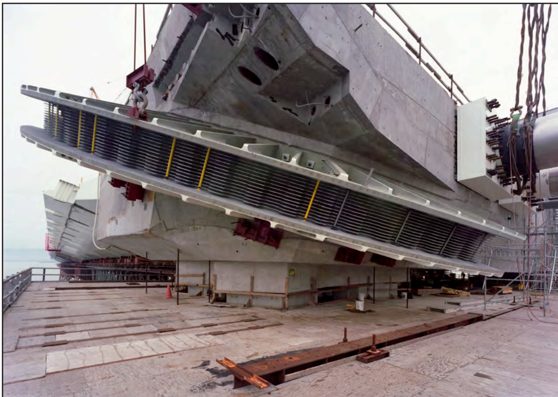
West Deviation Saddle Erected on W2
