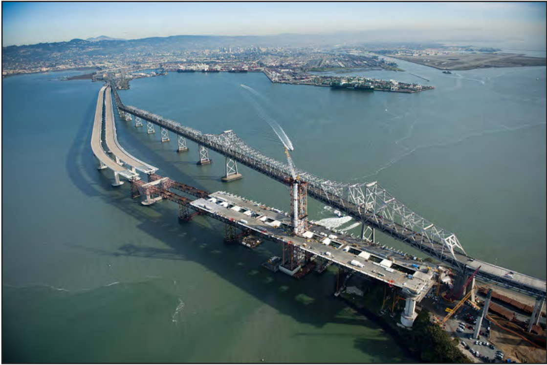
Overview of Progress of Roadway Boxes and Tower Lift 3 Partially Erected
