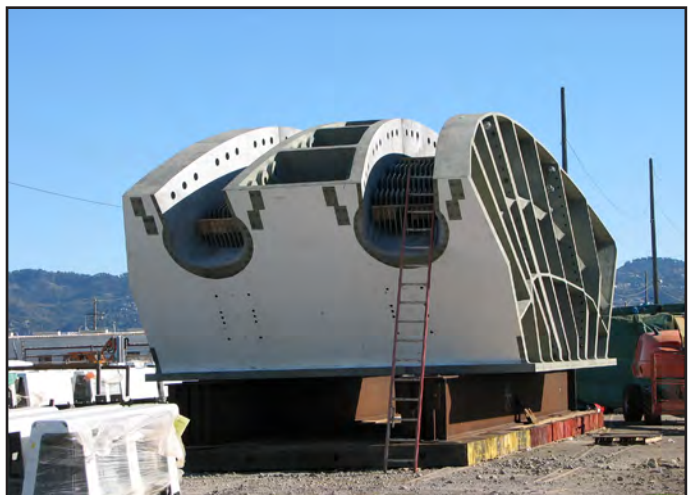
Tower Saddle Fabricated and on Site
