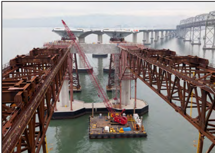
Temporary Support Structures with E2 Cap Beam and Completed Skyway in background
