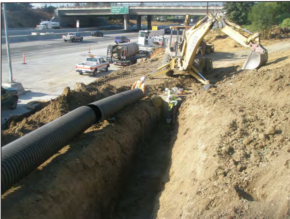
Drainage Works on the Old Hesperian Off Ramp
