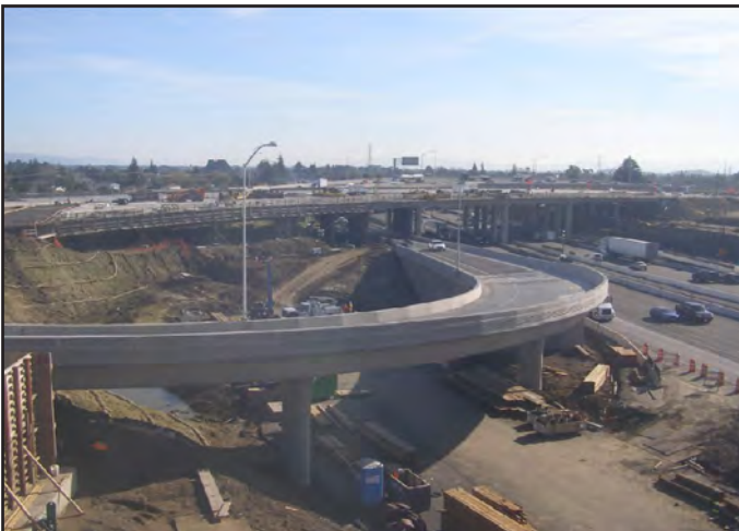
92/880 NWCONN Bridge Construction in Progress
