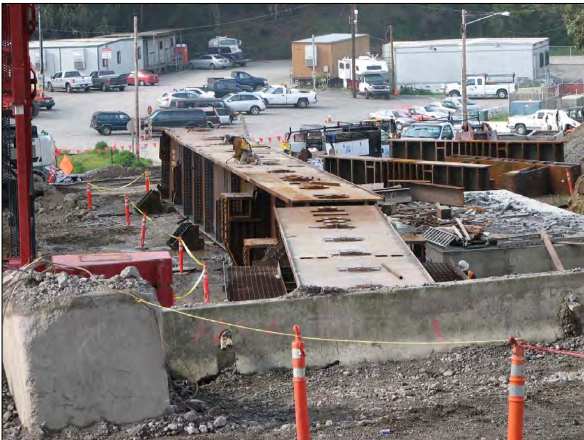
Skid Beams A1 and A2 Disassembled
