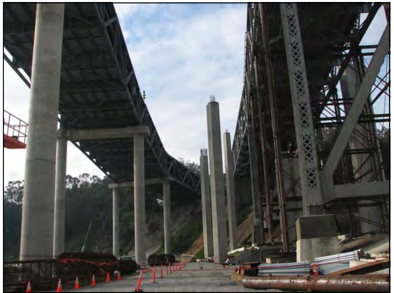
Yerba Buena Island Transition Structure Columns W6 and W7 Looking West
