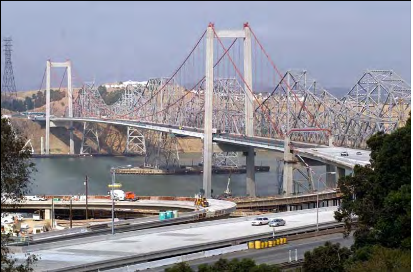
New Alfred Zampa Memorial (Carquinez) Bridge Soon after Opening to Traffic, with Crockett Interchange Still under Construction
