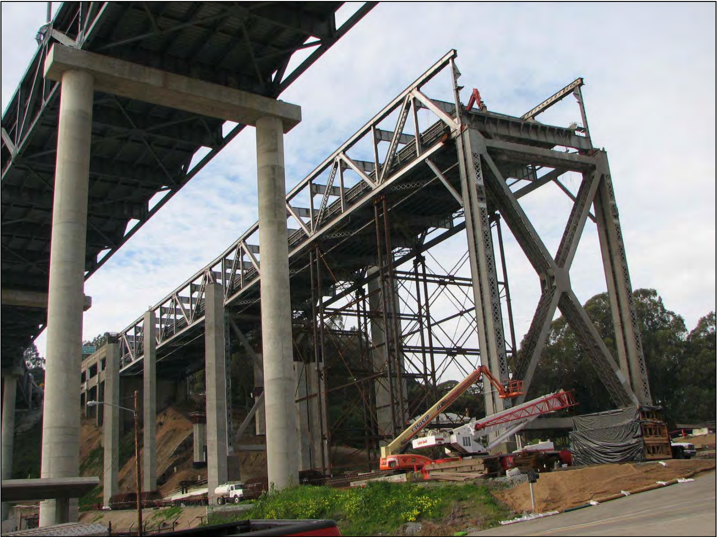
Demolition of Existing Bridge Spans YB2 and YB1
