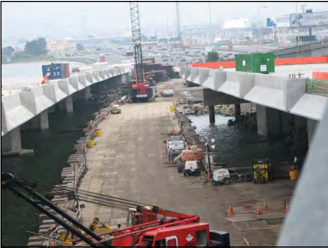
Oakland Touchdown #1 Westbound and Eastbound Overview Looking East
