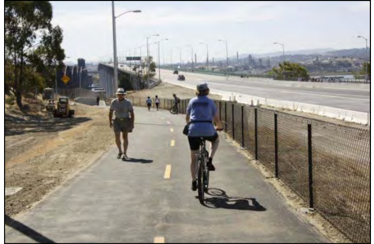
Benicia-Martinez Bridge Newly Opened Pedestrian/Bicycle Pathway
