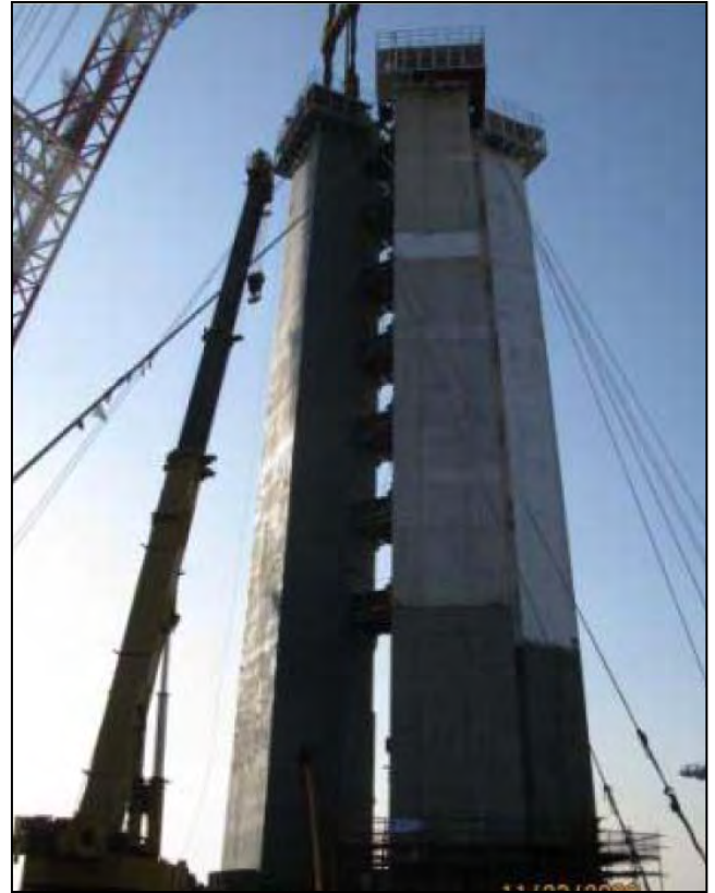
SAS Tower Lift1 East and West Shaft Placed onto the Base Plate during Trial Assembly on the Heavy Duty Dock
