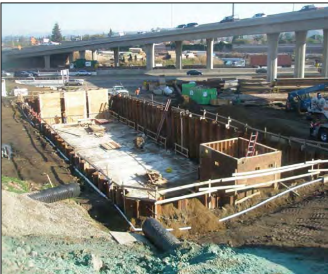
92/880 Pump Station Construction in Progress
