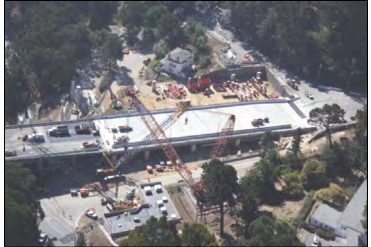
Successful Labor Day Weekend 2007 Roll-In Structure to the Tunnel
