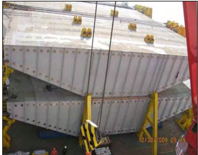
SAS OBG Lifts 1-4 East and West Loaded on Ship
