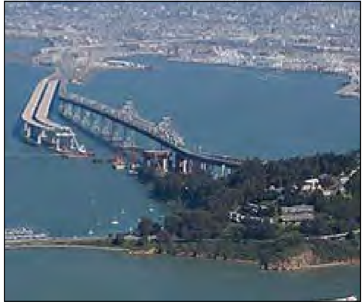
Completed Skyway Left of Existing East Span
