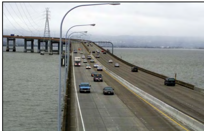
High-Rise Section of San Mateo-Hayward Bridge
