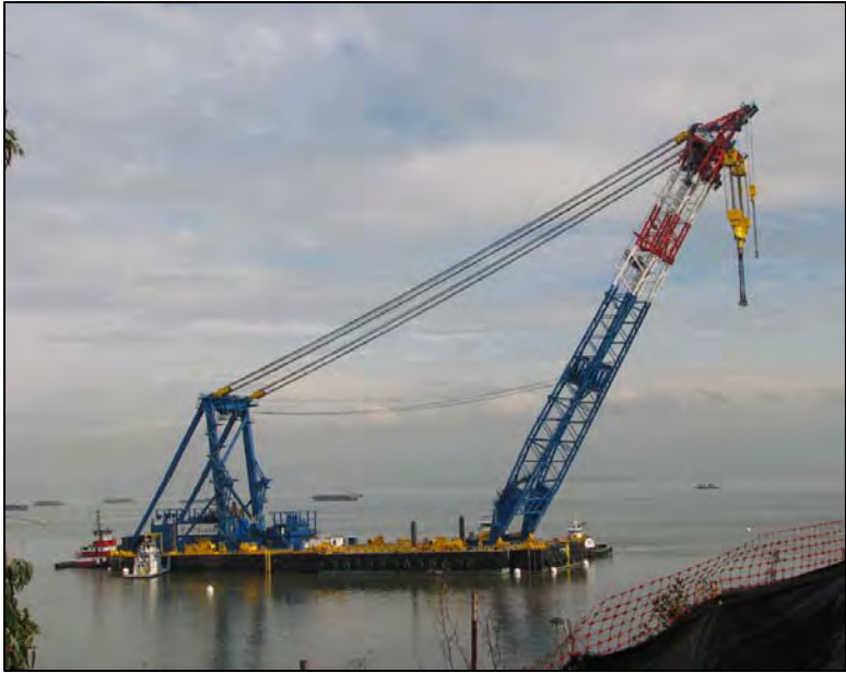
Shear-Leg Barge Crane
