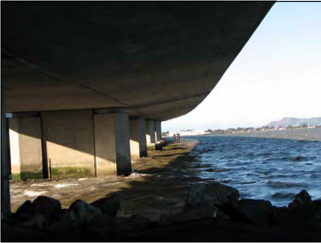
Oakland Touchdown #1 Westbound Falsework and Piles Removed
