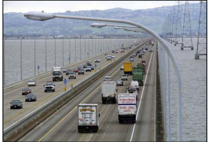
Widening of the San Mateo-Hayward Bridge Trestle on Left
