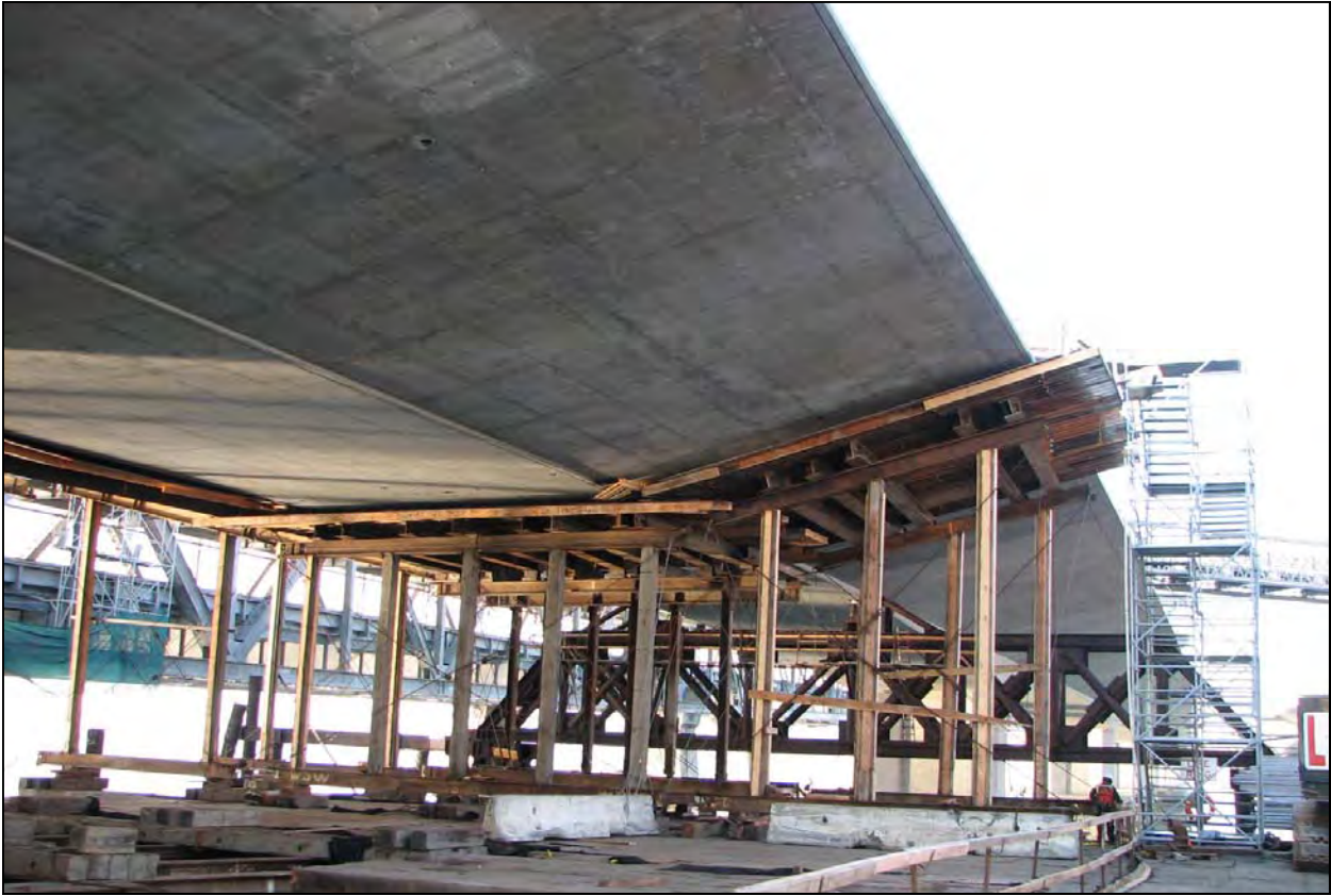
Oakland Touchdown Falsework Removal
