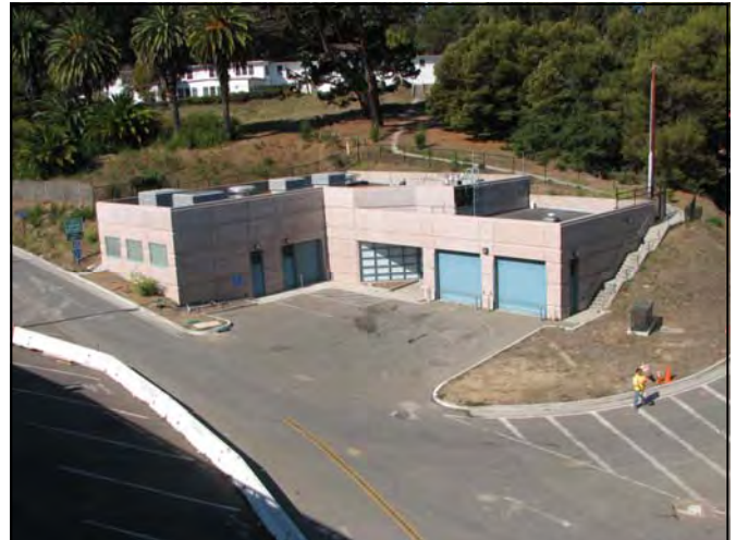
New YBI Electrical Substation
