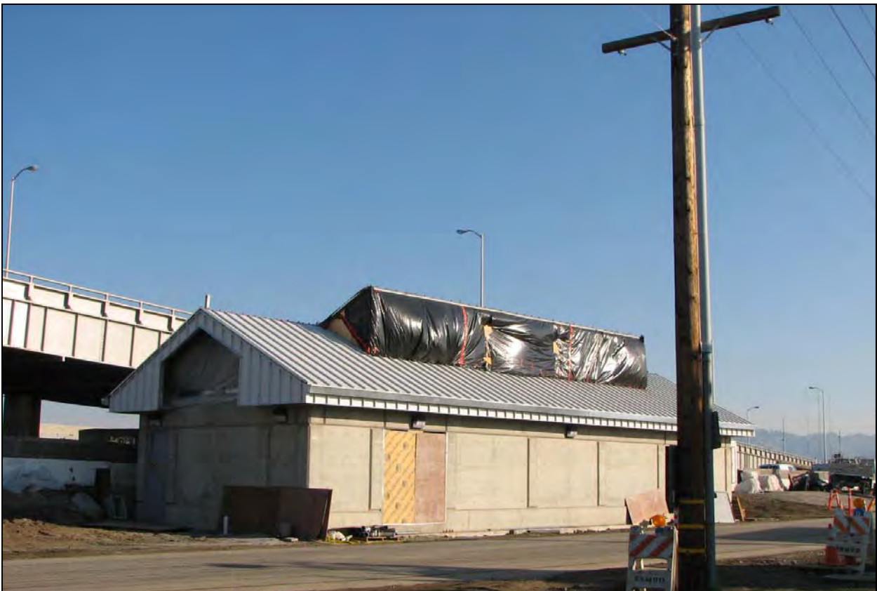
Oakland Touchdown Mole Substation Exterior View
