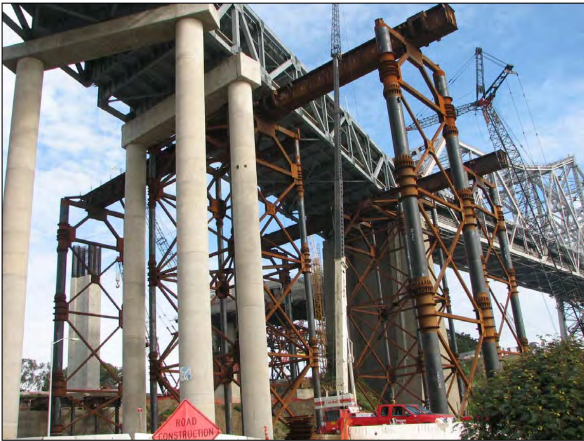
Skid Bent System Disassembly in Progress
