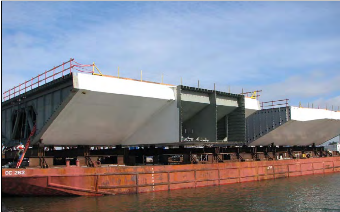
SAS - OBG Lifts 3 and 4 Stored onto the Barge
