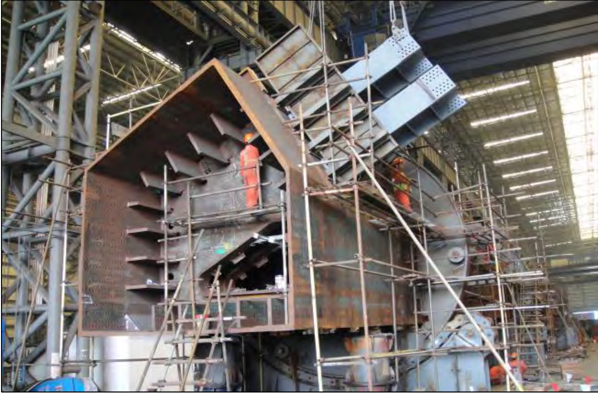
SAS Tower Lift 2 North Shaft Being Fabricated in Bay 10
