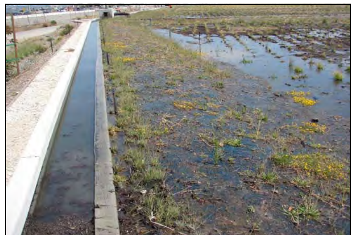
Stormwater Retention Basin
