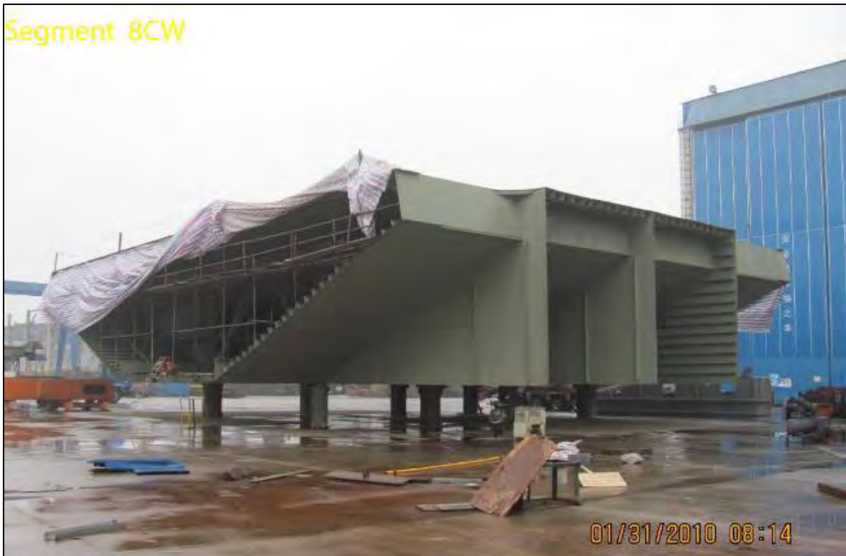
SAS Lift 8CW Being Prime Coated
