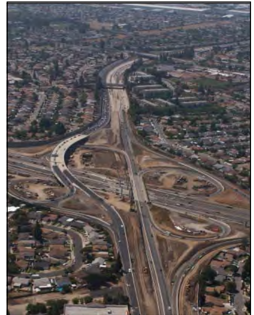
Overview of Progress to Date
