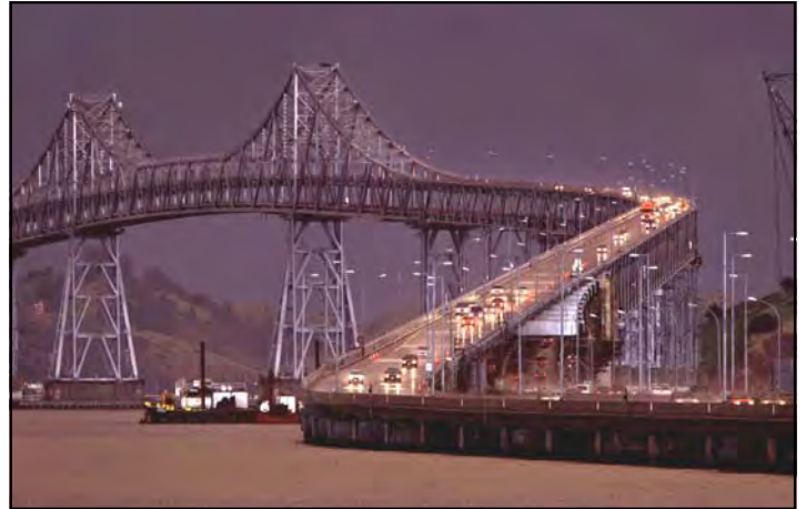
Richmond-San Rafael Bridge
