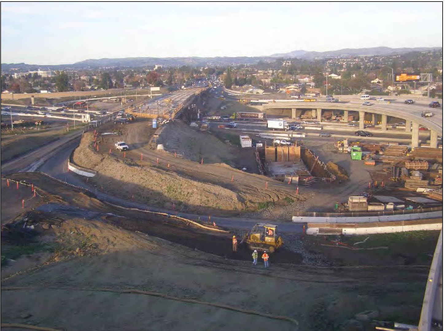
92/880 Site Preparation of New Route 92 and Interstate 880 Separator
