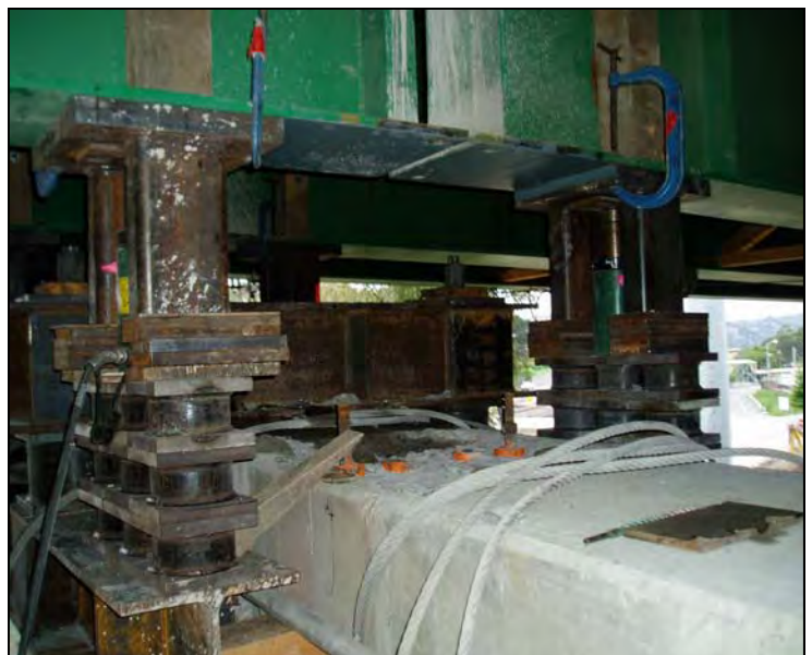
Mococo Road Bridge Jacking
