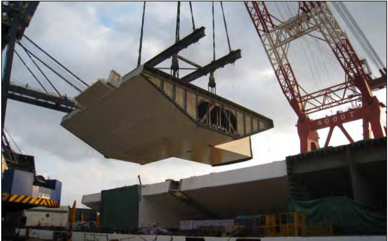
SAS OBG Lift 3W Being Loaded onto the Ship
