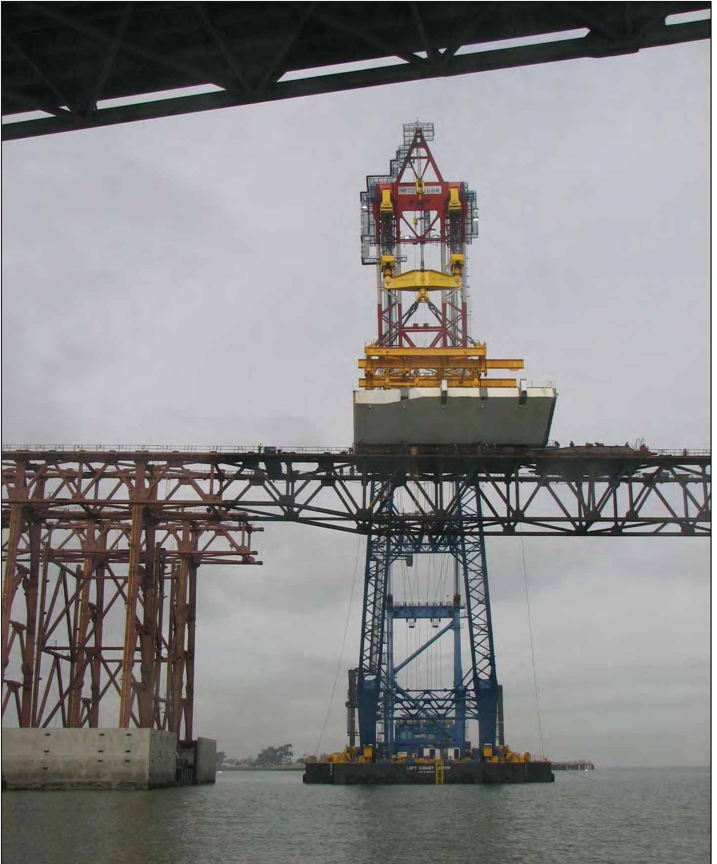
SAS OBG Lift 1E Placed on top of Temporary Eastbound Structure
