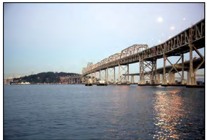
Existing East Span of Bay Bridge
