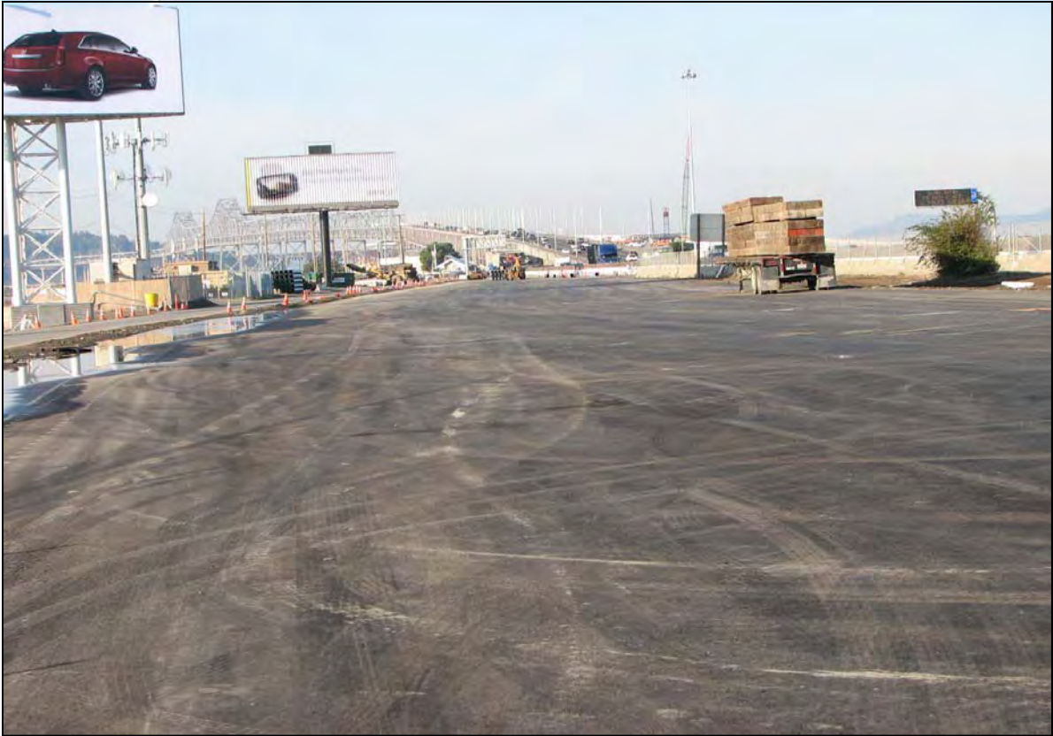
Oakland Touchdown Eastbound Detour Road Paved
