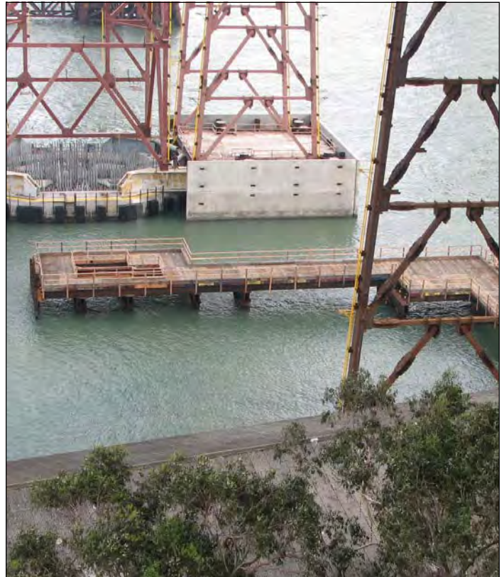
SAS T1 Trestle Construction Overview
