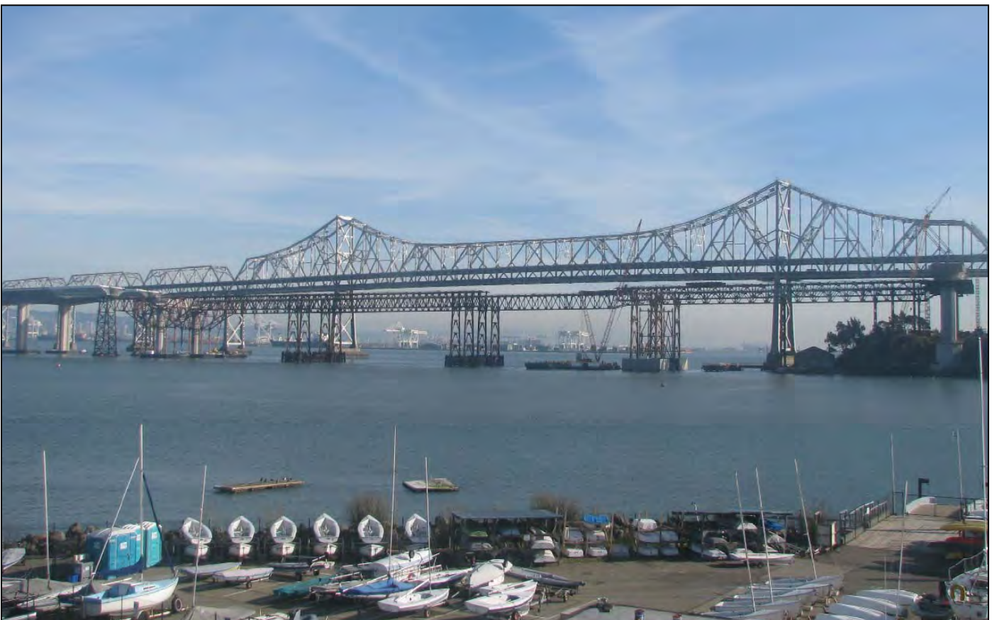
SAS Temporary Support Structures and Existing East Span
