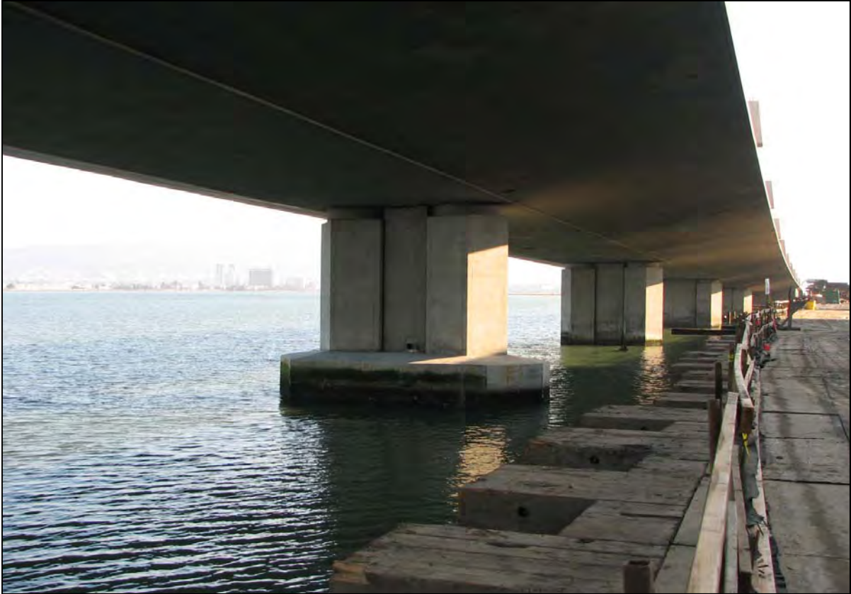
Oakland Touchdown Westbound Falsework Piles Removed
