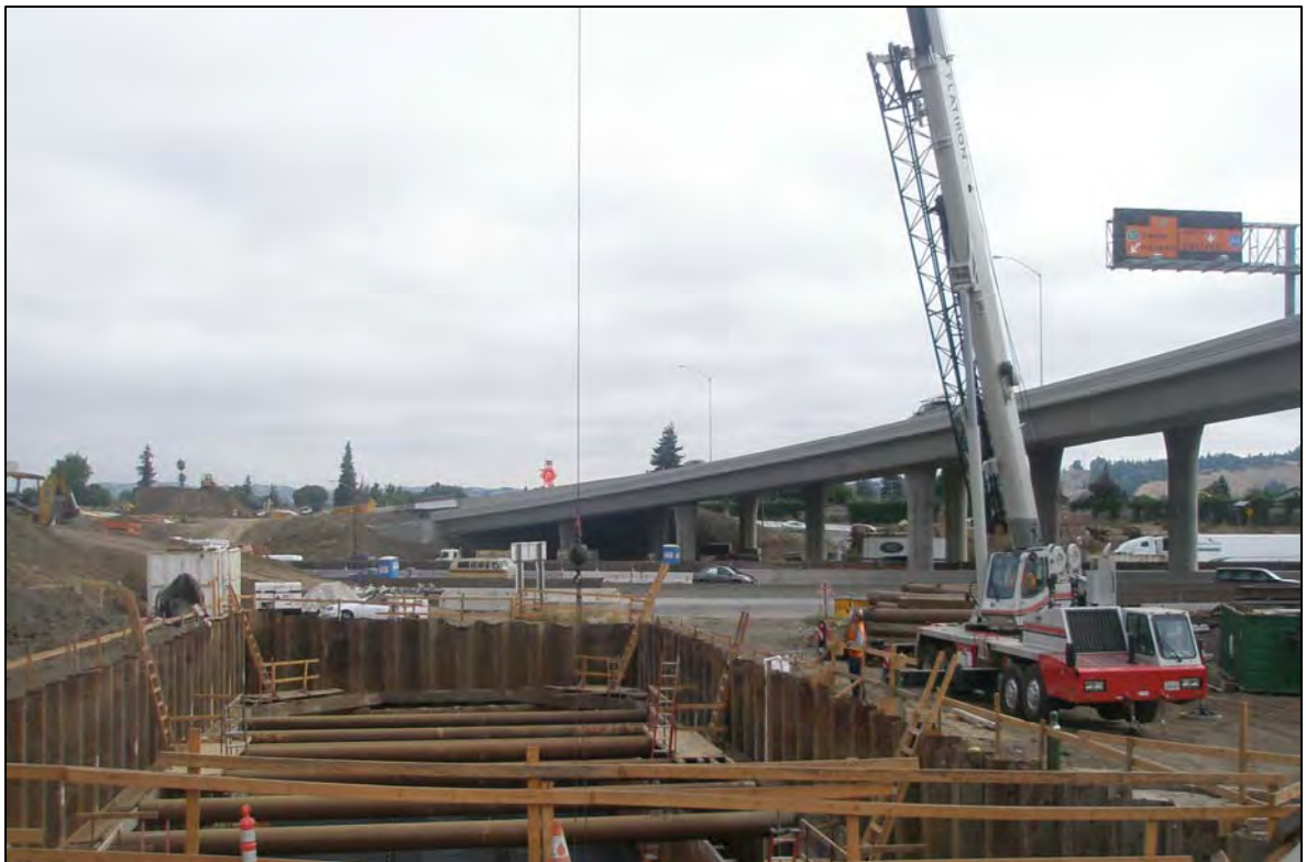
92/880 Pump Station Construction in Progress
