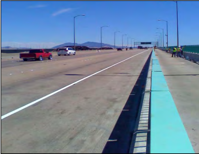
New Pedestrian Bicycle Path on Benicia-Martinez Bridge Under Construction
