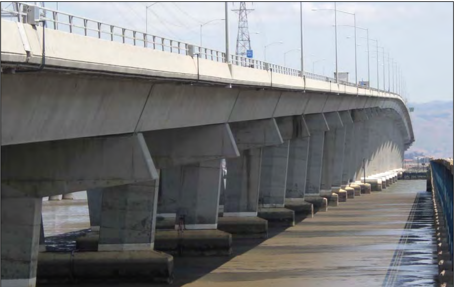
Existing Dumbarton Bridge Looking East toward the Alameda County Foothills
