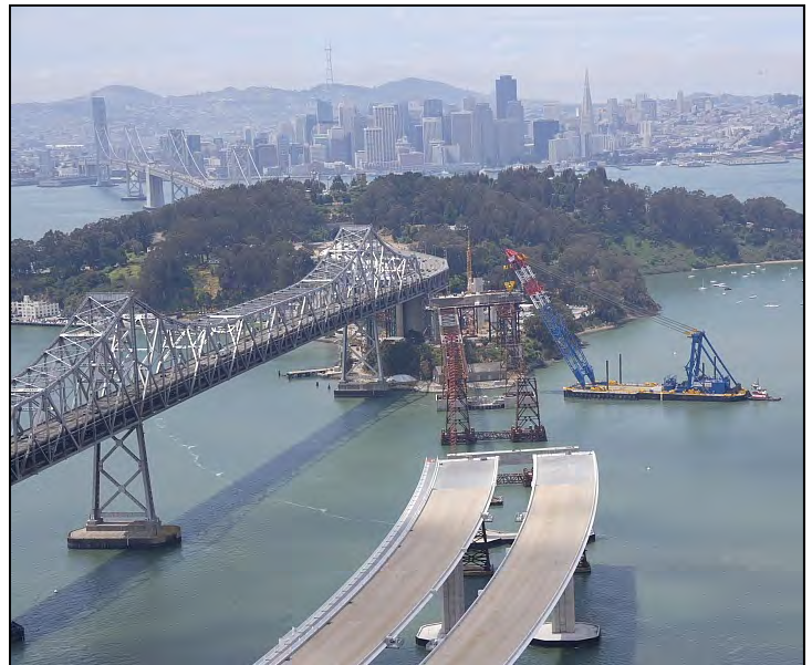
Western End of Completed Skyway
