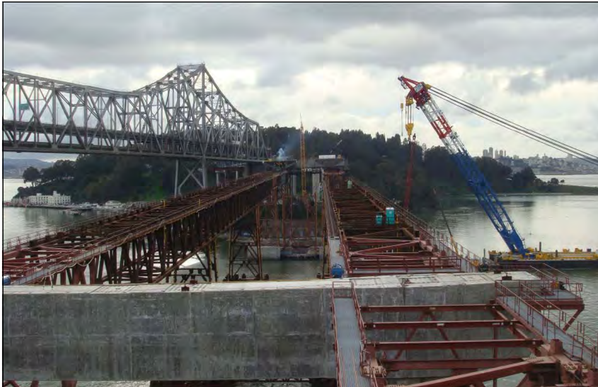
SAS - First OBG Lift 1E Completed
