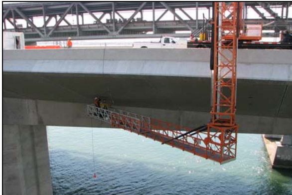
Cormorant Nesting Platform Installation
