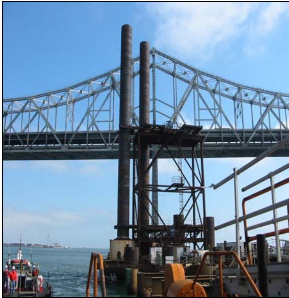
Pile Driving Operations at E2 (one)
