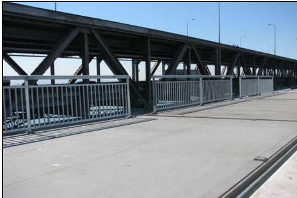
Bike Path Railing for the Eastbound Skyway
