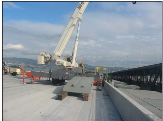
Installation of Bike Path Panel Segments
