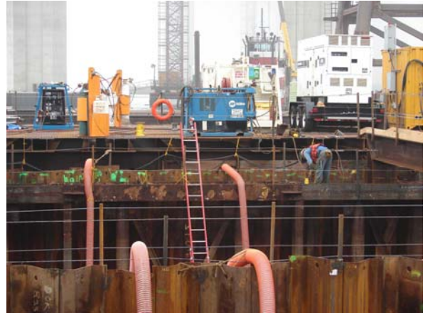
Pumping Water out of Cofferdam at E2
