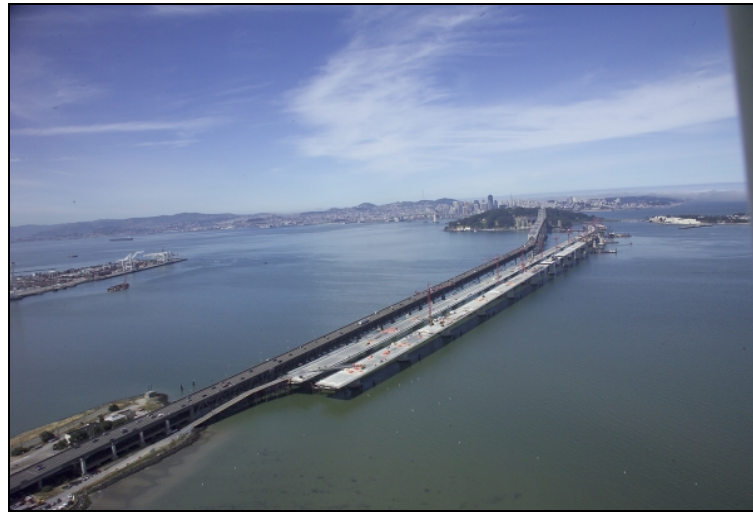
Aerial view of Skyway construction
