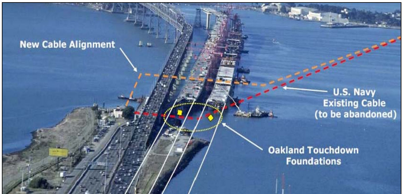
Submarine Cable Relocation
