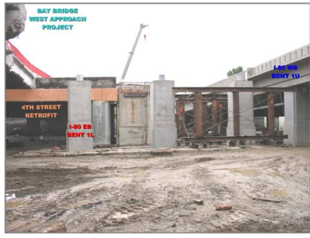
West Approach Progress Photo (four)
