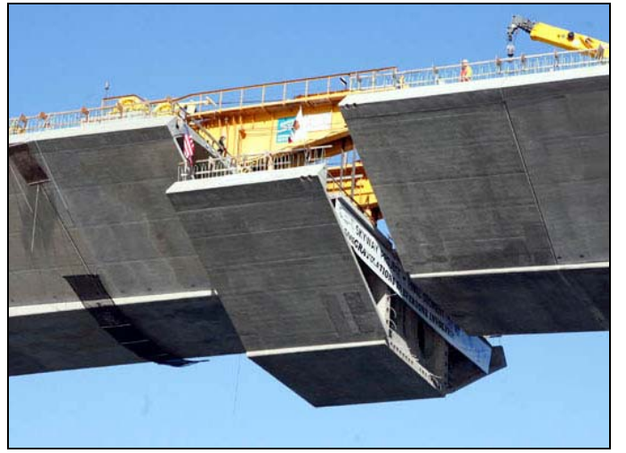
700-ton segment squeezes into place
