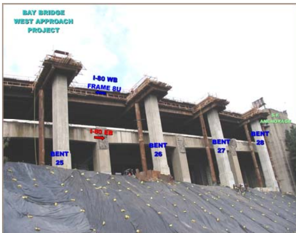
West Approach Progress Photo (five)
