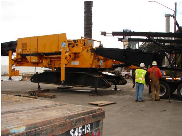
Demobilization of the SSD construction equipment (one)
