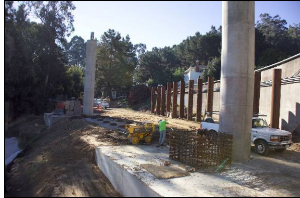
Footing and Pier Columns for Bent 48
