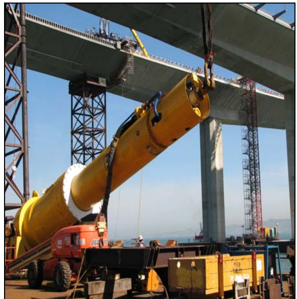
Lifting the Pile Driving Hammer
