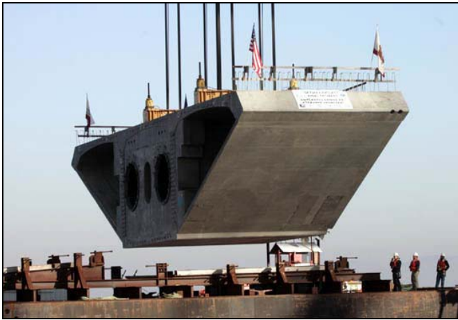
700 ton segment is slowly lifted off the barge
