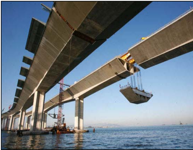
700-ton segments are slowly hoisted into place
