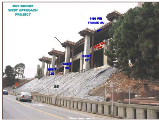
West Approach Progress Photo (six)
