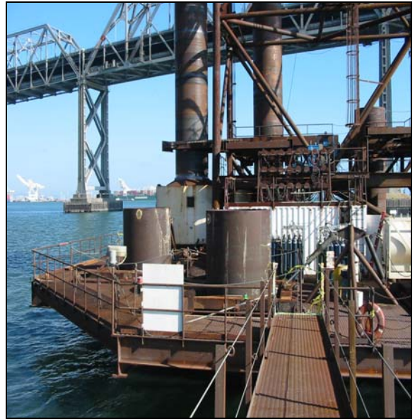
Pile Driving Operations at E2 (two)
