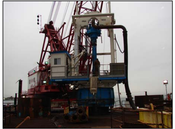
Rock Socket Drilling in Pile # 4 at T1
