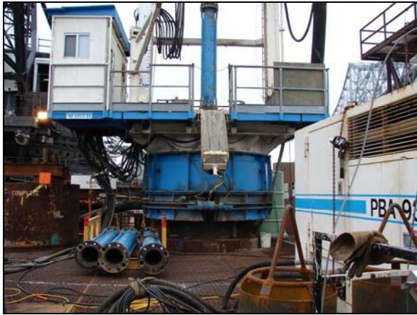
Rock Socket Drilling in Pile # 12 at T1
