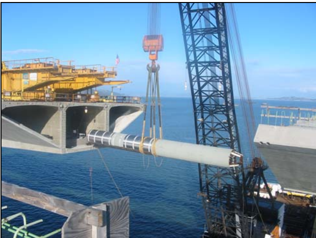
Installing HPB BW
