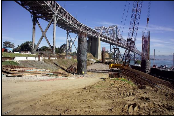
Pier Column Construction for Bents 50 and 51
