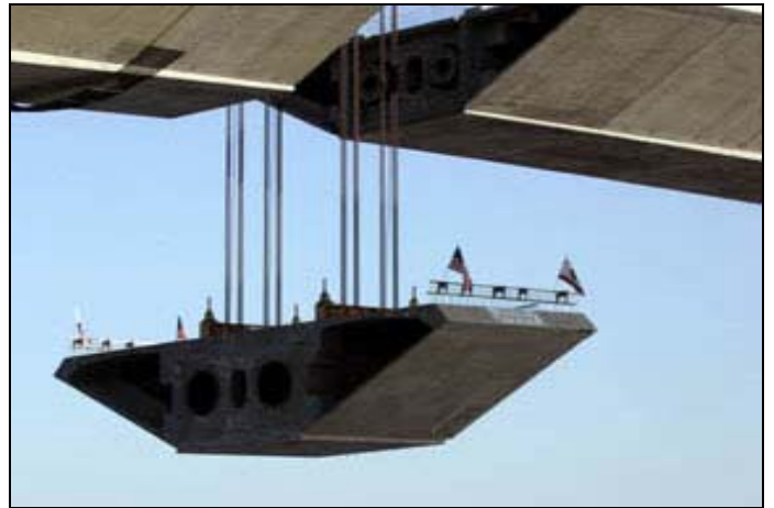
700-ton segment slowly travels up to the deck
