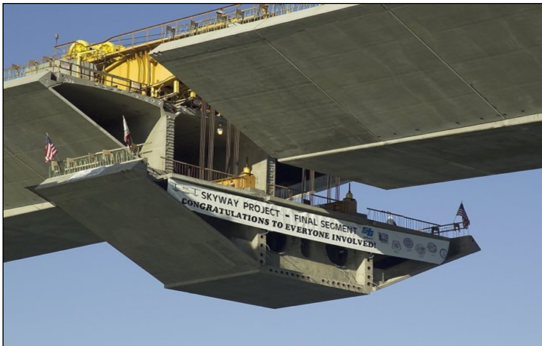
Lifting of the Last Skyway Segment
