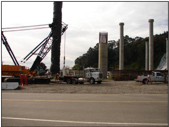
Demobilization of the SSD construction equipment (two)
