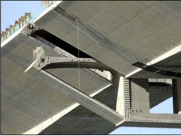
700-ton segments is almost in place
