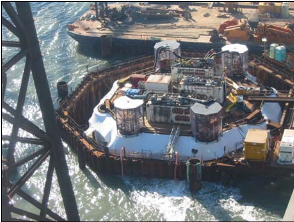
E2 Prepared and Sheltered for pile head connection
