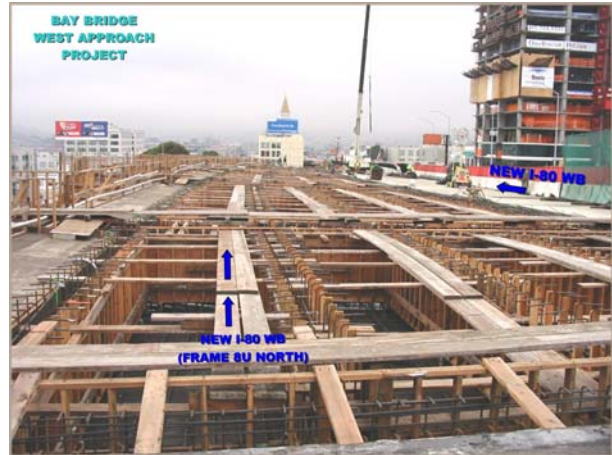
West Approach Progress Photo (two)
