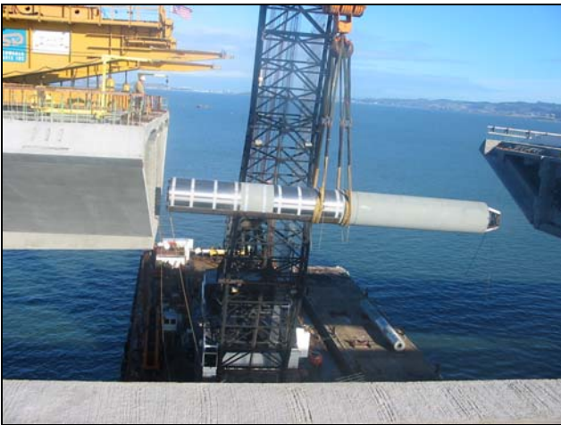
Inserting HPB BW into the Bridge
