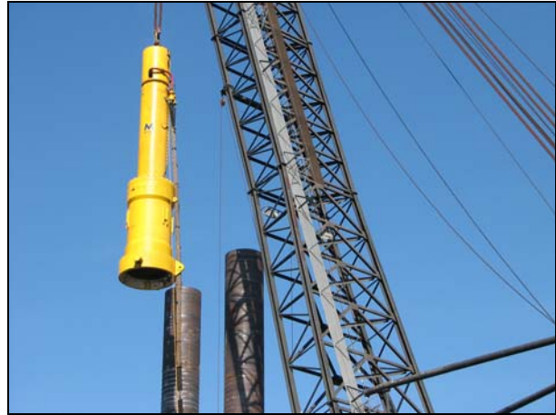
Pile Driving at SAS East Pier
