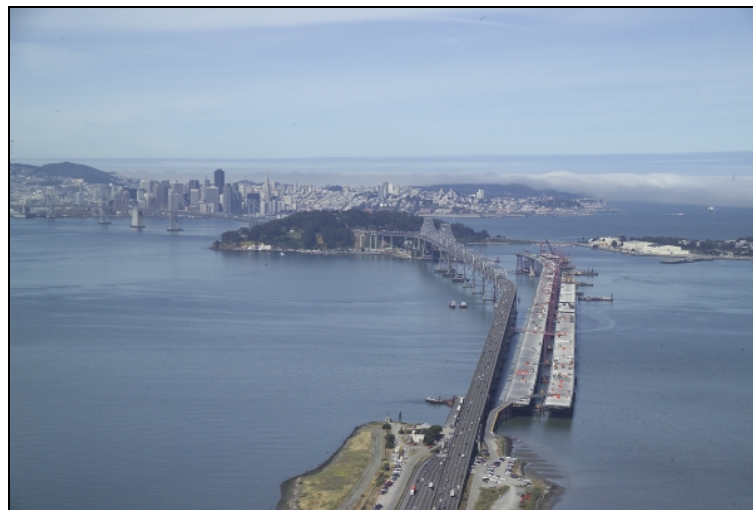
Aerial view of Bay Bridge East Span and new Skyway
