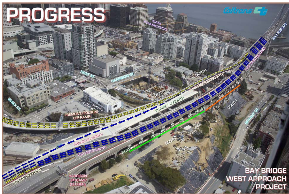
West Approach Project (two)
