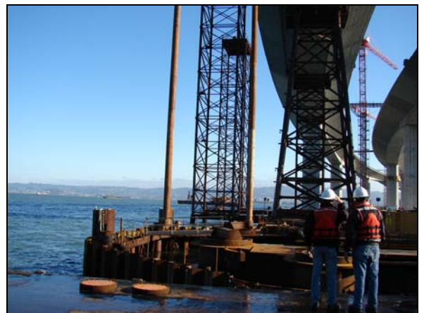
Spud Piles for Cofferdam Access Platforms at E2
