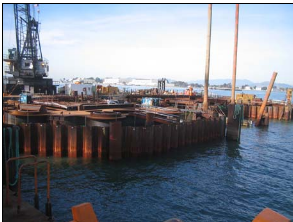
Sheet piling Cofferdam at E2
