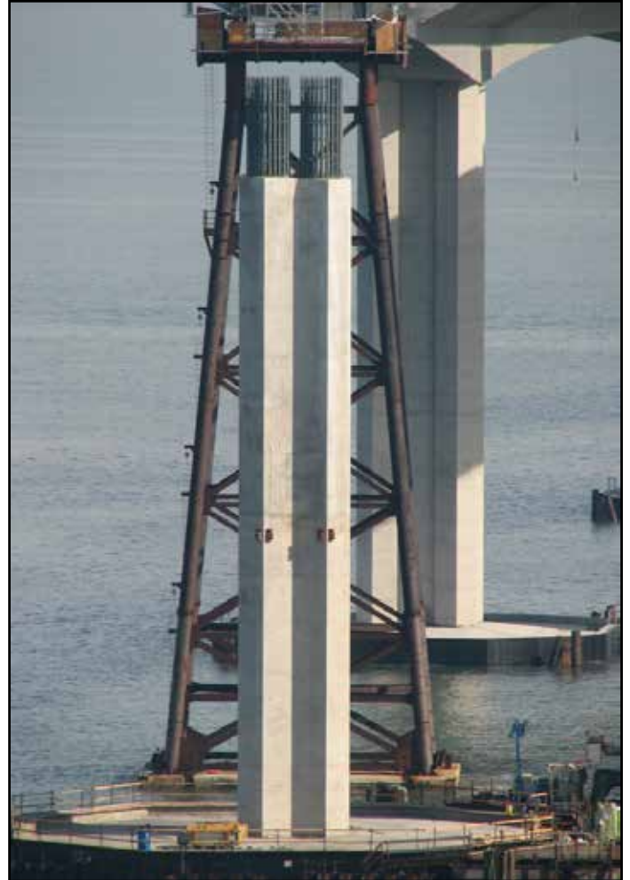
SAS Marine Foundation - E2 Foundation with Completed Westbound Column
