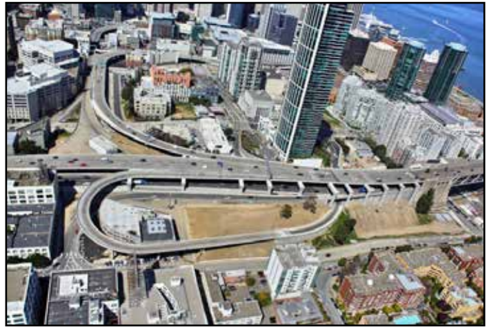
West Approach Overview
