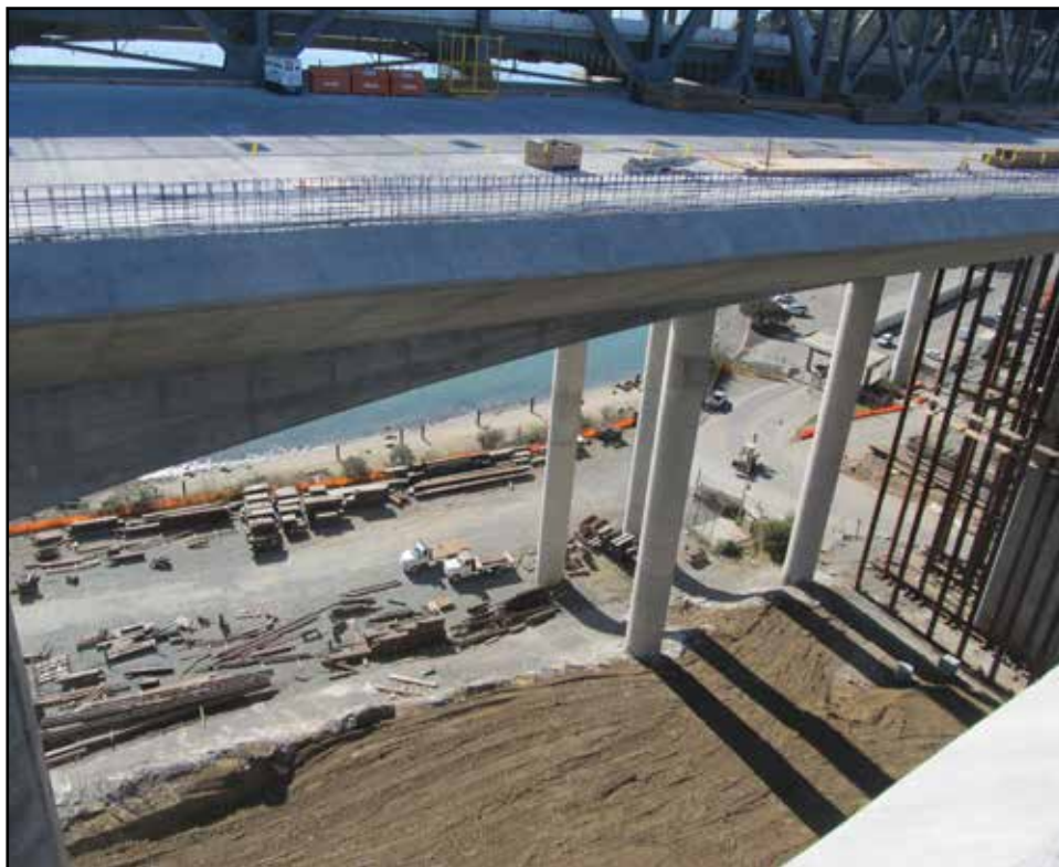
YBITS #1 Eastbound Falsework Removed to Column 4
