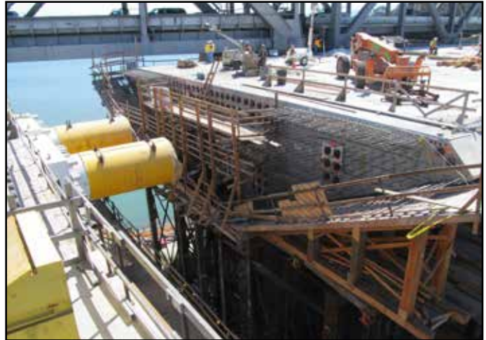
YBITS #1 Eastbound Concrete Deck Post Tensioning Complete
