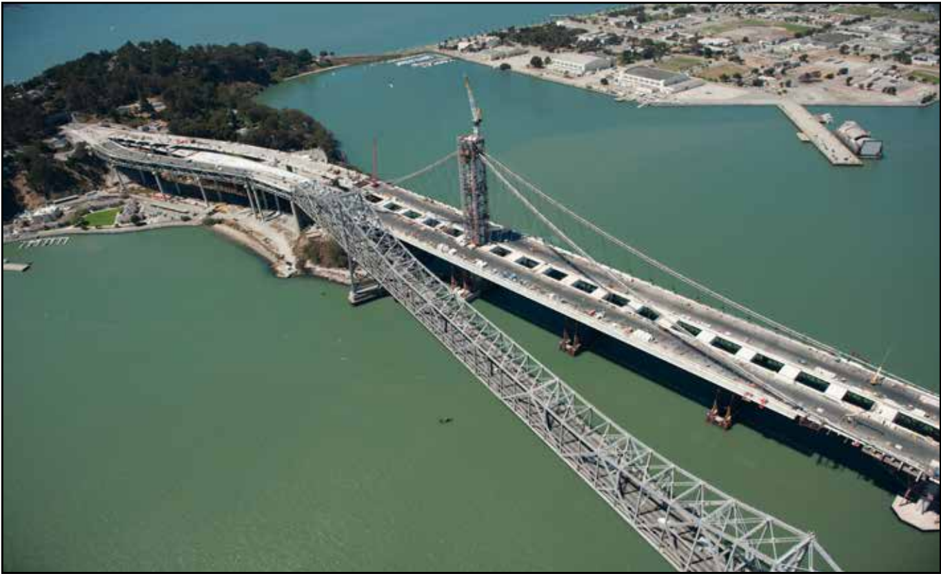
YBITS #1 Roadway Deck and SAS Construction in Progress next to Existing Cantilever Bridge
