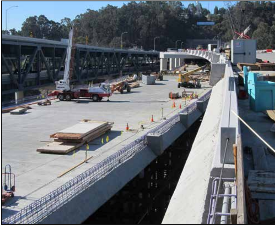
YBITS #1 Eastbound Deck Concrete Placement Completed
