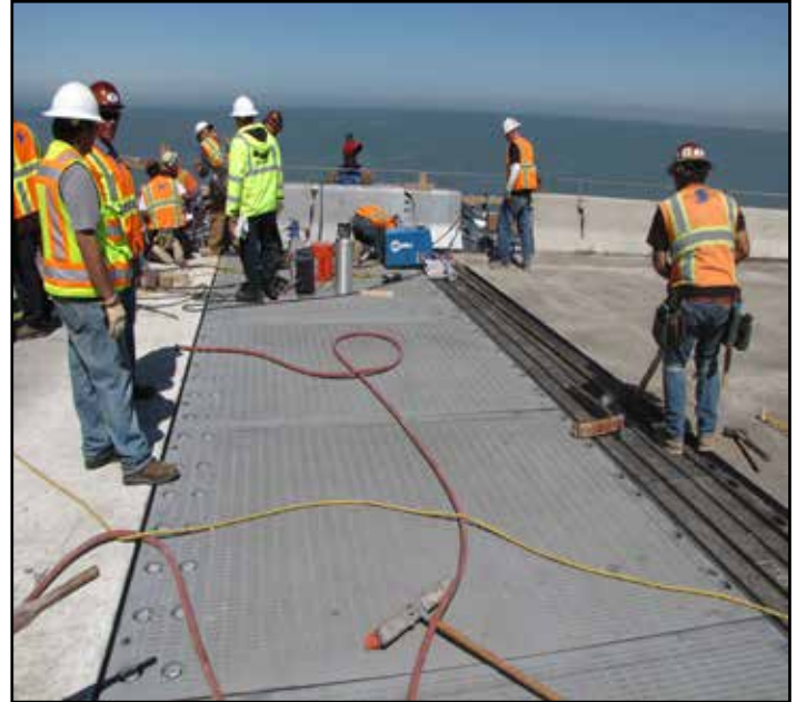
Dumbarton Bridge Seismic Joint at Pier 31
