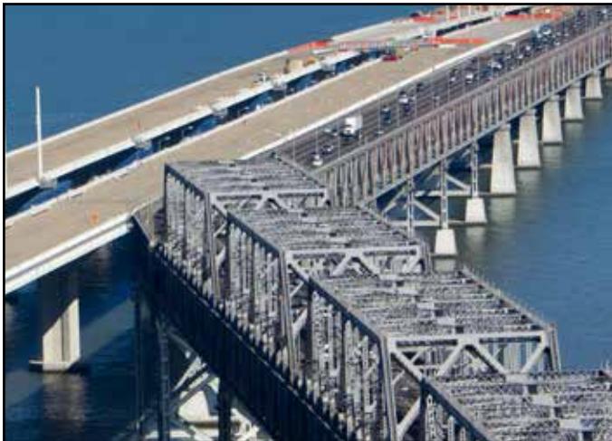
Existing San Francisco-Oakland Bay Bridge on right and new Skyway on left
