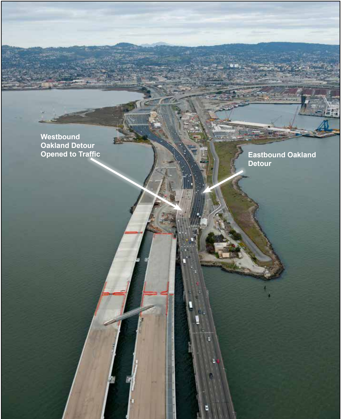
Westbound Oakland Detour Construction Progress
