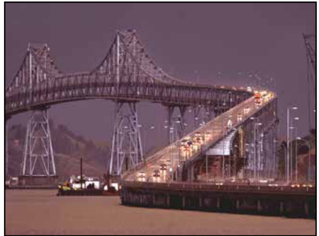
Richmond-San Rafael Bridge
