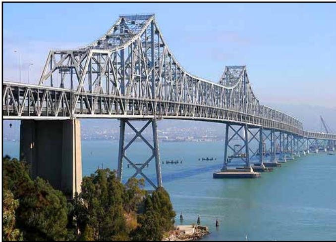
Existing San Francisco-Oakland Bay Bridge Cantilever Section to be Dismantled as Part of the YBITS #2 Contract
