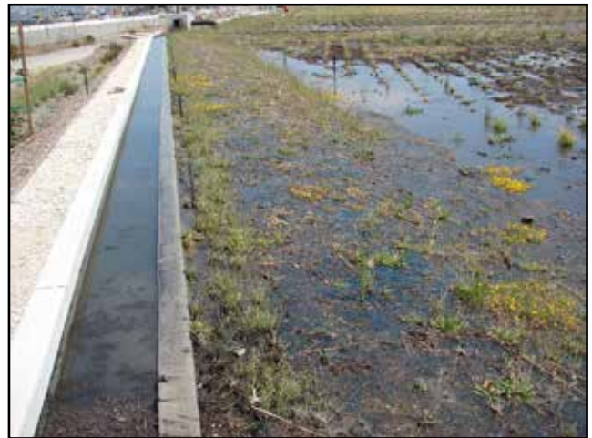
Stormwater Retention Basin
