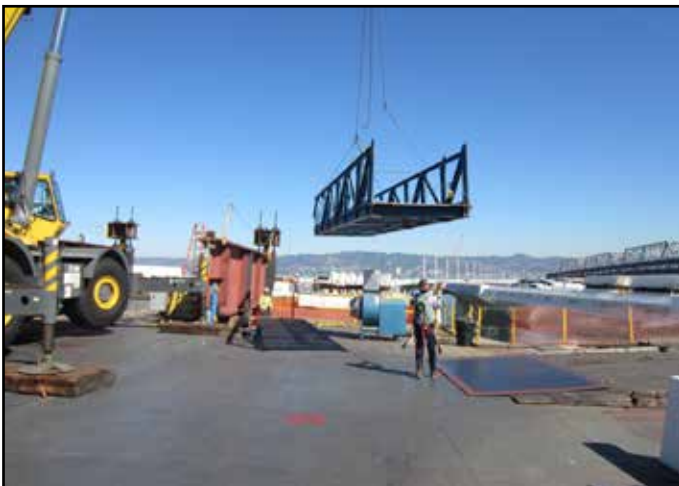
Self-Anchored Suspension Bridge Removing Eastbound Bailey Bridge
