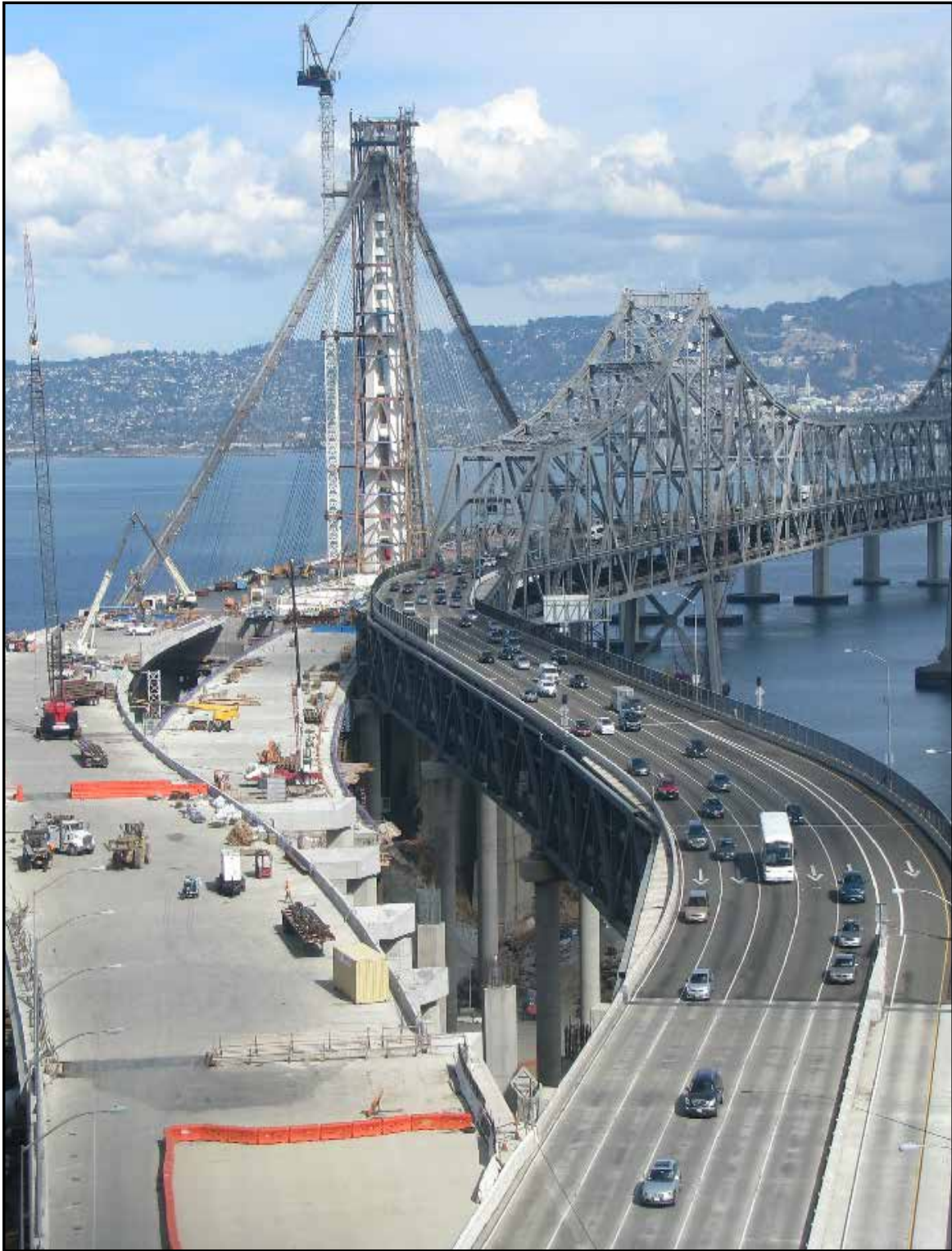
YBITS #1 Eastbound and Completed Westbound Roadway Deck Concrete Placement
