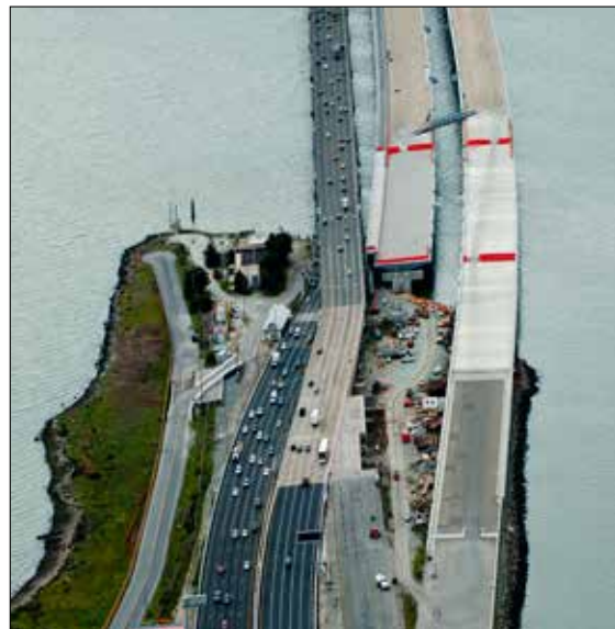
Aerial View of the Eastbound Oakland Touchdown #2 Construction Progress
