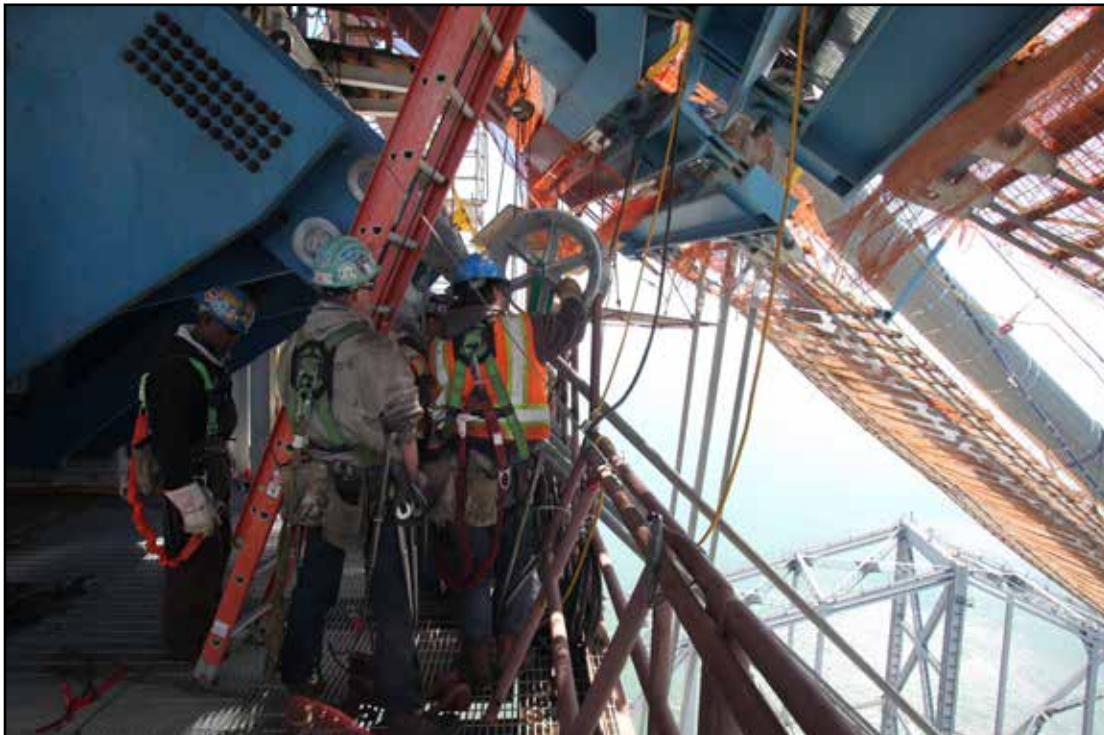
Self-Anchored Suspension Bridge Iron Workers Removing the Tie-Back Cables
