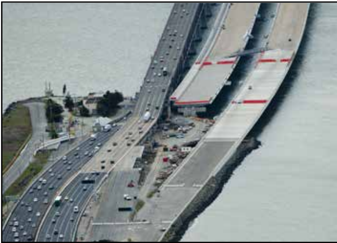
Oakland Detour - Westbound Opened to Traffic
