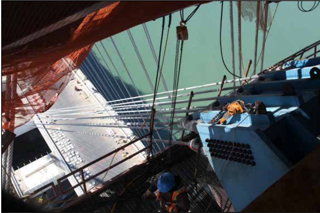
Self-Anchored Suspension Bridge Tower Tie-Back Cables
