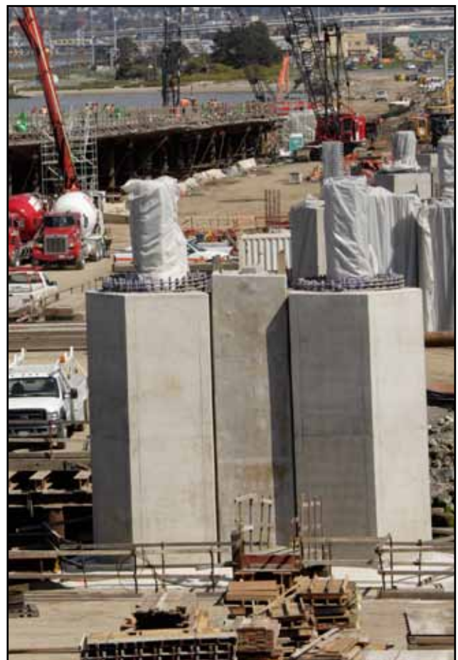
Oakland Touchdown #1 Eastbound Piers with Westbound in Background
