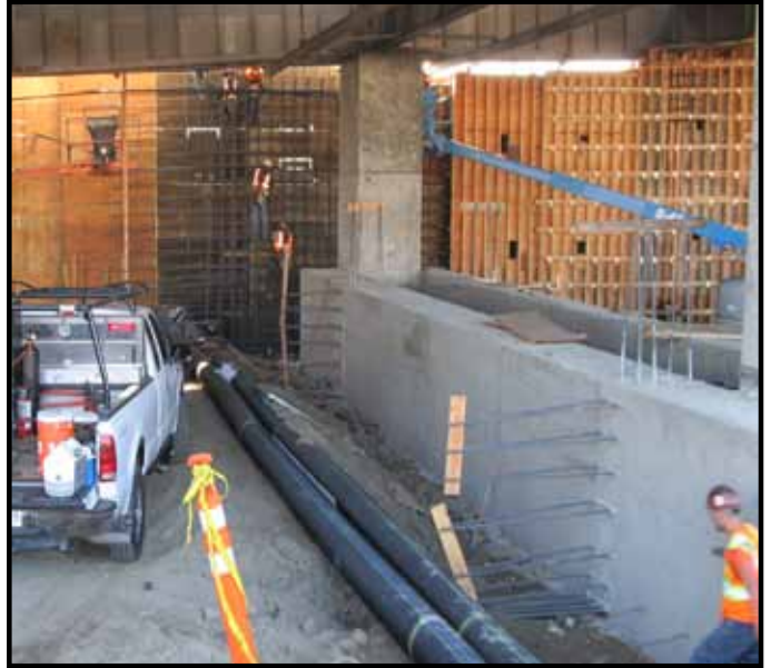
Straddle Wall Drainage
