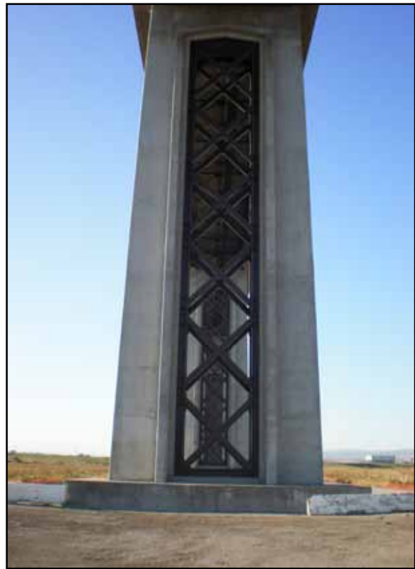
Completed Cross Frames on Sherman Island
