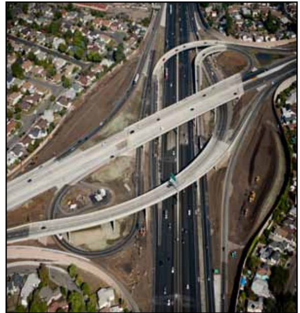
Aerial View of Construction Progress
