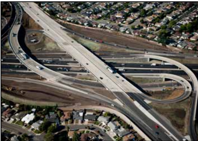
Aerial View of the Recently Completed 92/880 Interchange Looking East
