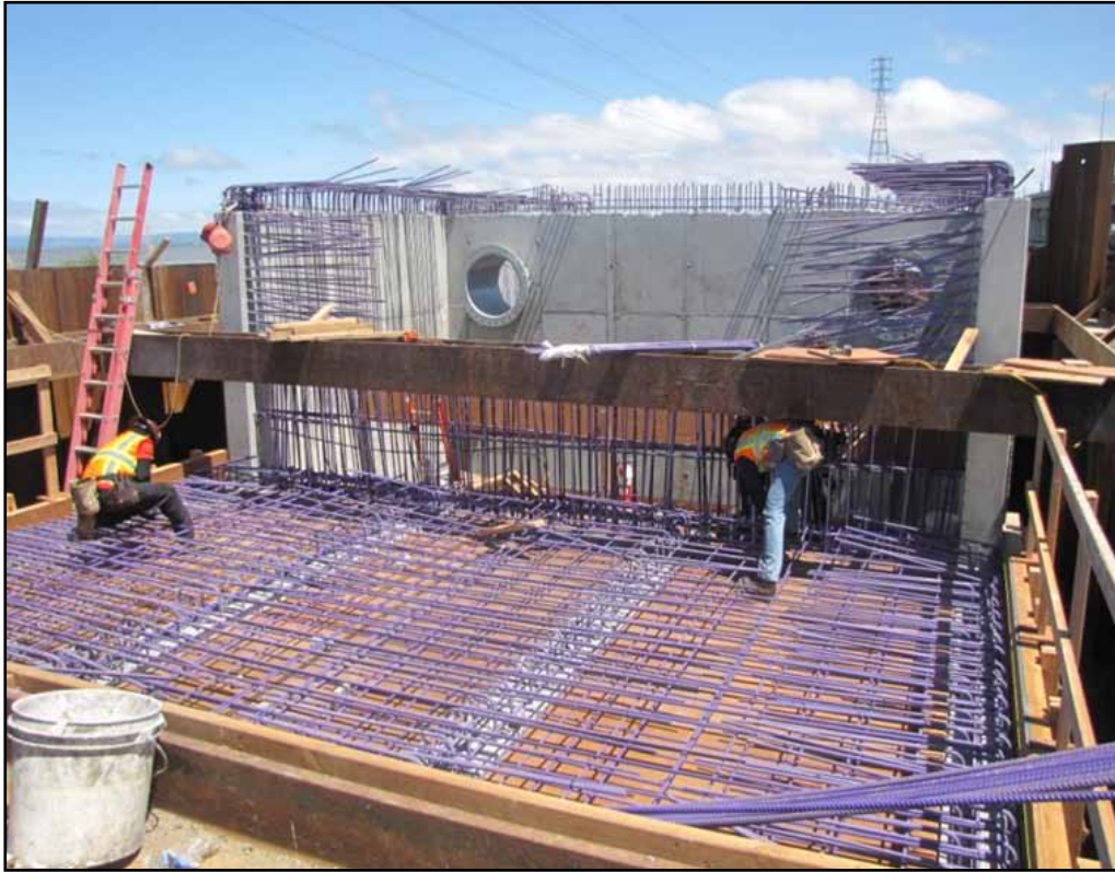
Pump Station Deck Rebar Being Placed
