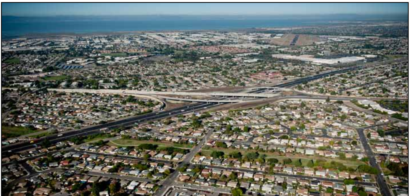
Aerial View of Construction Progress
