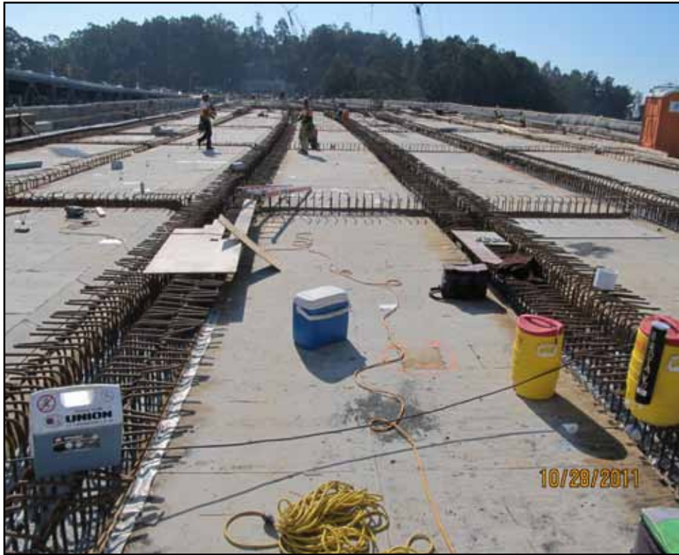
First Westbound Roadway Deck Formwork Installed between Bent 4 and Pier Cap 7
