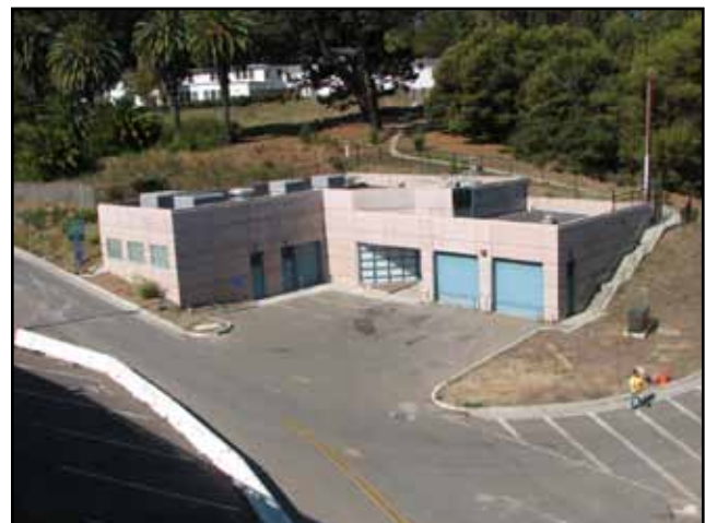
New YBI Electrical Substation
