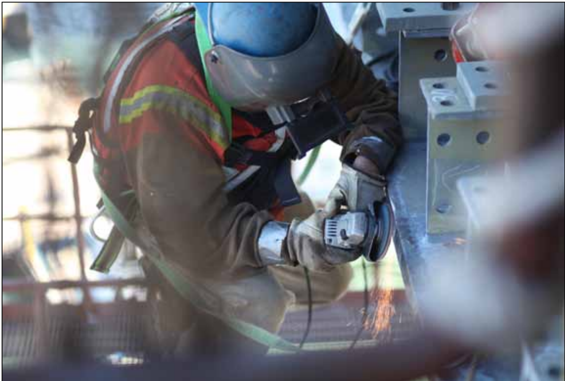
Grinding the Edge of Floorbeam Plate
