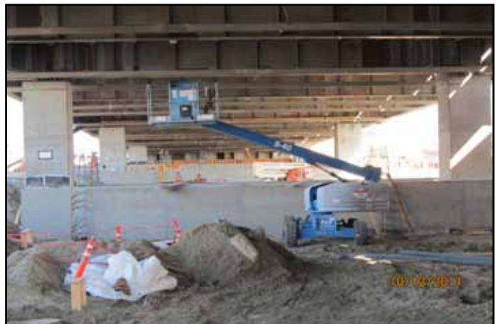
Straddle Foundations Poured and Formwork Stripped
