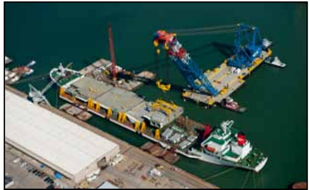
Off Loading the Final Four Roadway Boxes at Pier 7 in Oakland
