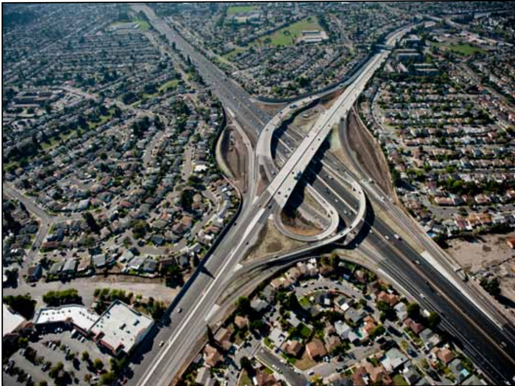
Aerial of Recently Completed SR 92/880 Interchange Looking West
