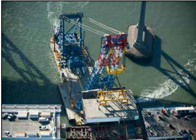
Shear-Leg Barge Crane Hoisting Roadway Box 13 Eastbound for Installation
