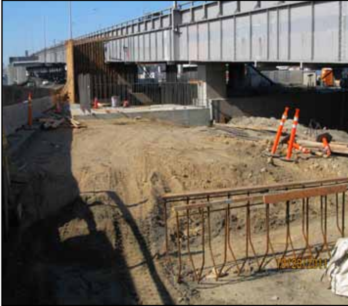
Foundation Footings for Pier Wall
