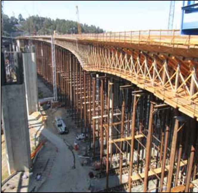
YBITS #1 Westbound Falsework Looking West
