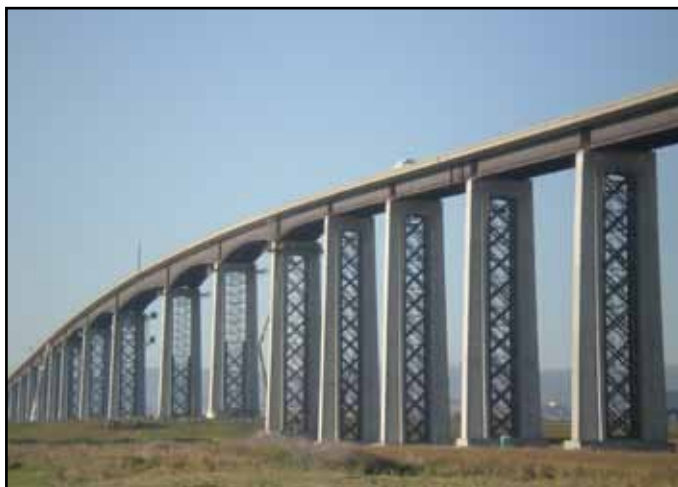
Antioch Bridge - Last Cross Frames Being Installed at Piers 20 and 21
