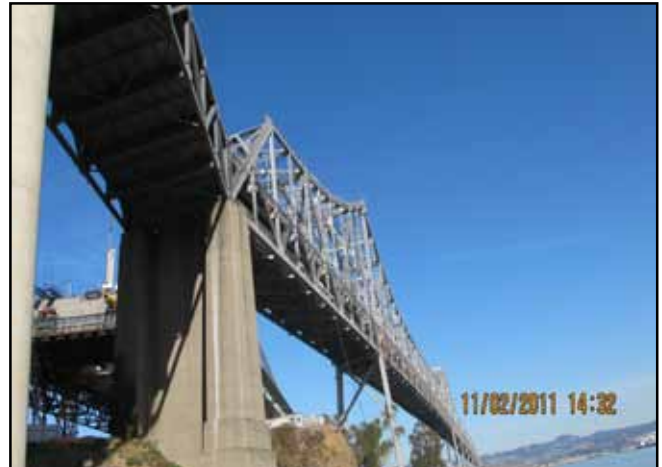
Dismantling Scope Included in the Future YBITS#2 Contract - YBI Detour at left, E-1 Center, Cantilever at right
