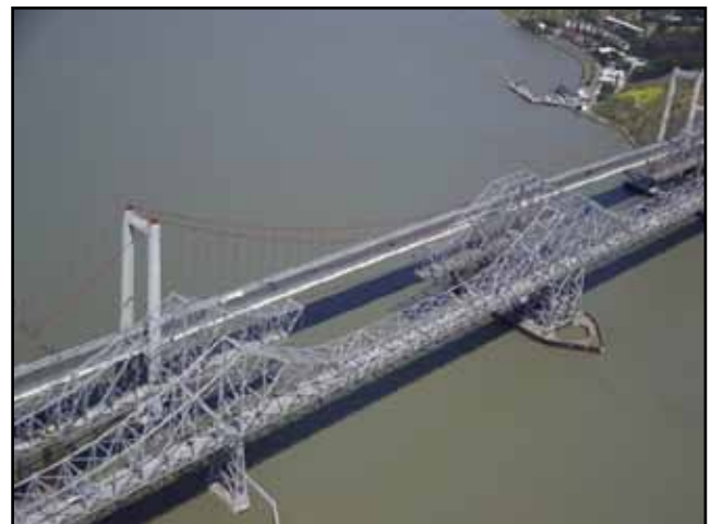
1958 Carquinez Bridge (foreground) with the 1927 Span (middle) under Demolition and the New Alfred Zampa Memorial Bridge (background)
