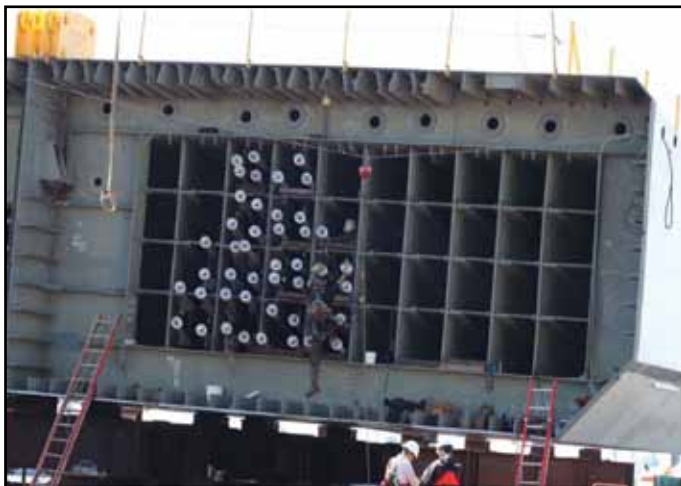
Parallel Wire Strand Cable Anchorage Rods Installation in Roadway Box 14 Eastbound
