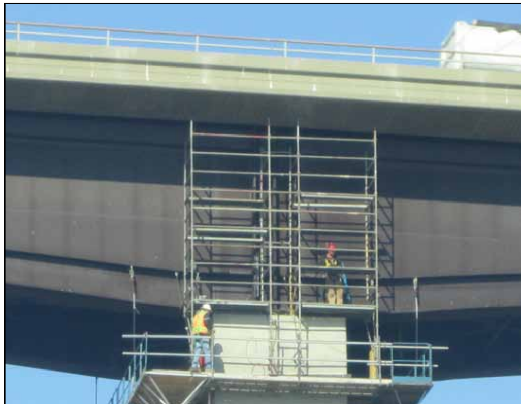
Installation of Web Stiffeners at Jacking Point, Pier 22
