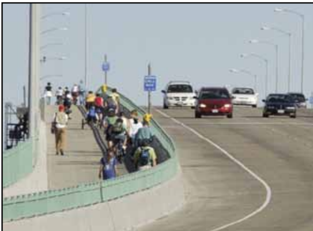
Benicia-Martinez Bridge Bicycle/Pedestrian Pathway Opened to the Public in August 2009
