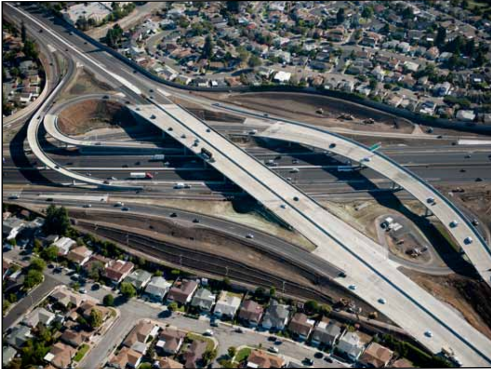
Aerial of Recently Completed 92/880 Interchange Looking East
