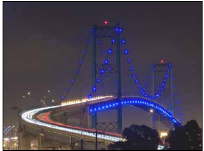
Los Angeles-Vincent Thomas Bridge
