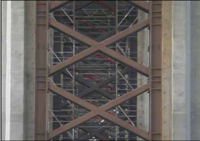
Antioch Bridge - Cross Frames Installed between Bent Columns
