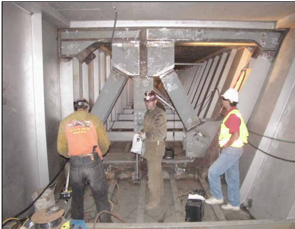
Welding Jacking Frame at Pier 18 Exterior Cell Eastbound Structure
