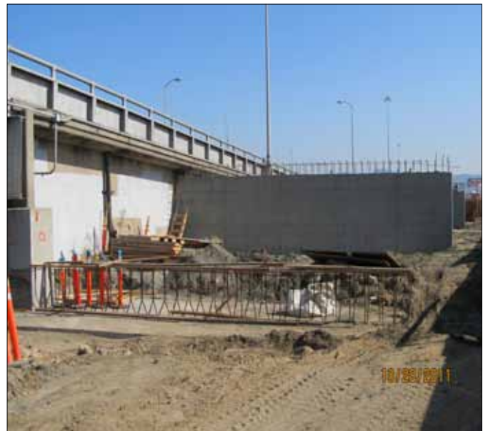
Foundation Pier Wall
