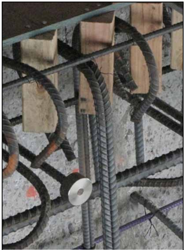
Pier Cap Drill and bond Dowels at Pier 18
