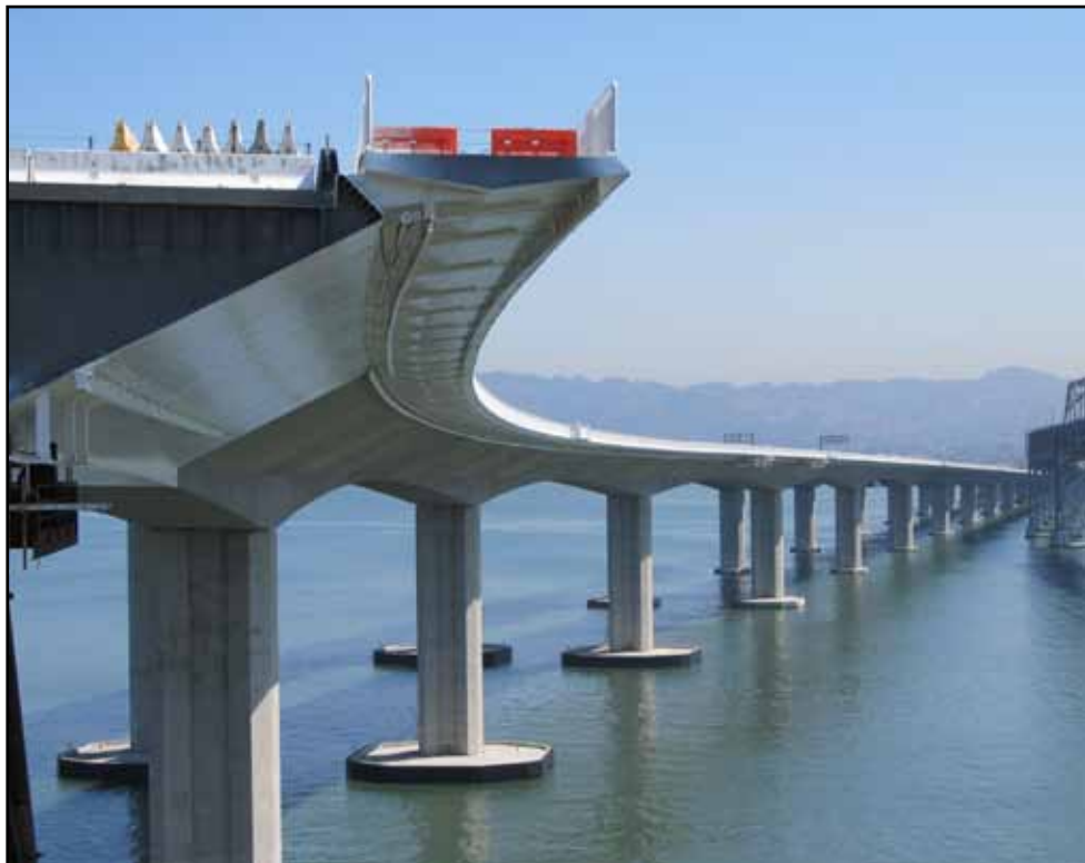
Skyway on the left and Existing Bridge on the Right Looking East toward Oakland
