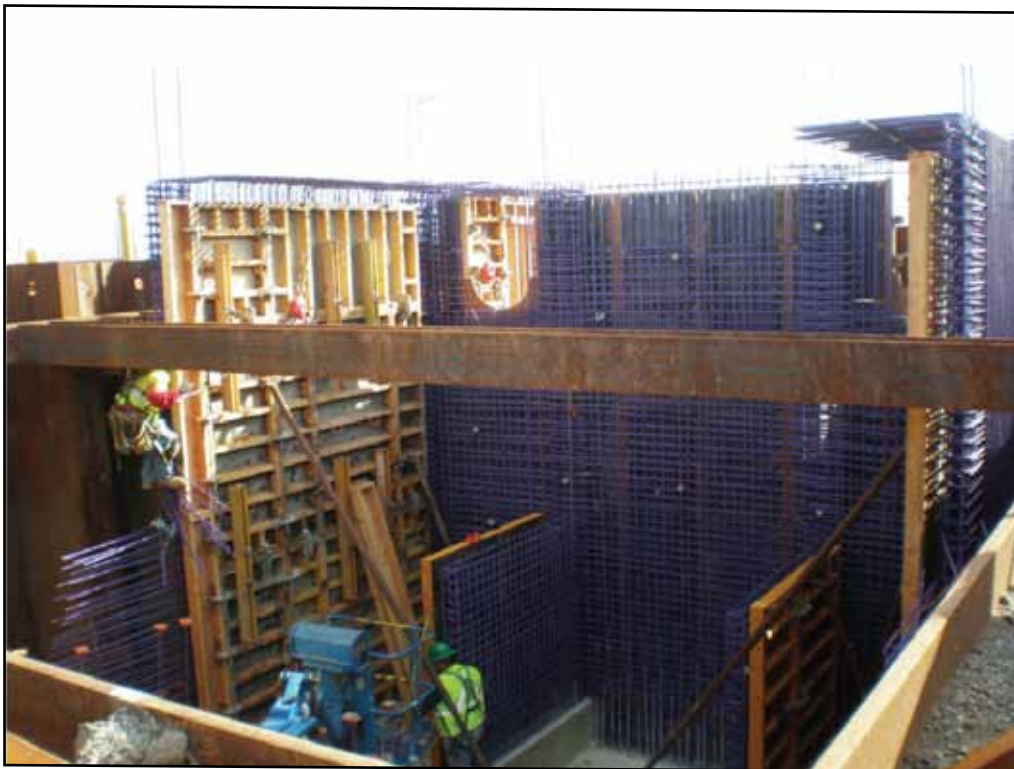
Dumbarton Bridge - Wall Being Cast for Pump Station
