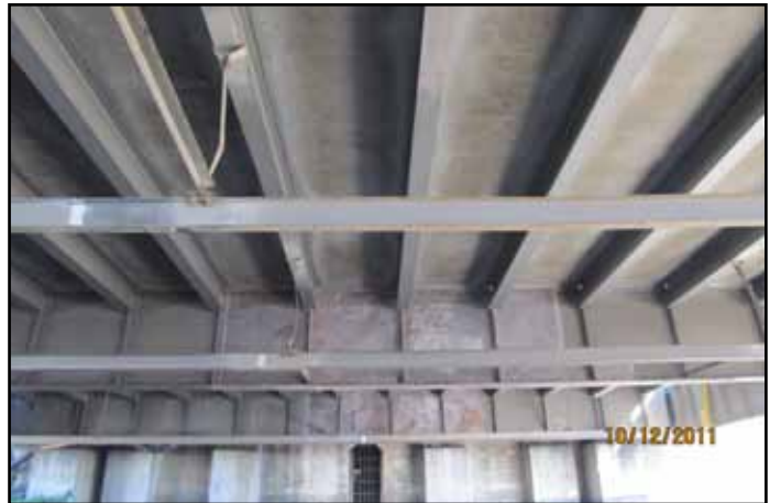
Oakland Detour Lead Abatement Completed
