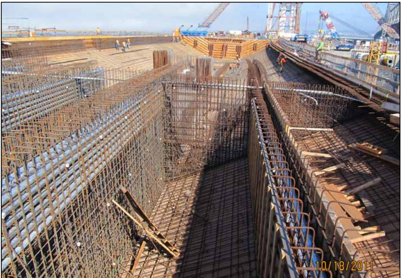
YBITS #1 Westbound Span 3 Rebar Installation for Soffit and Stem Walls
