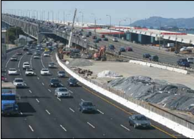
Oakland Detour - Westbound Work in Progress
