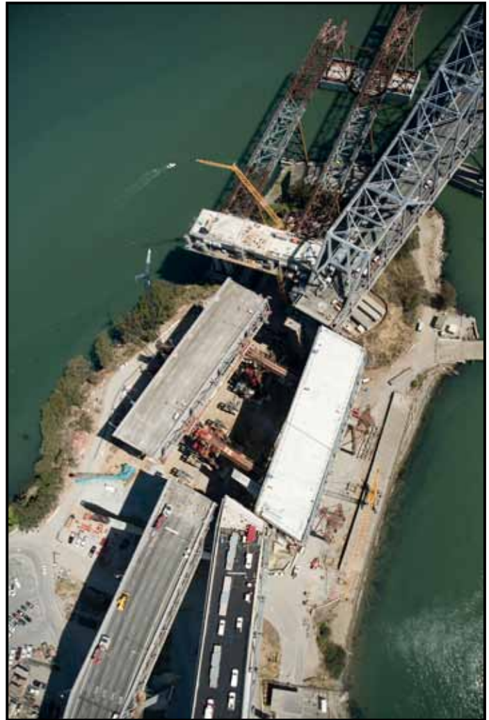
YBID East Tie-In Rolled in on Labor Day 2009 Weekend
