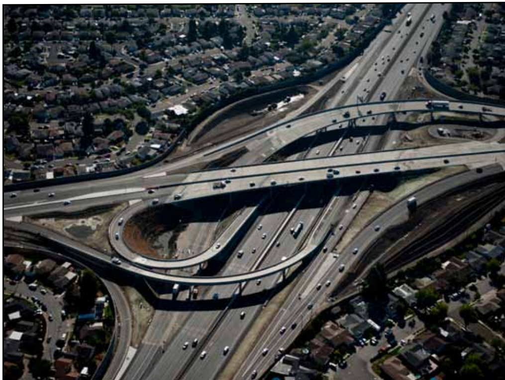
Aerial of Recently Completed SR 92/880 Interchange Looking South
