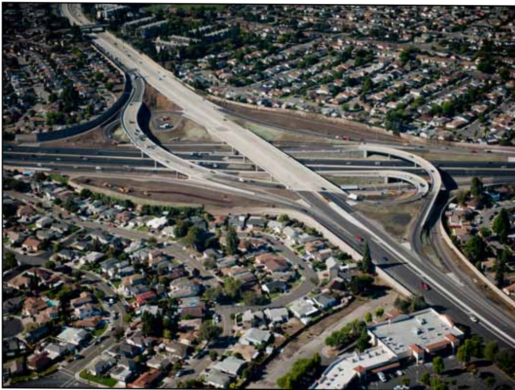
Aerial of Recently Completed 92/880 Interchange Nearing Completion Looking West
