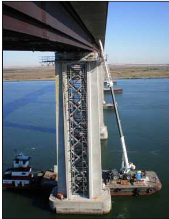
Superstructure Lowered onto New Isolation Bearing at Pier 15
