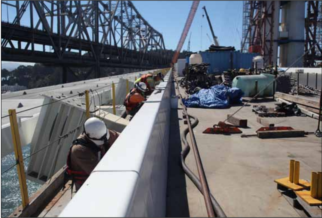
Conduits Installation on Eastbound Roadway Barrier
