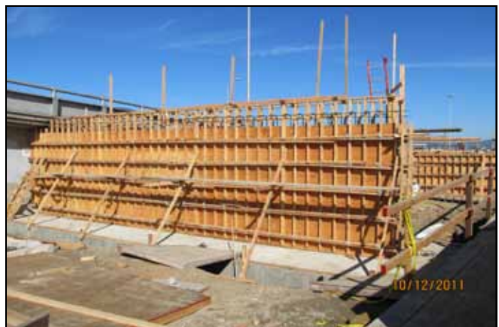
Westbound Foundation Wall Formwork
