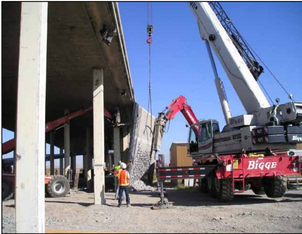
Removal of Curtain Wall
