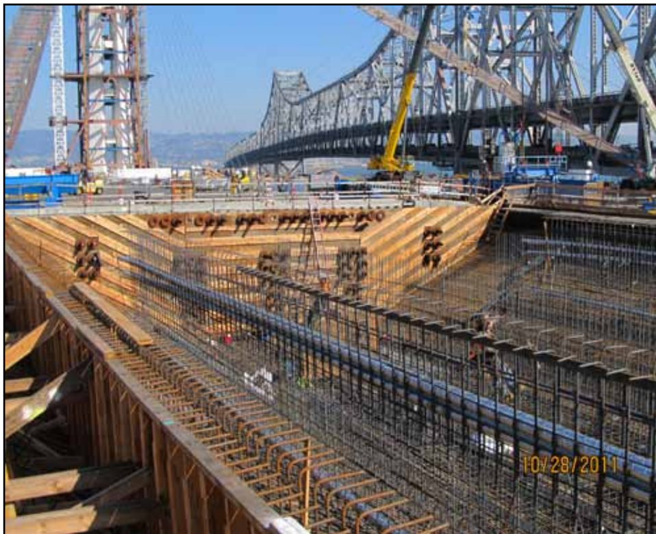
YBITS #1 Westbound Span Rebar Installation
