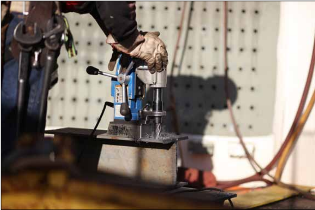
Drilling Holes at I-Beam for Support at the Tower Grillage
