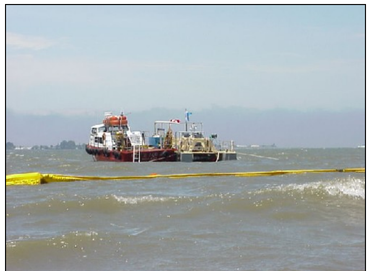
Turbidity Curtain and Water Quality Monitoring Boats
