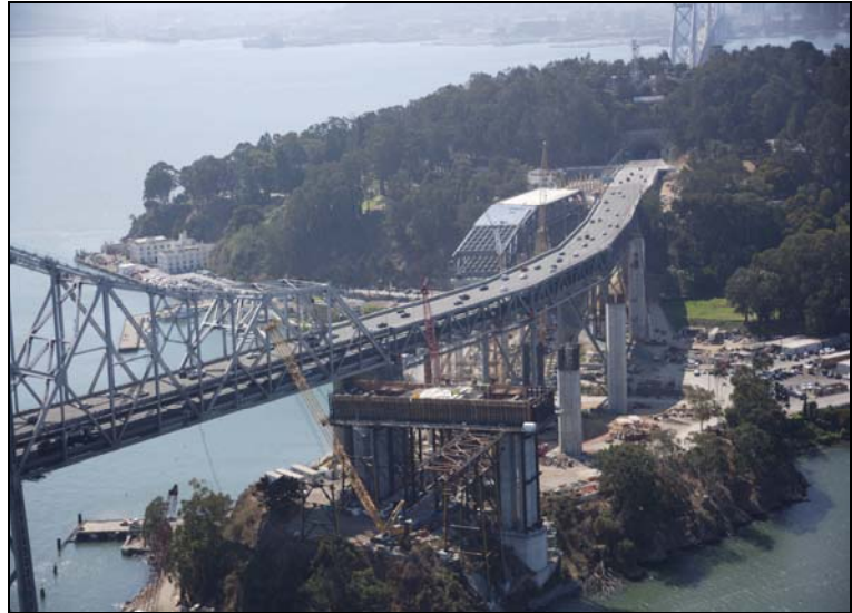
Aerial Photo of SAS W2 Cap Beam and YBID Viaduct
