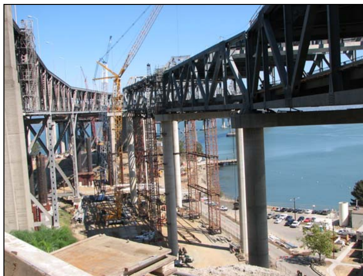
YBID – Viaduct Span 48, 49 & 50
