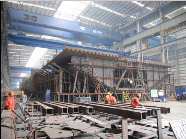
OBG (Orthotropic Box Girder) and Temporary Work
