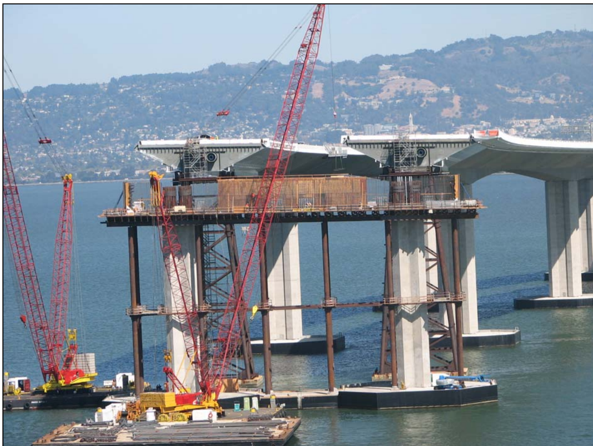
SAS – E2 Crossbeam Temporary Work
