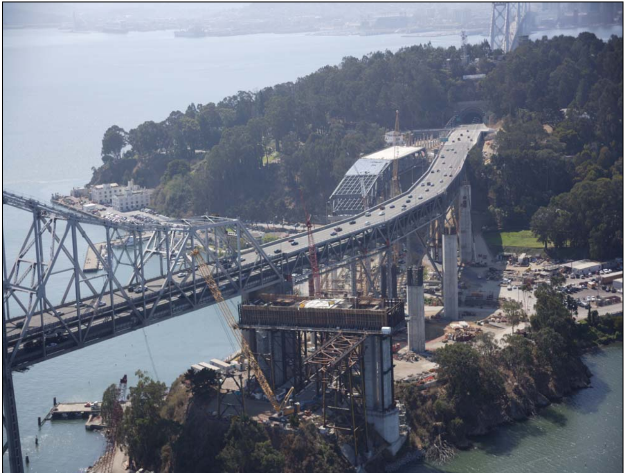
Aerial Photo of SAS W2 Cap Beam and the YBID Viaduct
