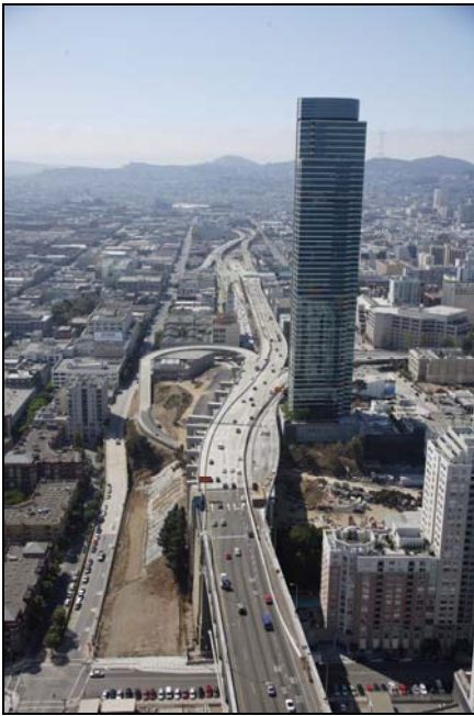
The West Approach
