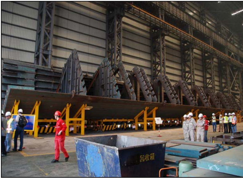
SAS – Tower Leg
