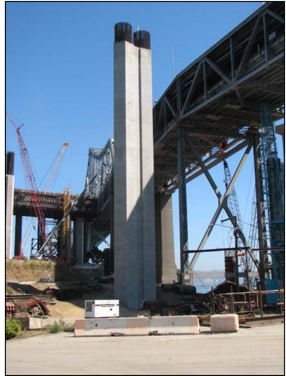
YBID Advanced Work Completed Column W4L
