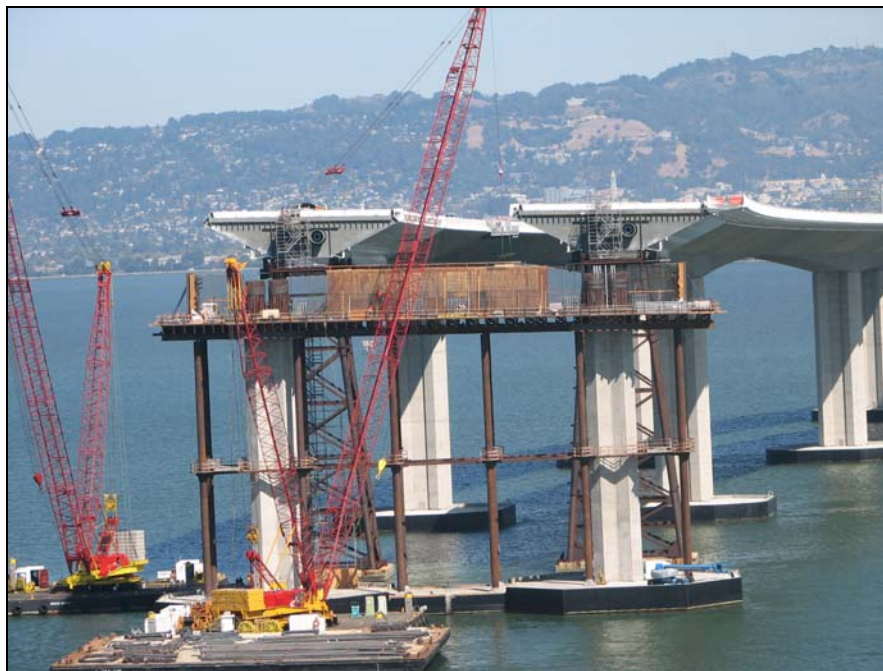
SAS – E2 Crossbeam Temporary Supports
