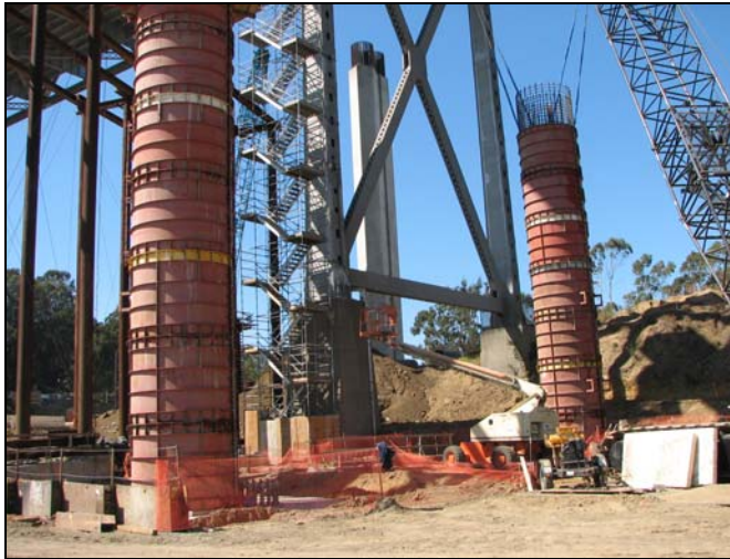
YBID - East Tie-In Skid Bents Columns 52A North and South
