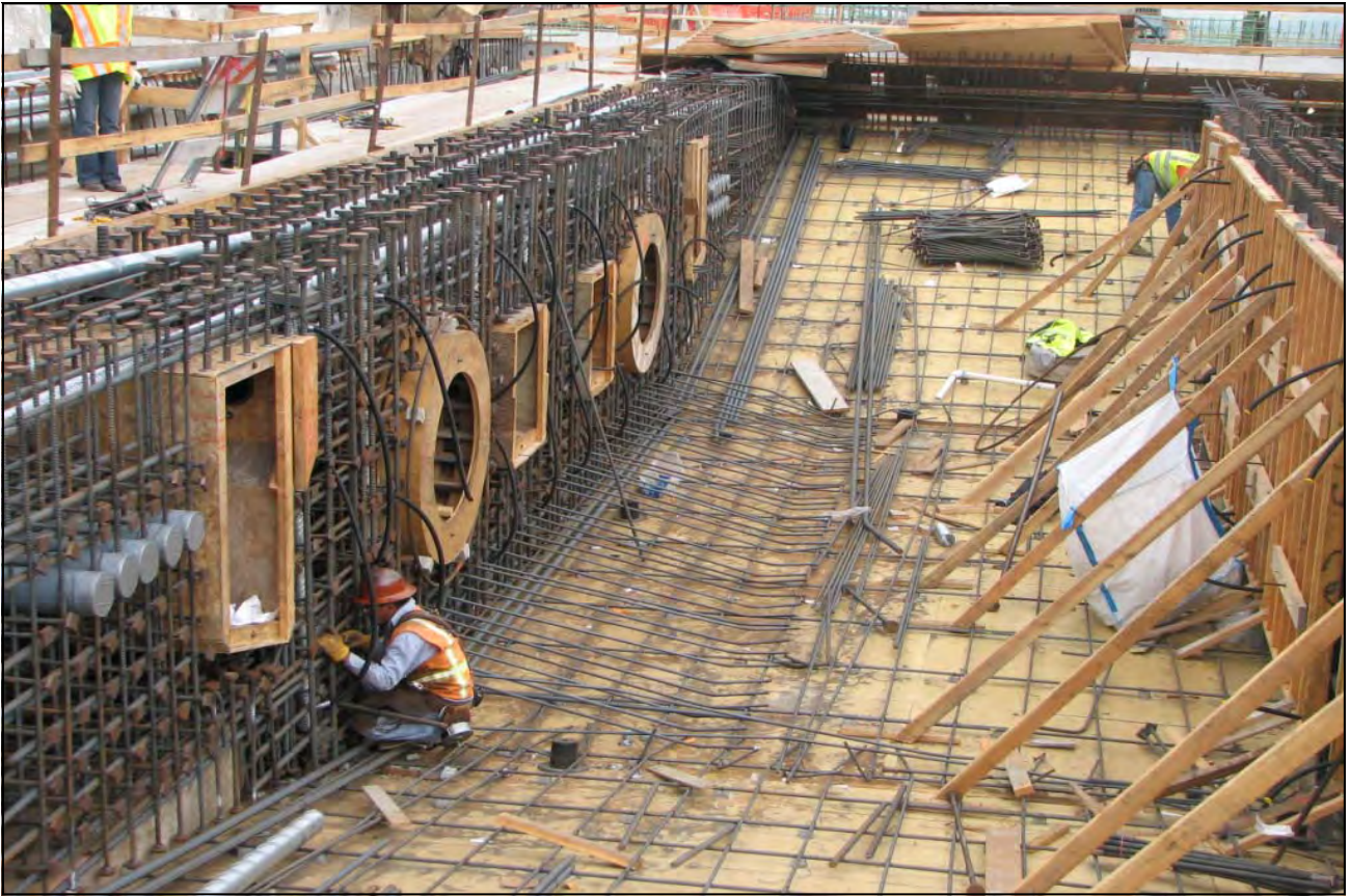
OTD1 Hinge Pipe EE Rebar and Blockout Installation
