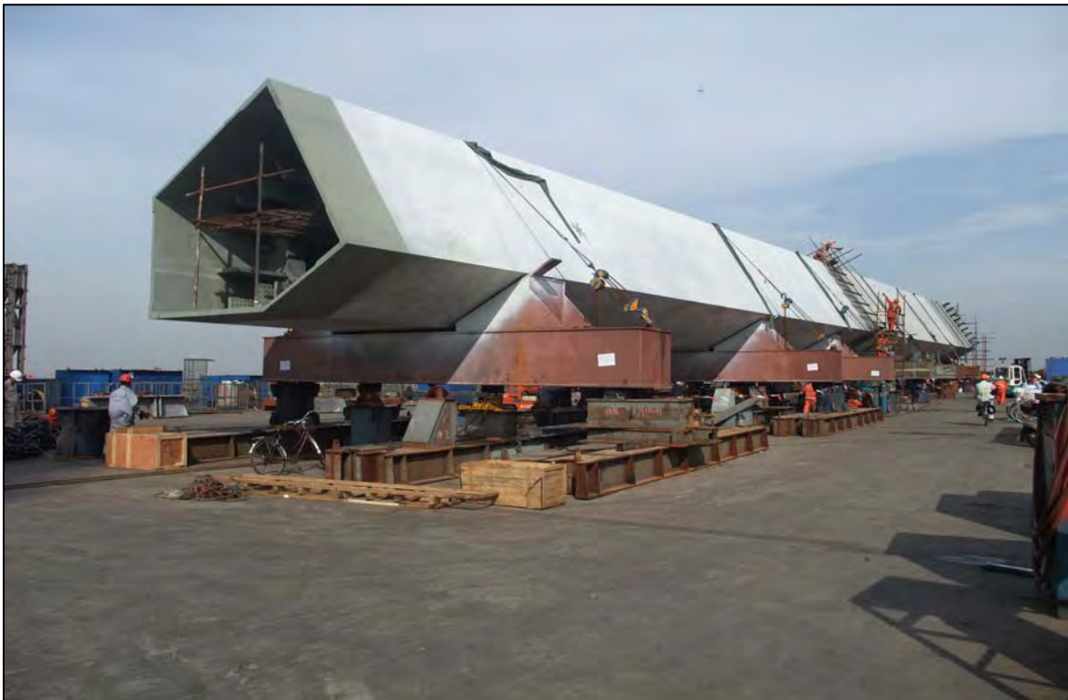
East Tower—Lifts 1 and 2 in Trial Assembly
