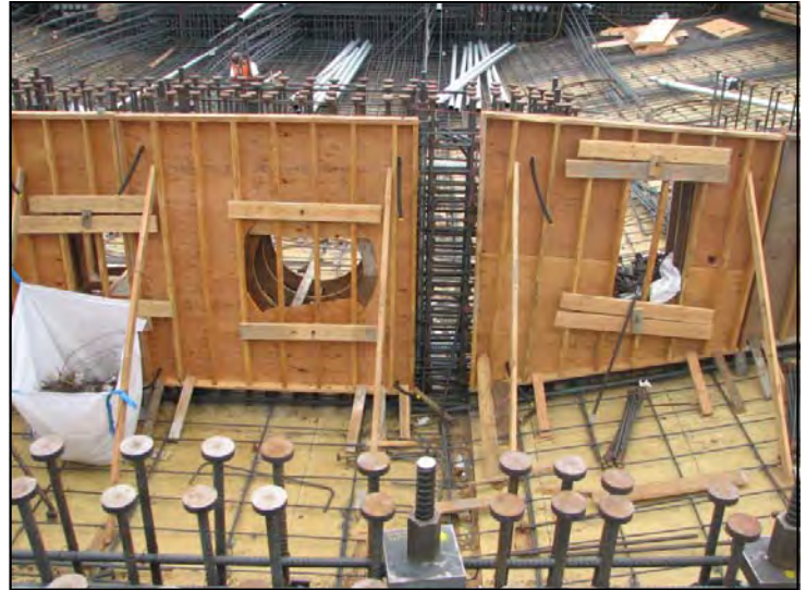
Hinge Rebar and Hinge Pipe Blockout Installation
