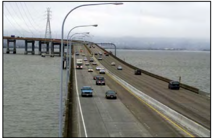
High-Rise Section of San Mateo-Hayward Bridge
