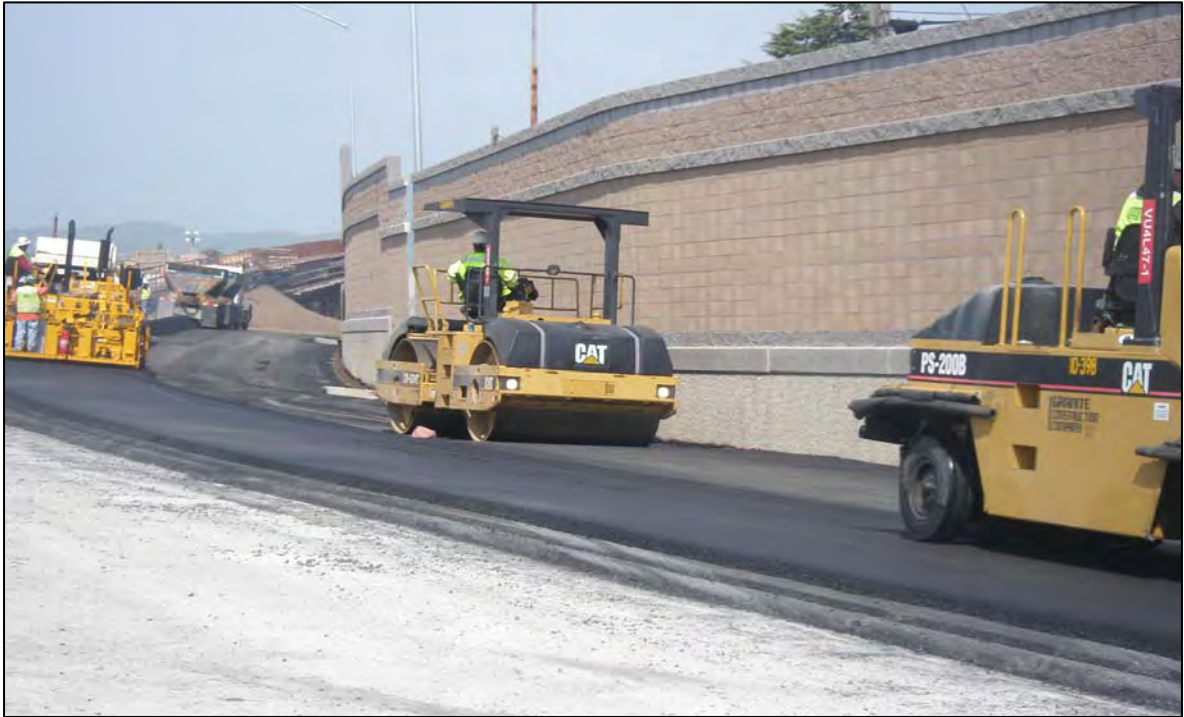
Paving Operation on Eastbound 92
