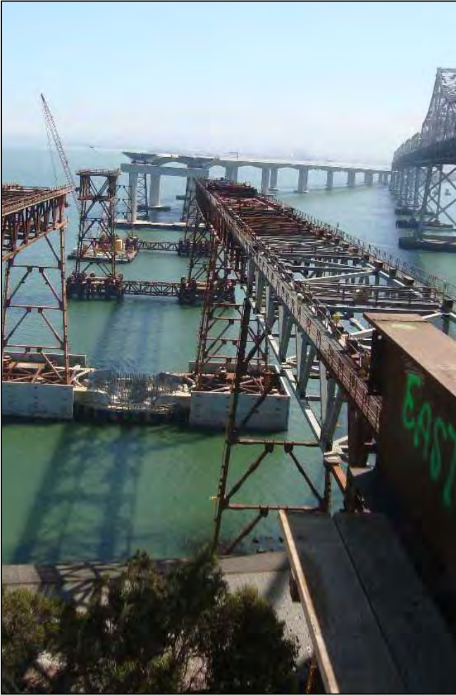
View of Temporary Truss
