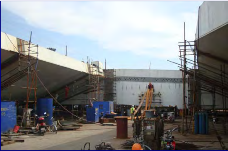
OBG Crossbeam Trial Fit Up
