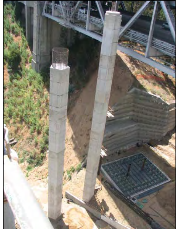
YBITS W7L-S, W7 EB Ramp Final Lift Complete
