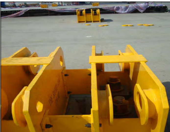
Yellow Lifting Lugs for Lifting the Roadway Decks
