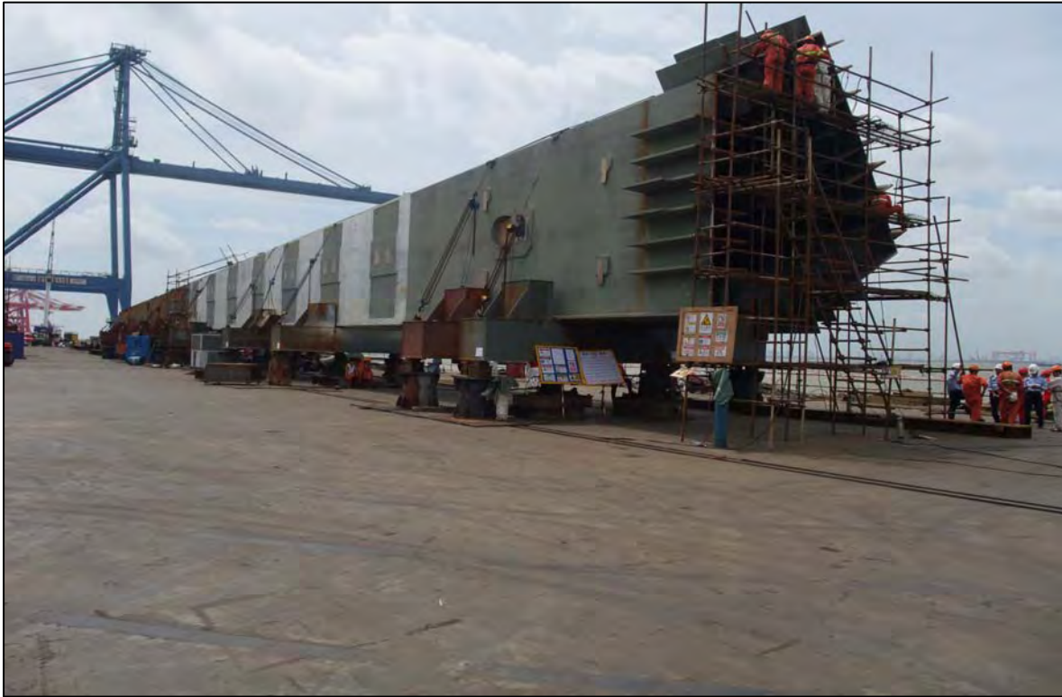
South Tower Lifts 1 and 2 in Trial Assembly
