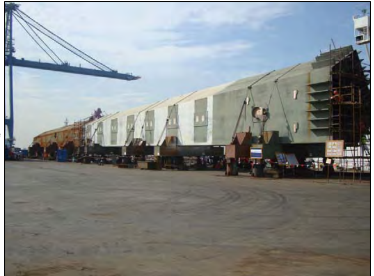
East & South Shafts, Lifts 1 & 2 at Heavy Duty Dock
