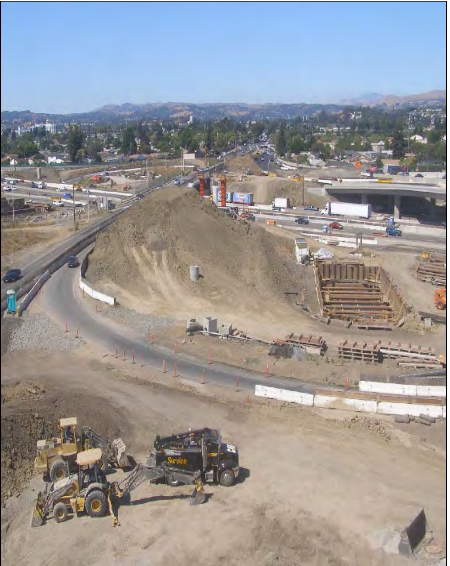
Site Preparation of New Route 92 and Interstate 880 Separator
