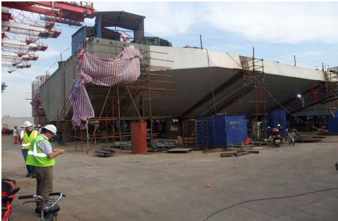
View of the West Line OBG which Contains the Abutment Transition
