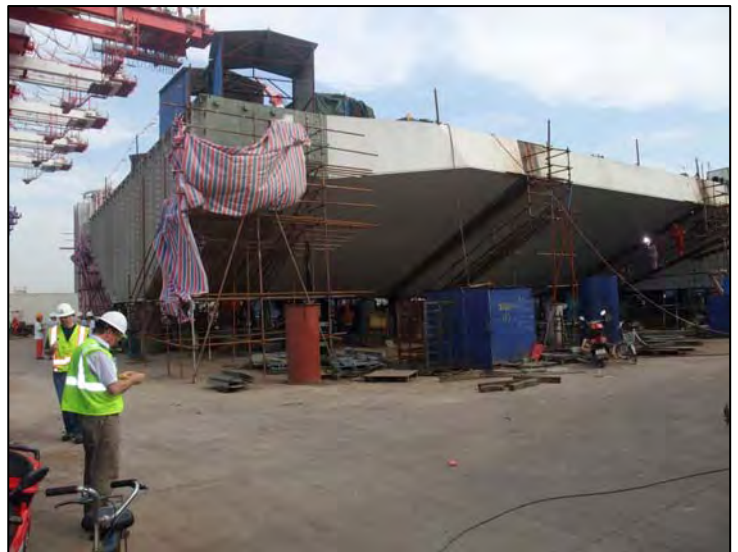
View of the West Line OBG which Contains the abutment Transition
