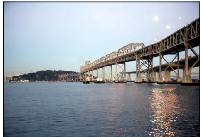
Existing East Span of Bay Bridge
