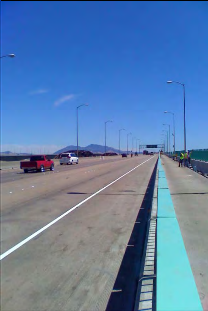
New Pedestrian Bicycle Path on Benicia-Martinez Bridge Under Construction
