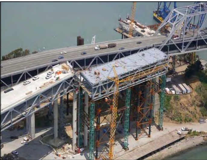
East Tie-in Truss Structure Being Erected on Yerba Buena Island
