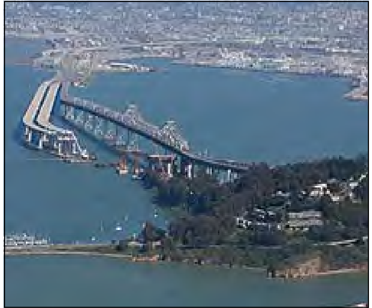
Completed Skyway Left of Existing East Span
