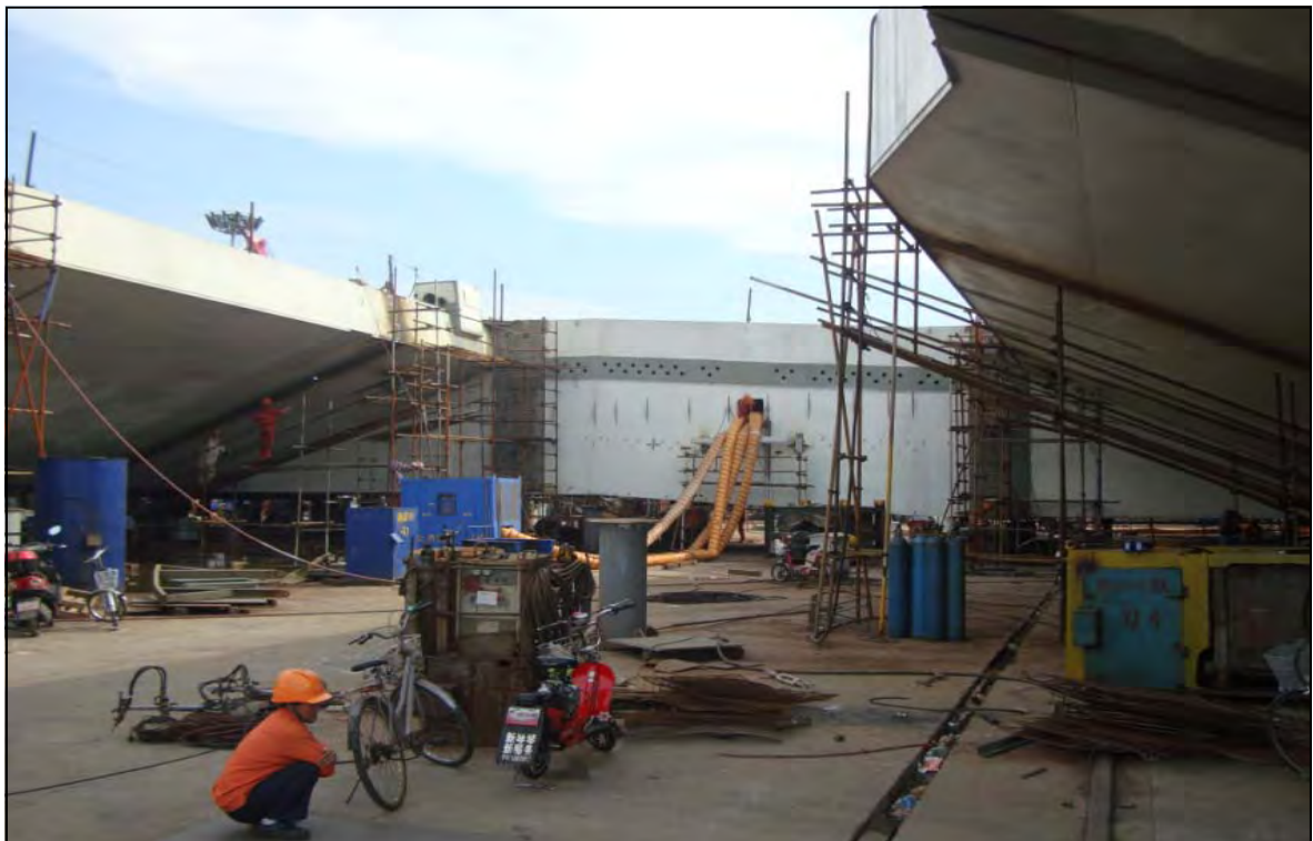
Cross Beam #1 Undergoing Fit Up between WB and EB Lift 1
