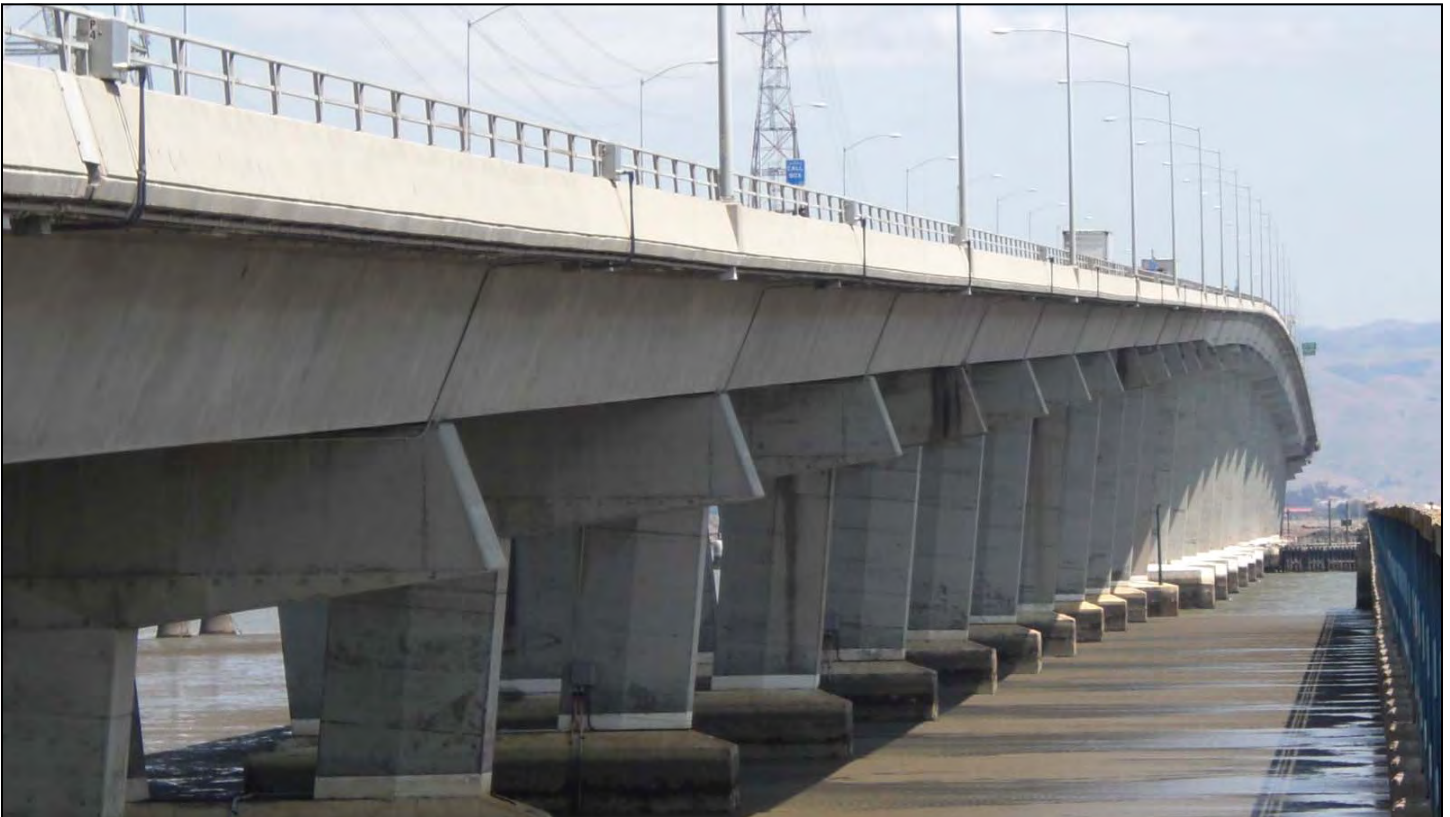
Existing Dumbarton Bridge Looking East towards the Alameda County Foothills
