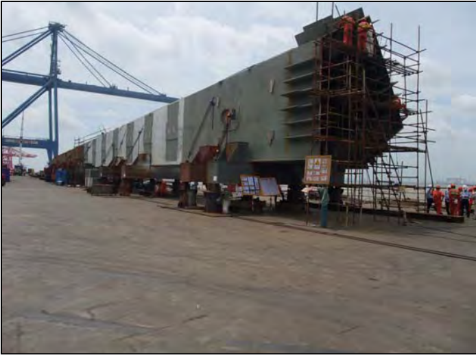
South Tower Lifts 1 and 2 Being Trial Assembled
