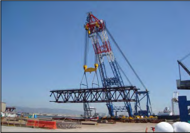
Shear-Leg Barge Crane Lifting Truss
