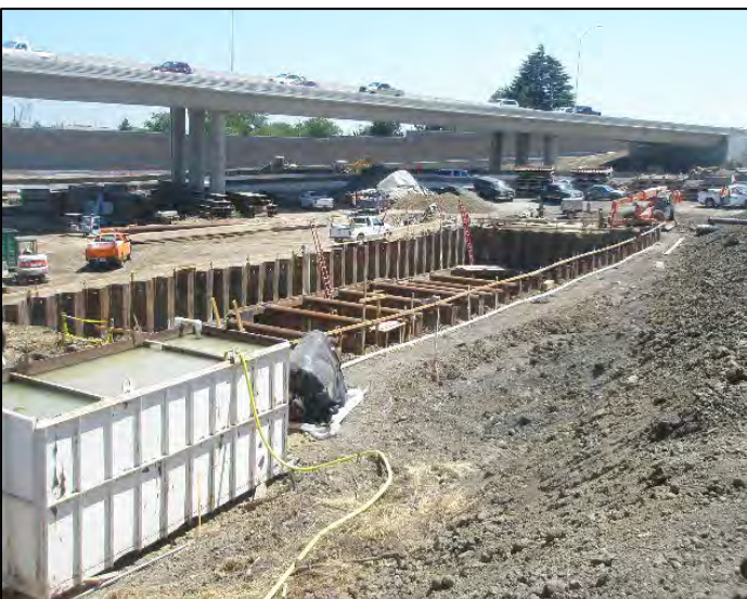
Embankment Construction for 92/880 Separator Bridge
