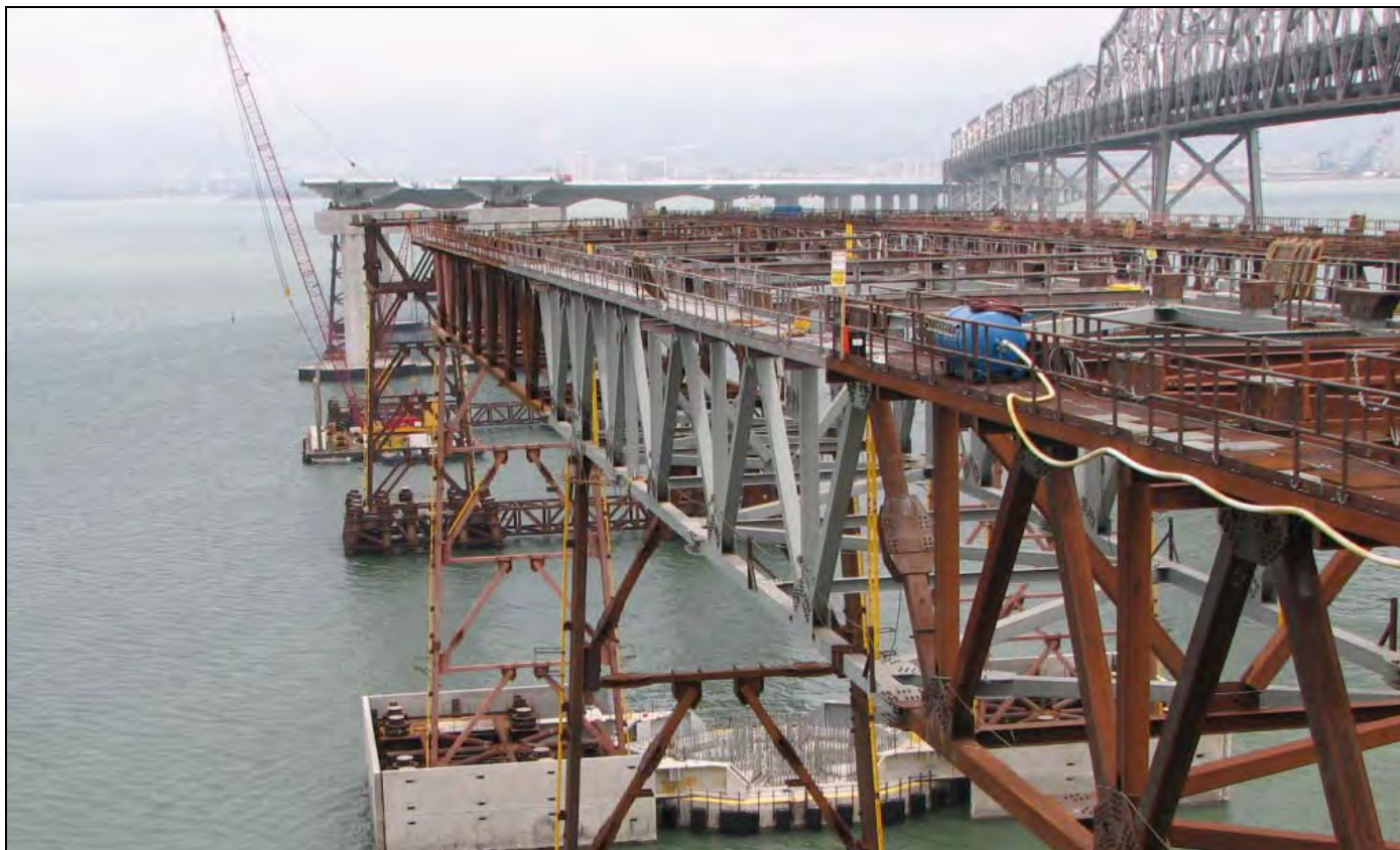
Temporary Truss Erection Westbound
