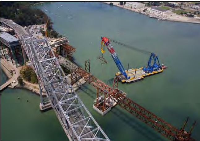
Shear-Leg Barge Crane Placing Temporary E Line Truss (D to F)
