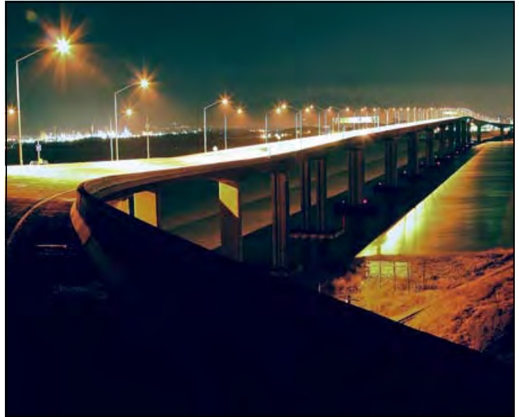
New Benicia-Martinez Bridge Opened to Traffic in August 2007
