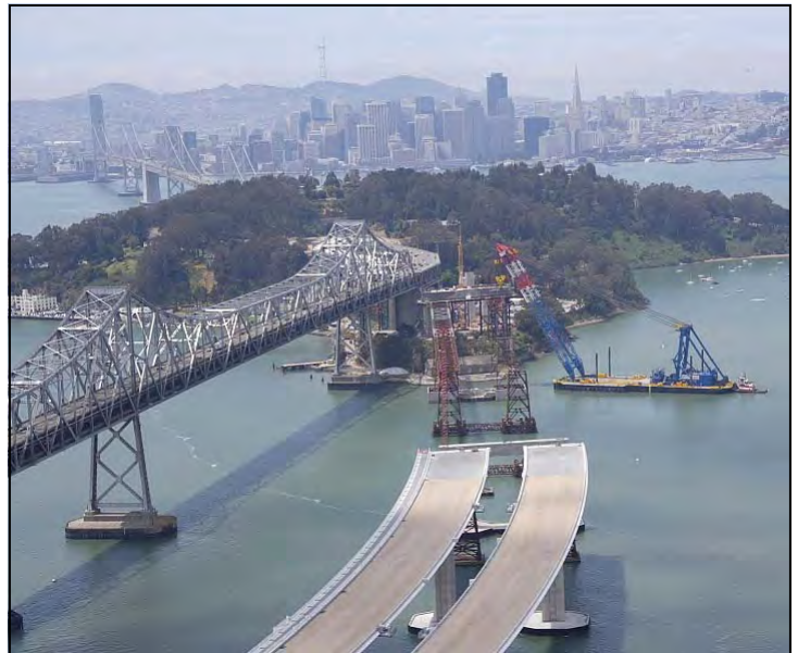
Western End of Completed Skyway
