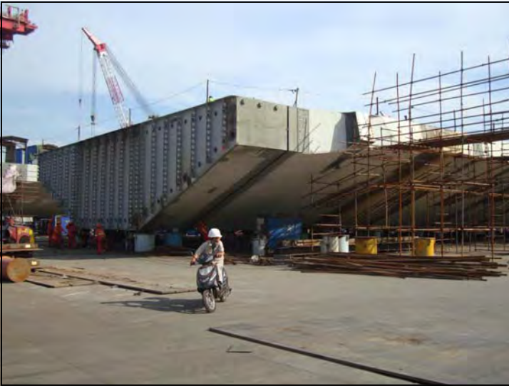
SAS Tower Fabrication OBG Segment 1AA
