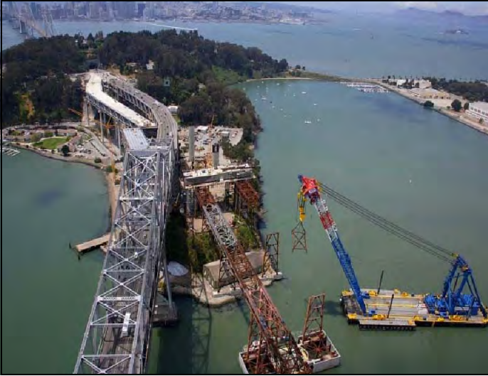
Temporary Tower Truss Erection with Shear-leg Barge Crane
