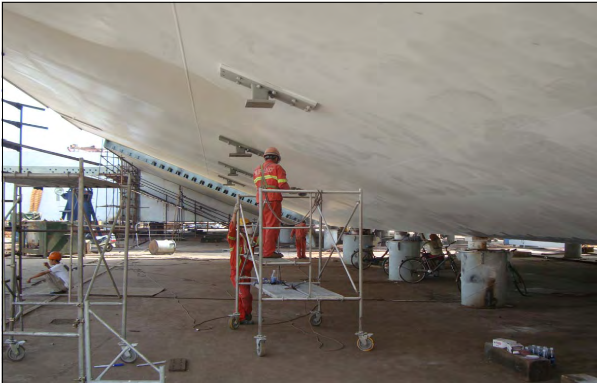
OBG Deck with Lifting Mechanism Being Installed
