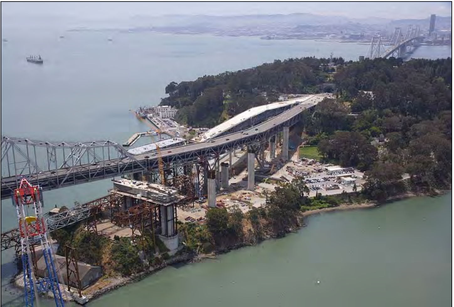
YBITS Advanced Foundation and Column Work in Progress
