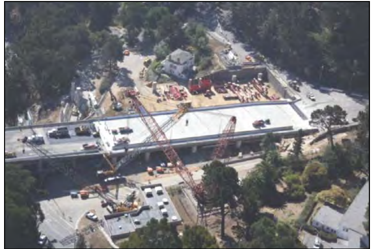
Successful Labor Day Weekend 2007 Roll-In of Replacement Tunnel Approach Roadway
