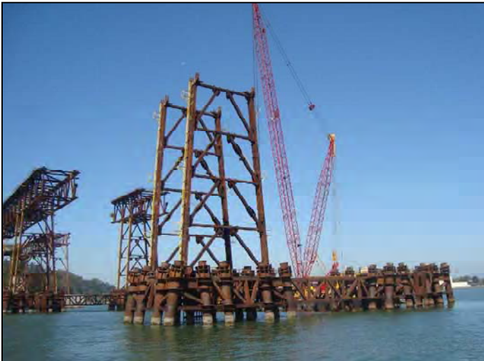
Temporary Truss Erection off of Yerba Buena Island
