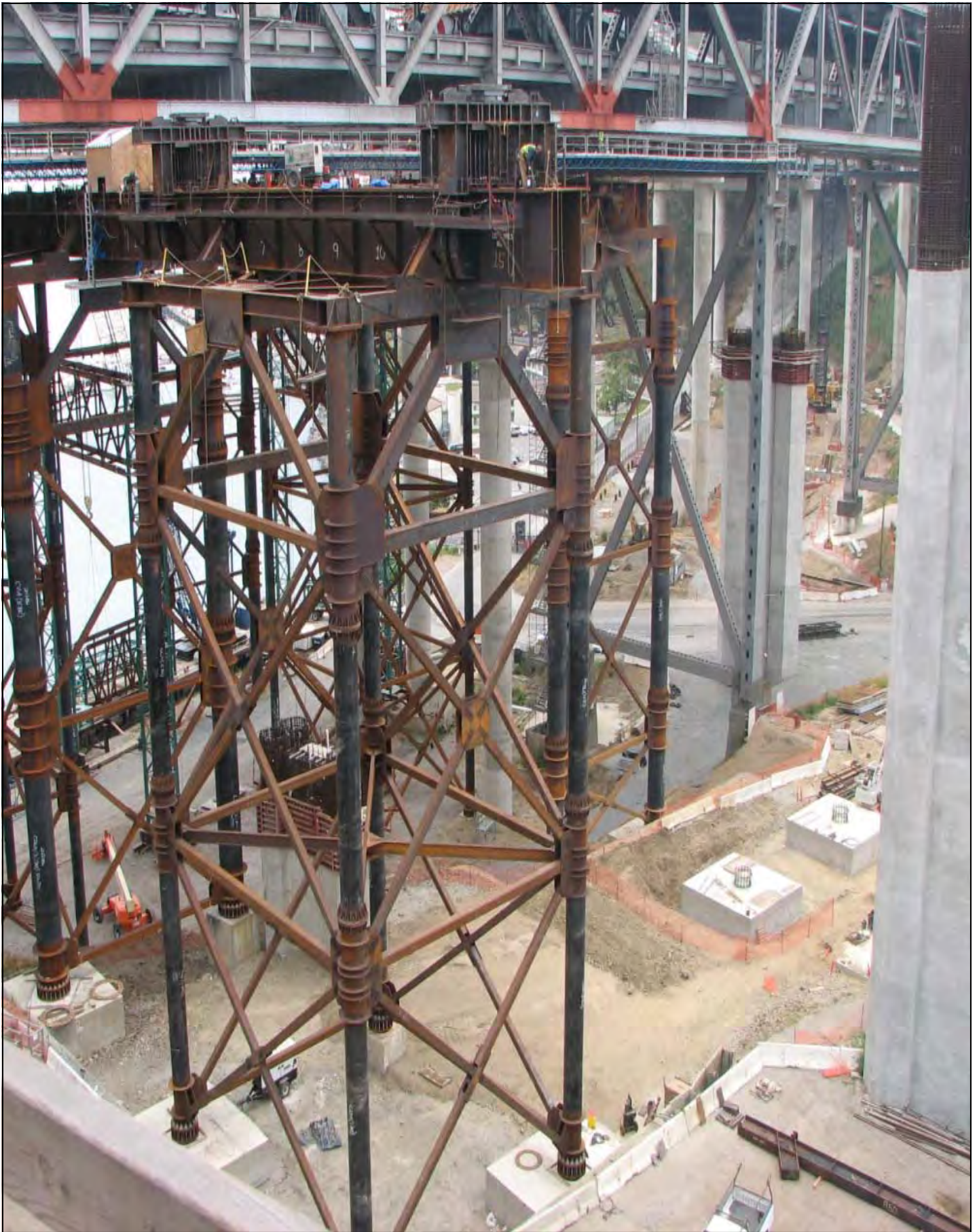
Skid Bent Structure
