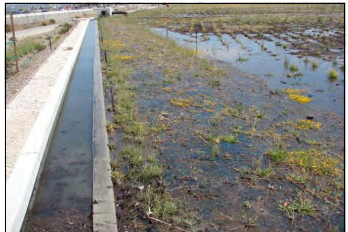
Storm Water Retention Basin
