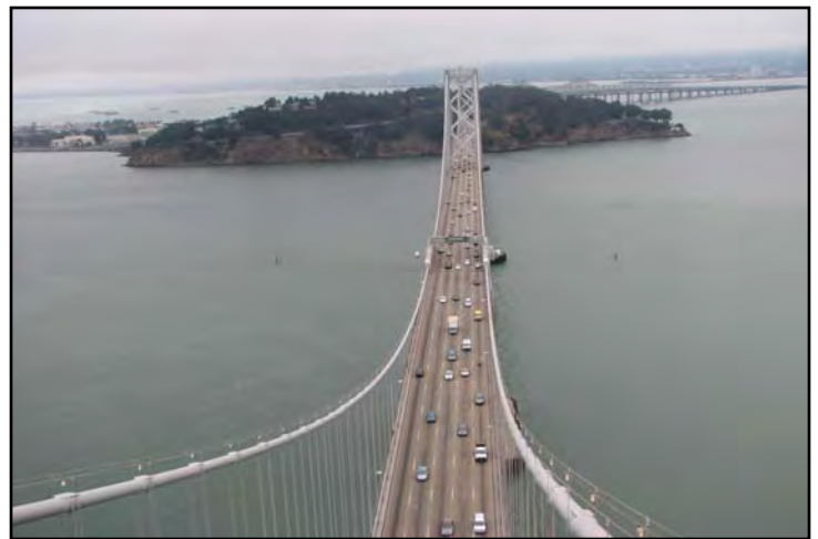
West Span of the Bay Bridge
