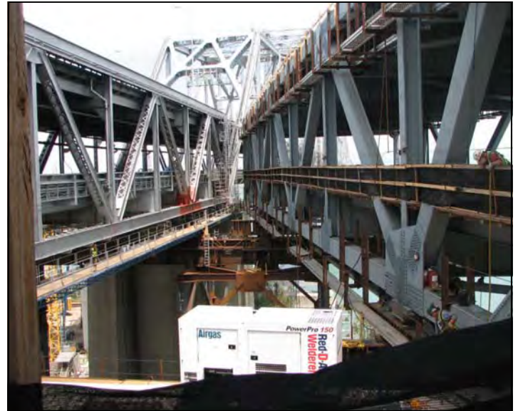
East Tie-In Truss Erection
