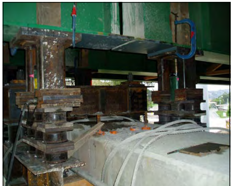
Mococo Bridge Jacking
