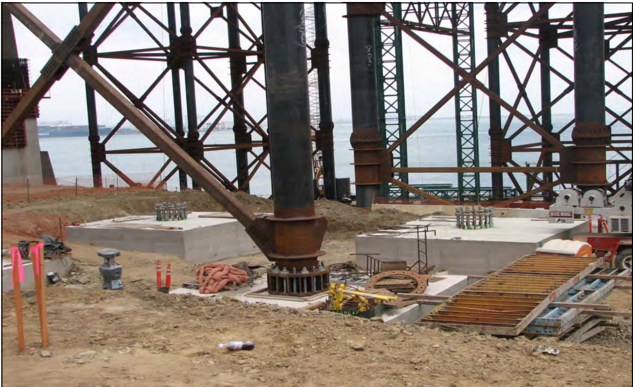
East Tie-In Skid Bent Line A Footings
