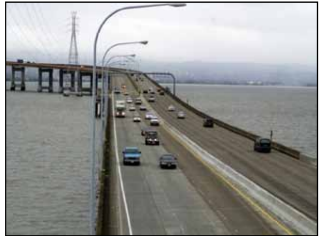
High-Rise Section of San Mateo-Hayward Bridge
