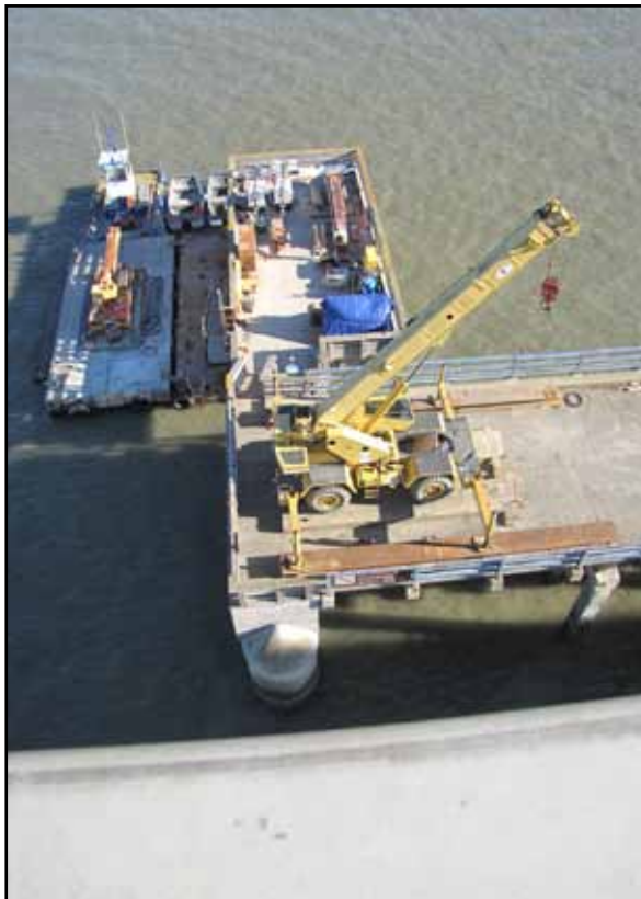
Ravenswood Staging for Footing Overlay Work
