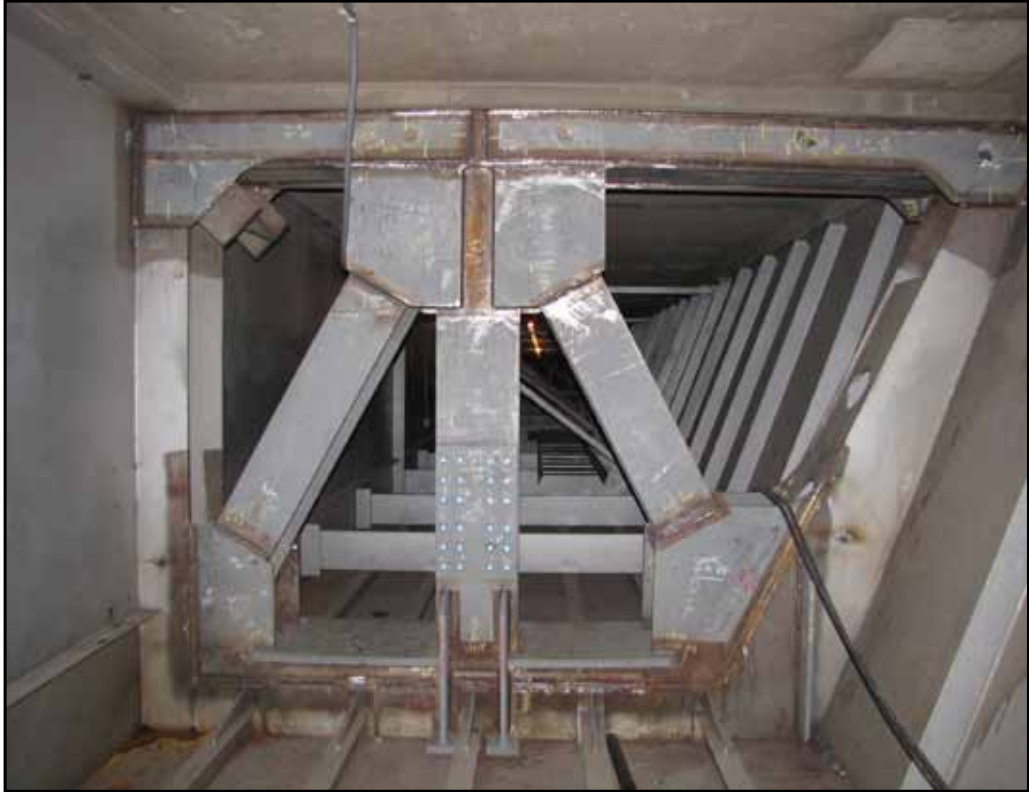
Pier 28 Jacking Frame
