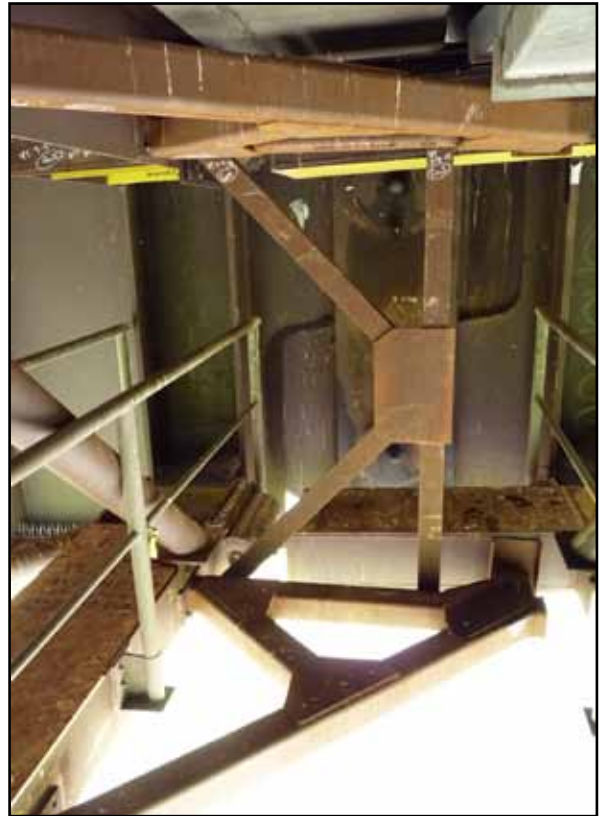
Internal Shear Keys Installed to Prevent Bending of Pin Hangers
