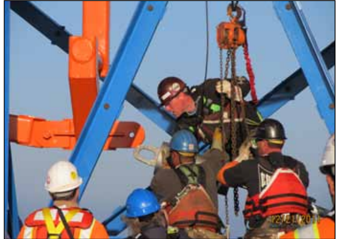
(2) Connecting the Cable Strand Lead Socket to the Hauling Arm
