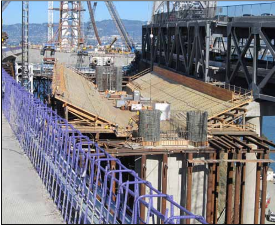
YBITS #1 Soffit Formwork and Falsework Installation in Progress
