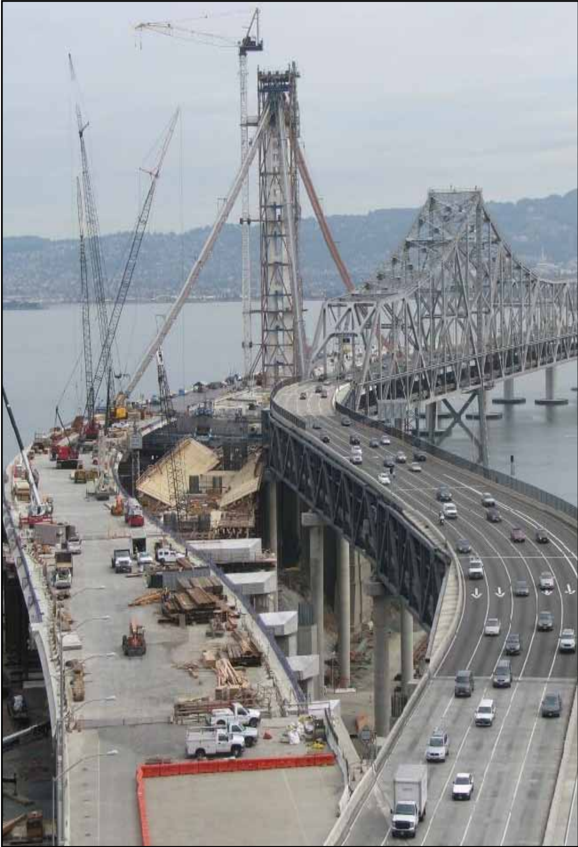
YBITS #1 Westbound Roadway Deck Nearing Completion
