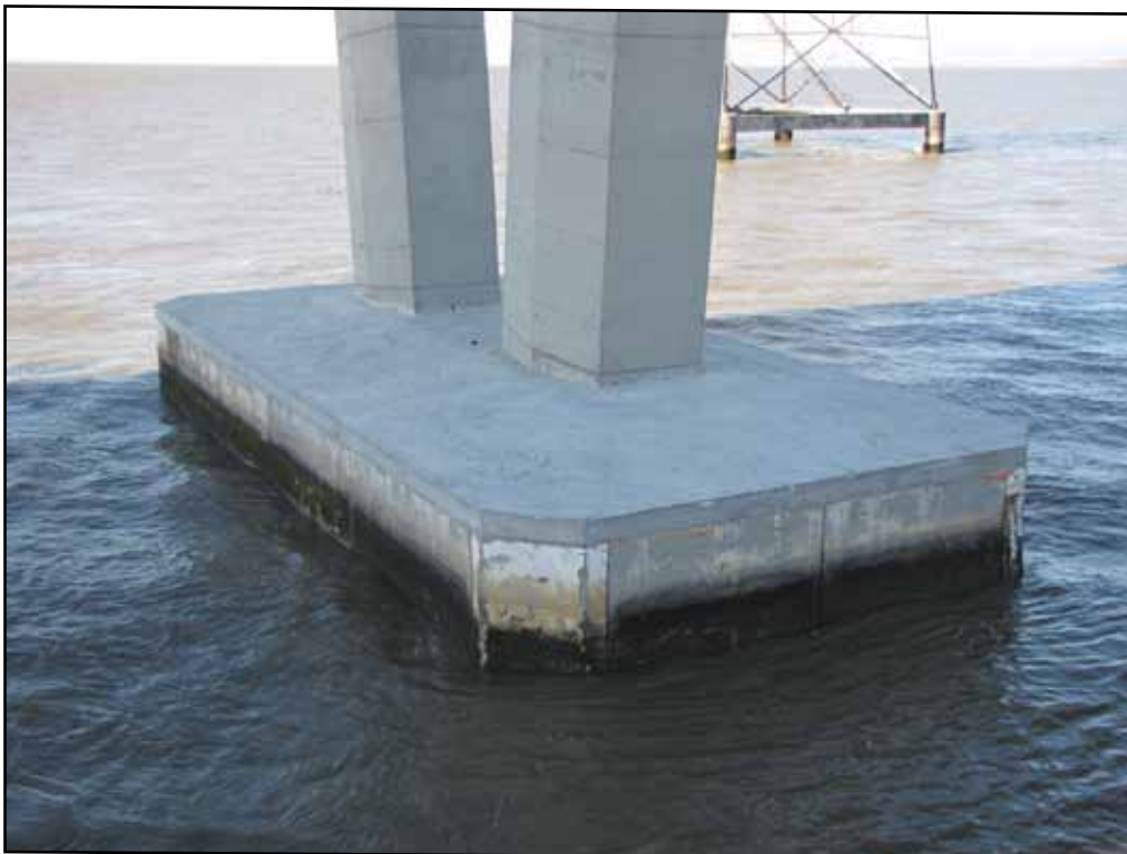
Dumbarton Bridge - Pier 26 Footing Overlay - All Footing Overlay Completed Except Piers 23 & 24
