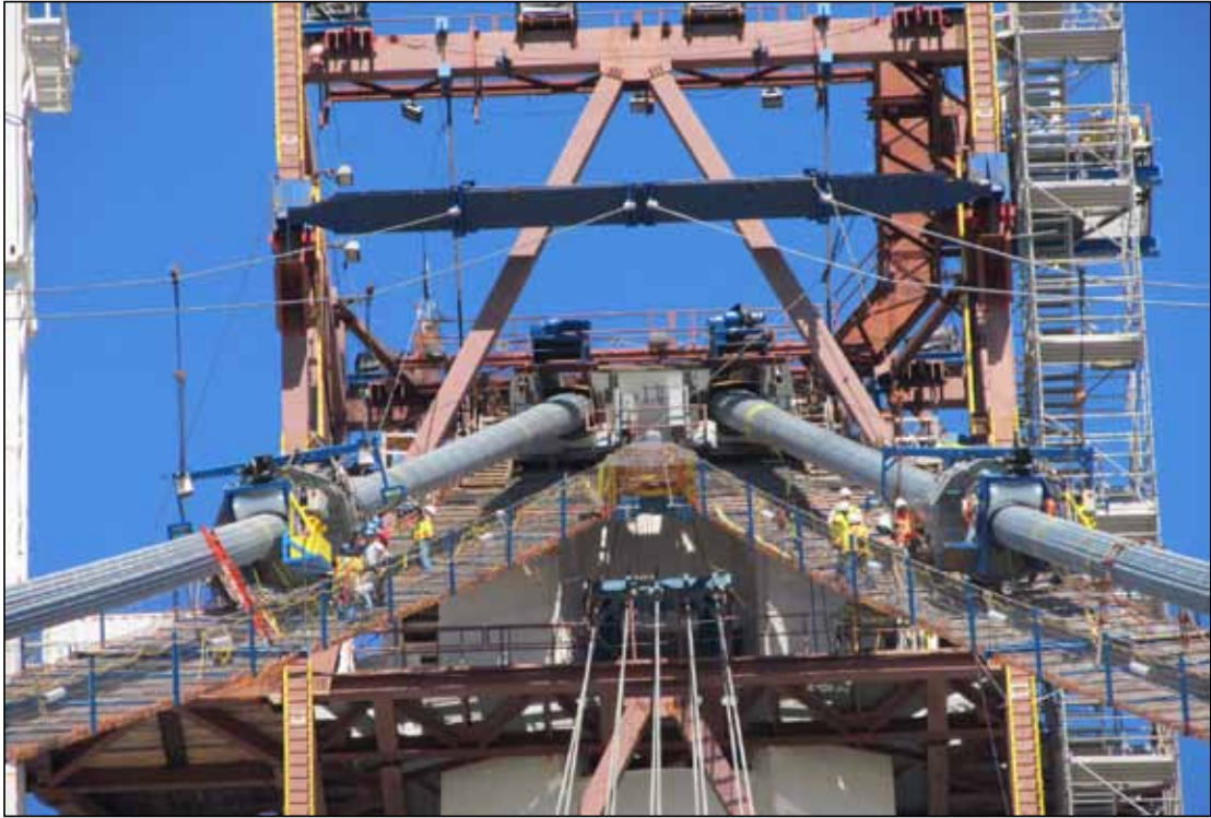
Compacting the Parallel Wire Strands (PWS)
