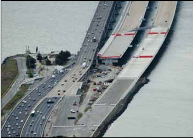
Oakland Detour - Westbound Opened to Traffic
