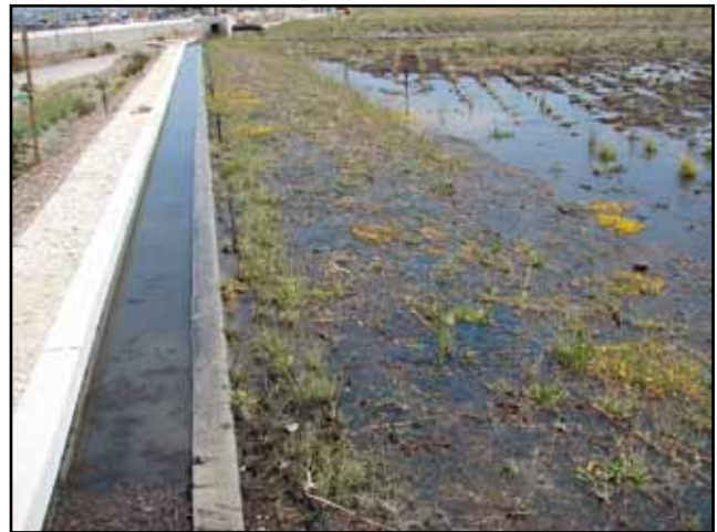
Stormwater Retention Basin
