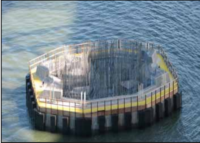
Foundation for the Self-Anchored Suspension Bridge Tower
