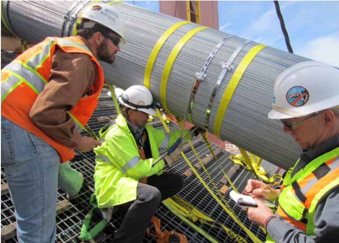
Verifying Circumference after Compaction
