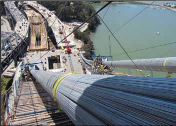
Parallel Wire Strands after Compaction
