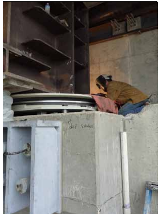
Welding of Isolation Bearing to Girder at Pier 41
