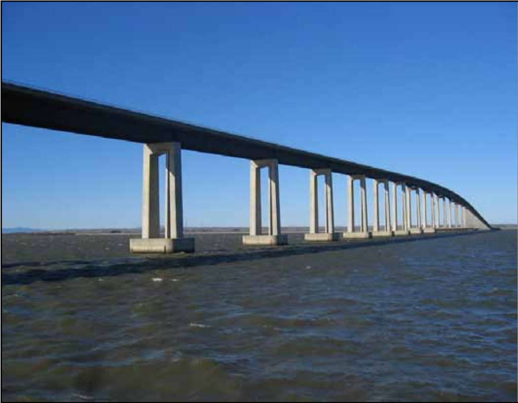
Antioch Bridge Installing Cross Bracing as Part of the Seismic Retrofit Construction
