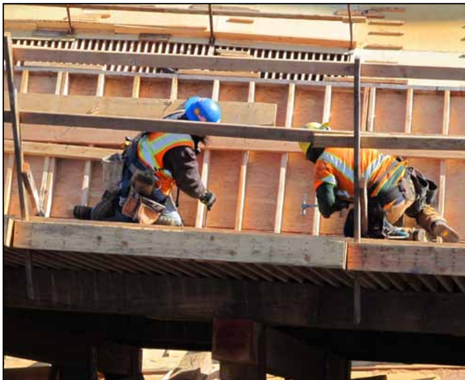
Carpenters Working on YBITS #1 Eastbound Formwork
