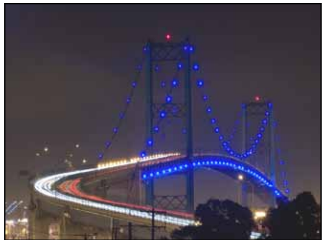
Los Angeles-Vincent Thomas Bridge
