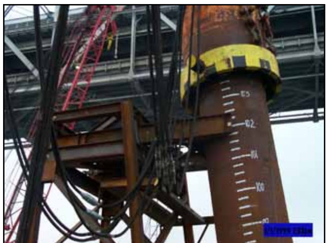
Battered Pile Installation Demonstration
