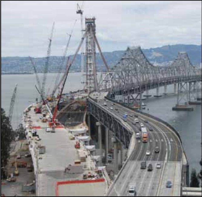
YBITS #1 Nearly Completed Westbound Roadway Deck Construction
