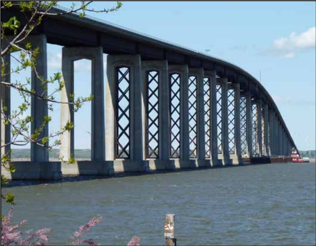
Antioch Bridge with Completed Cross Bracings
