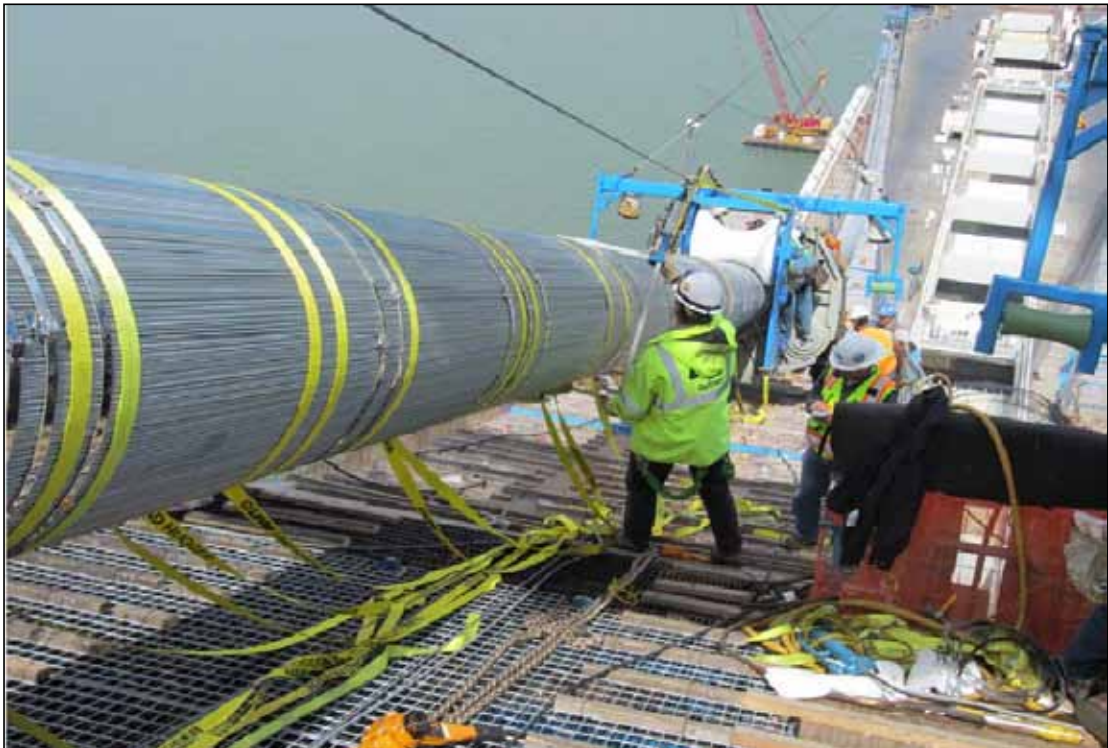
North Main Compactor - Checking Circumference after Compaction
