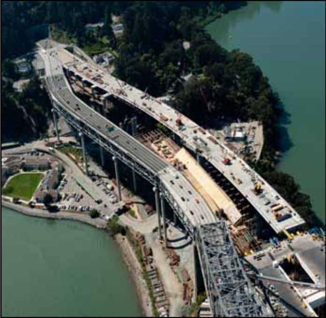
YBITS #1 Roadway Deck Construction in Progress
