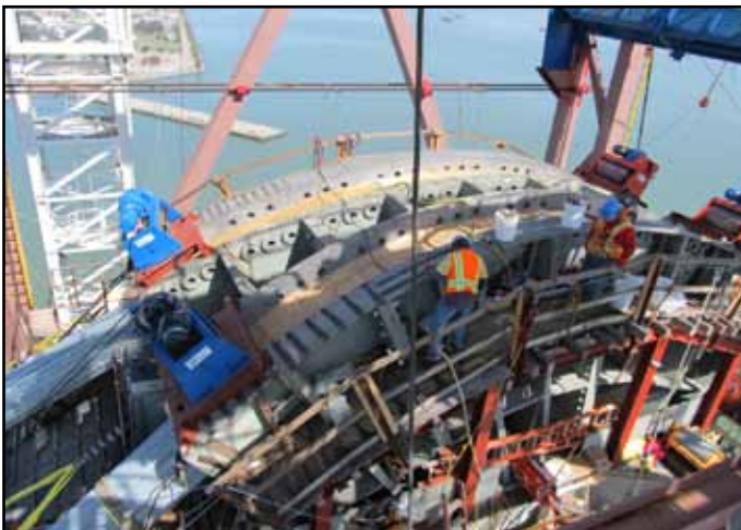
Self-Anchored Suspension Bridge Tower Saddle Housing Placed
