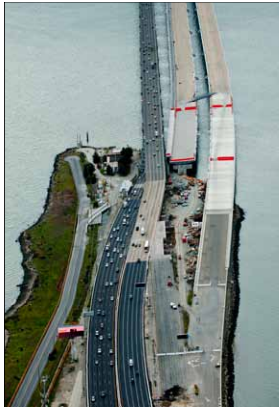
Aerial View of the Eastbound Oakland Detour with the EBMUD Outfall Crossing Structure on the left and the Westbound Oakland Detour Open to Traffic
