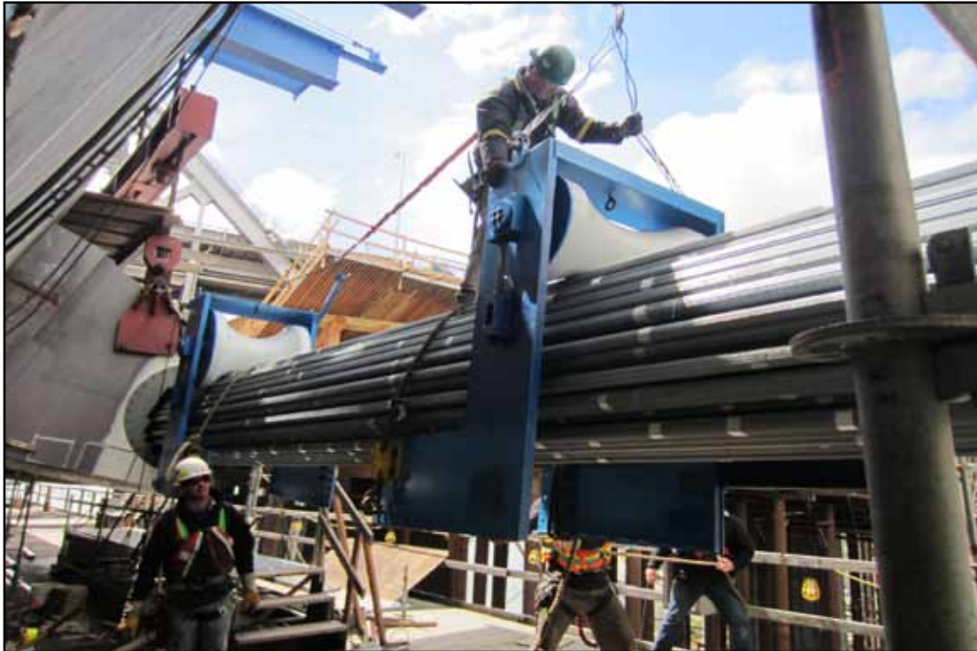
Installing Cable Compaction Rollers at West end
