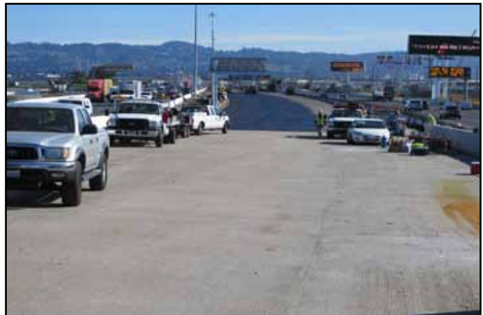
Oakland Westbound Detour (Looking East) AC Asphalt Installed
