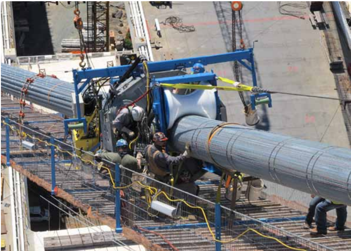
Cable Strands Being Compacted
