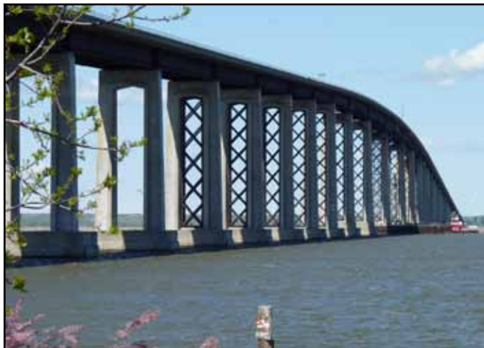
Antioch Bridge Seismic Retrofit
