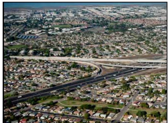
Aerial View of Construction Progress
