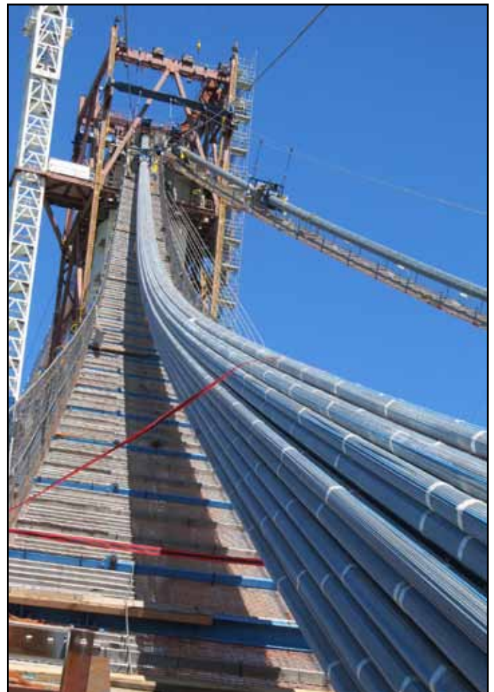
Parallel Wire Strand (PWS) before Compaction
