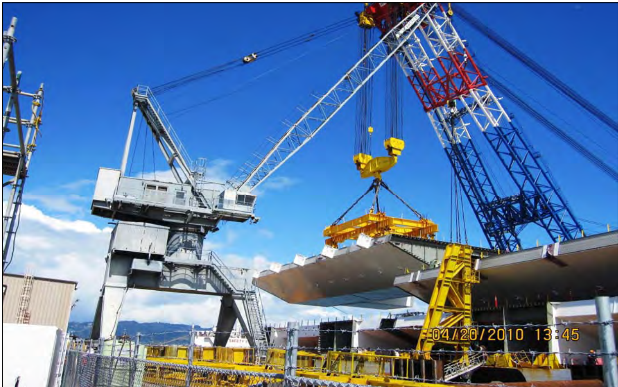
SAS - Offloading Roadway Box 5 East
