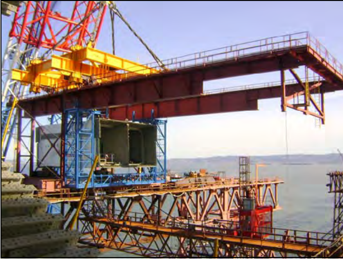
SAS - Crossbeam(CB)1 Being Placed on Temporary Support Structure
