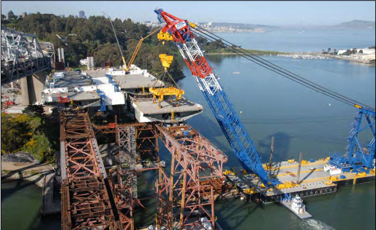
SAS - Roadway Box 4 West Being Placed on Temporary Support Structures
