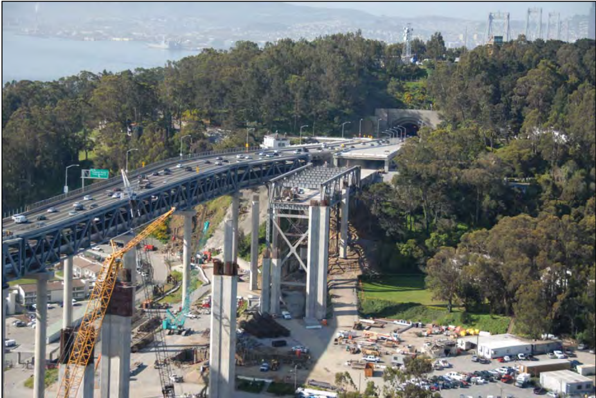
Aerial View of Demolition of Existing Bridge
