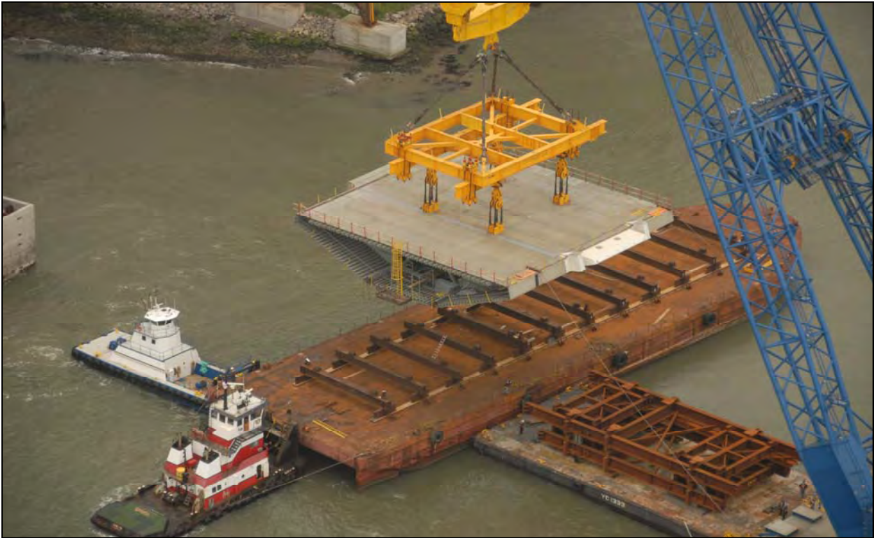
SAS - Roadway Box 4 West Being Lifted onto the Temporary Support Structures
