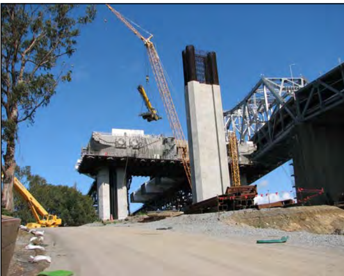
SAS - W2 Cap Beam and YBITS Column W3L
