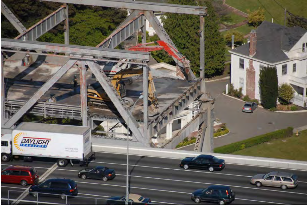
Aerial of Existing Bridge Demolition
