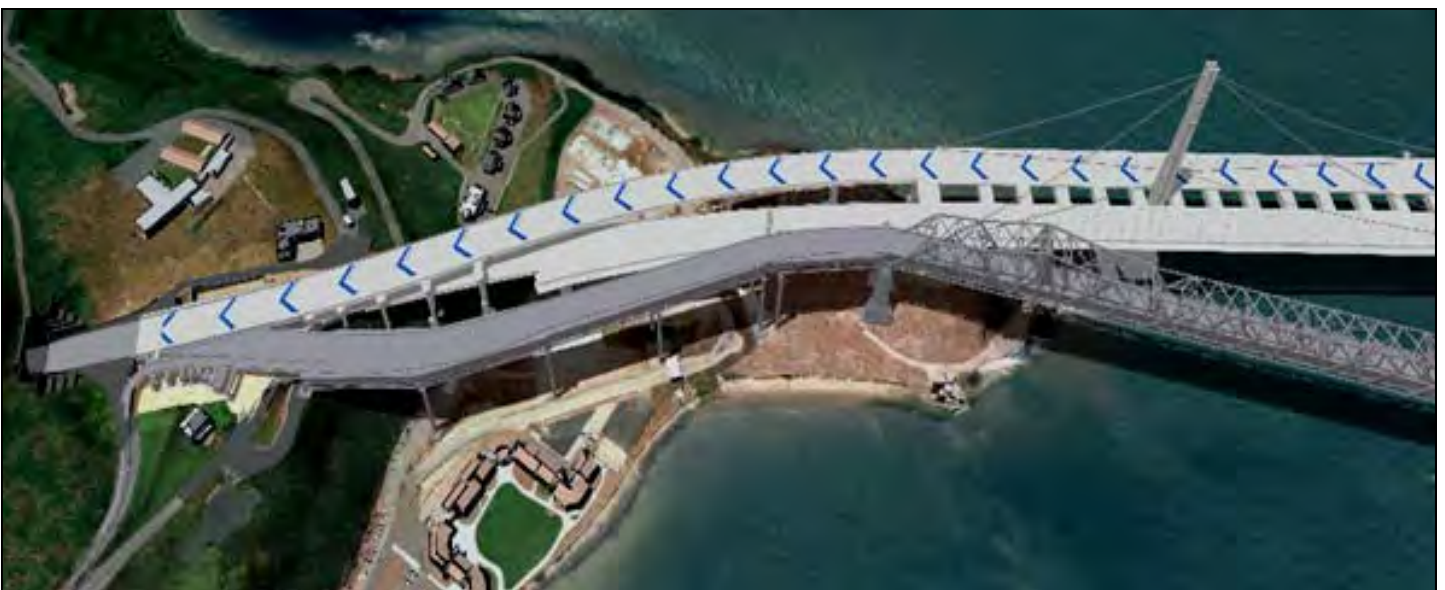
Rendering of Overview of Future Yerba Buena Island Transition Structures (top), in progress with Detour Viaduct (bottom) Completed
