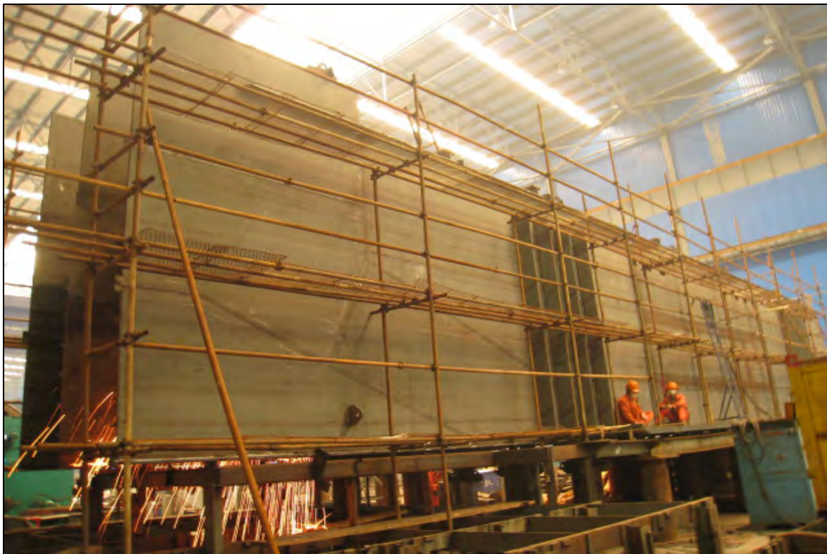
SAS - Roadway Box 13 Constructability Model in Bay 13
