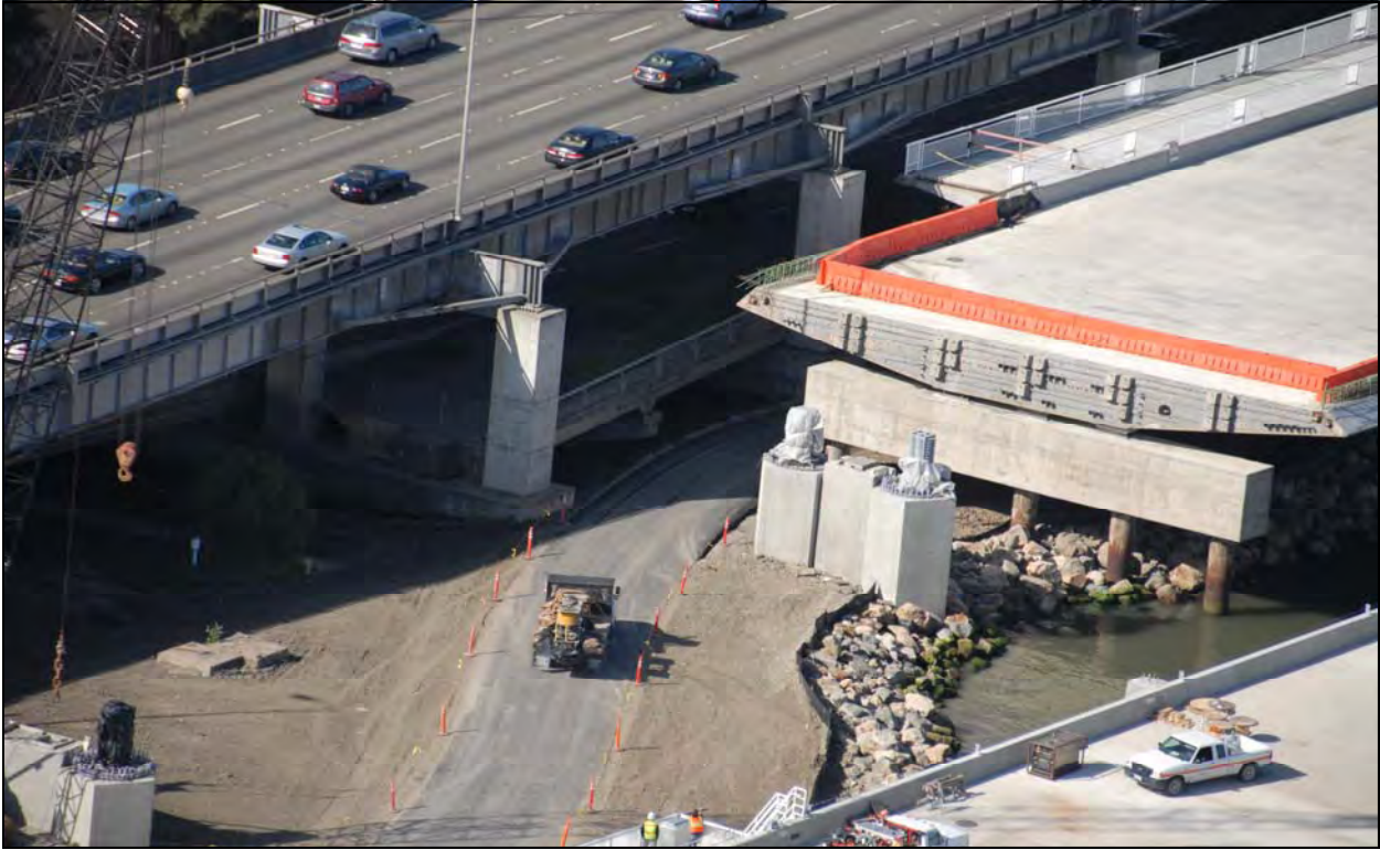
Oakland Touchdown #1 Overview of Completed Temporary Access Road OTD #1
