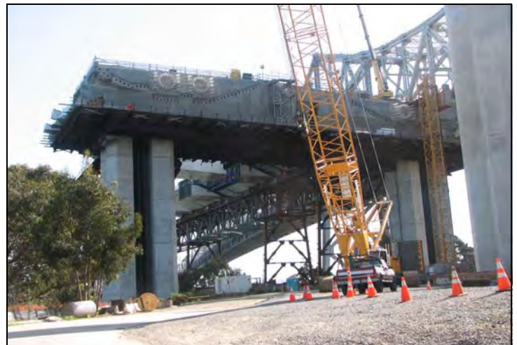
SAS W2 Cap Beam
