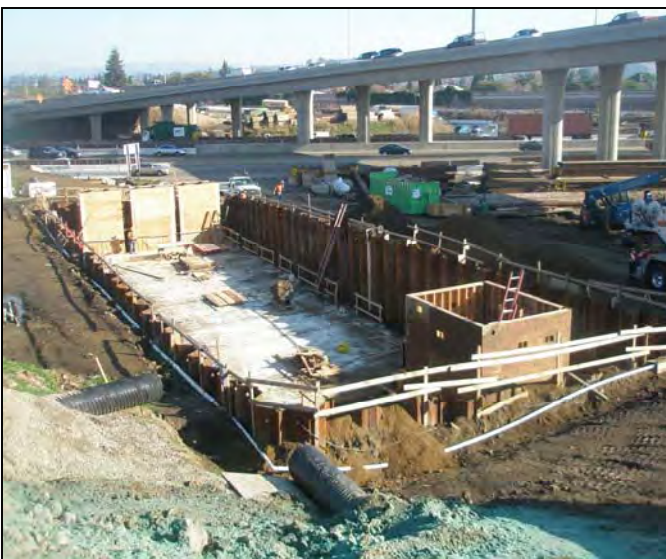
92/880 Pump Station Construction in Progress
