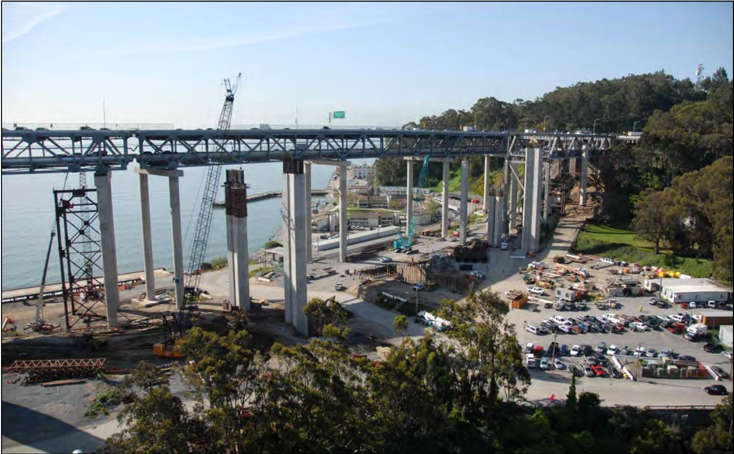
Yerba Buena Island Transition Structures
