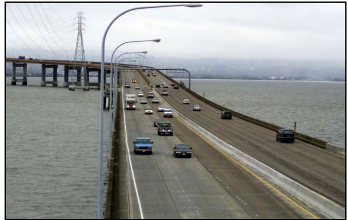
High-Rise Section of San Mateo-Hayward Bridge
