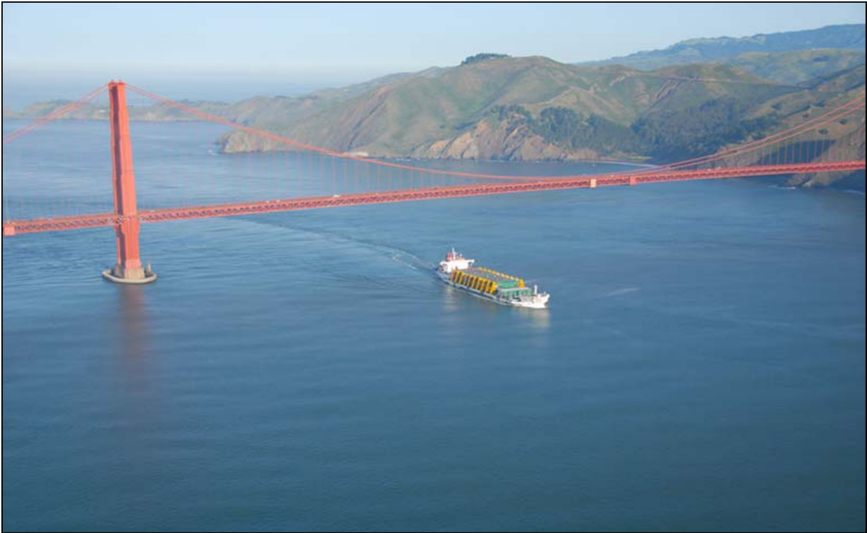
SAS- Arrival of Roadway Box 5 and 6 East and West Shipment #2
