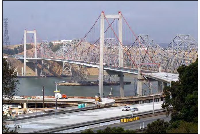
New Alfred Zampa Memorial (Carquinez) Bridge Soon after Opening to Traffic, with Crockett Interchange Still under Construction
