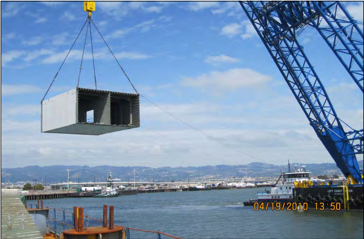
SAS- Offloading Crossbeam
