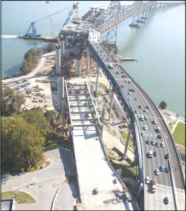
Demolition of Existing Bridge
