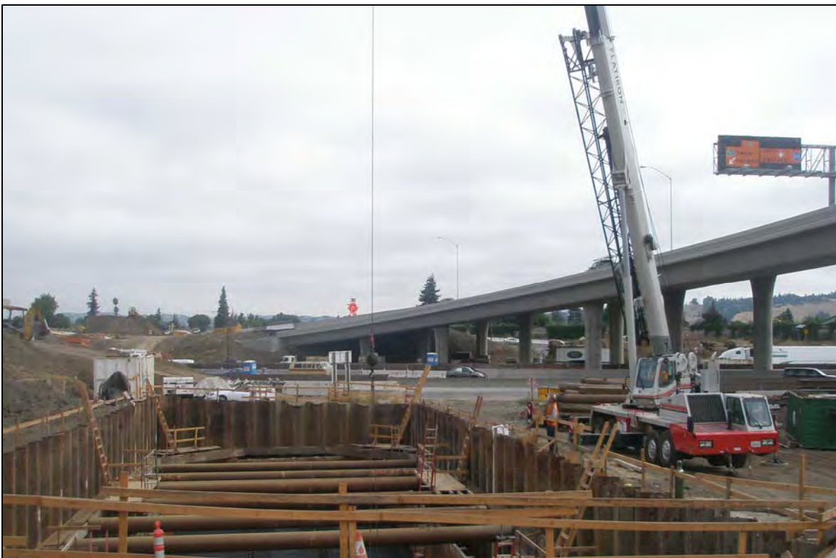
92/880 Widening at Mount Eden Overhead Crossing
