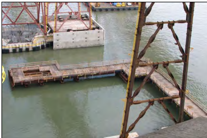
SAS T1 Trestle Overview
