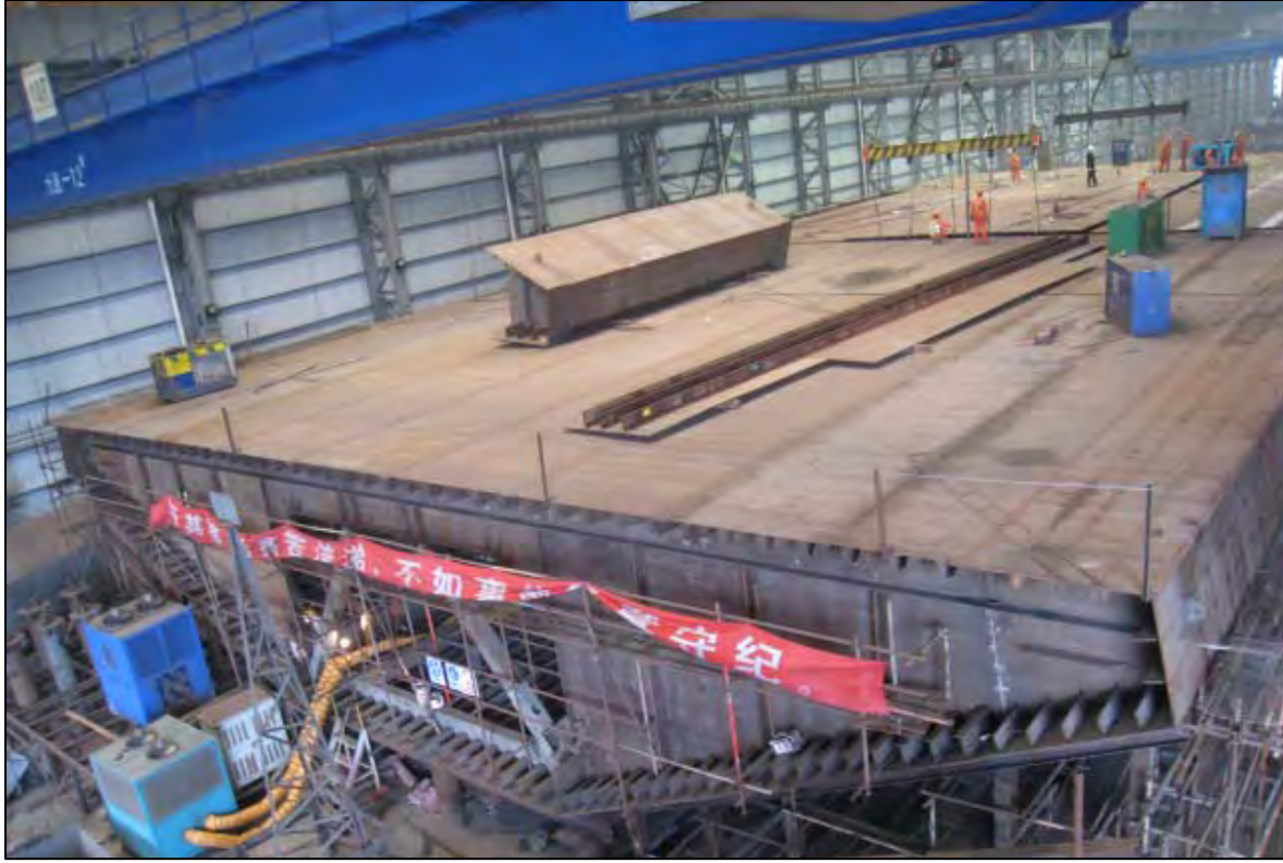
SAS - Overview of Roadway Box 11 & 12 East Line Assembly in Bay 14
