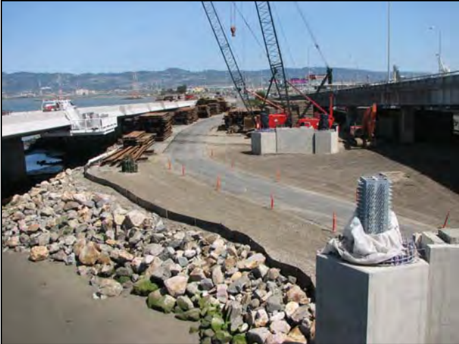
Oakland Touchdown #1 Newly Paved Temporary Access Road to Skyway
