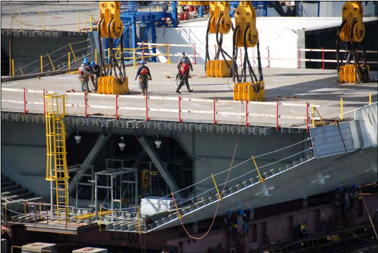
SAS Roadway Box Placement
