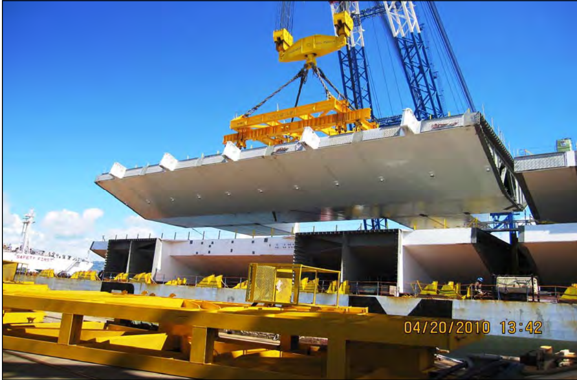
SAS—Offloading Roadway Box 5 East
