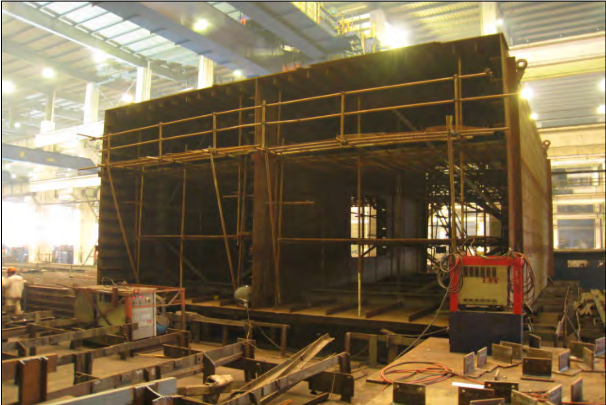
SAS - Crossbeam 15 Assembly in Bay 1
