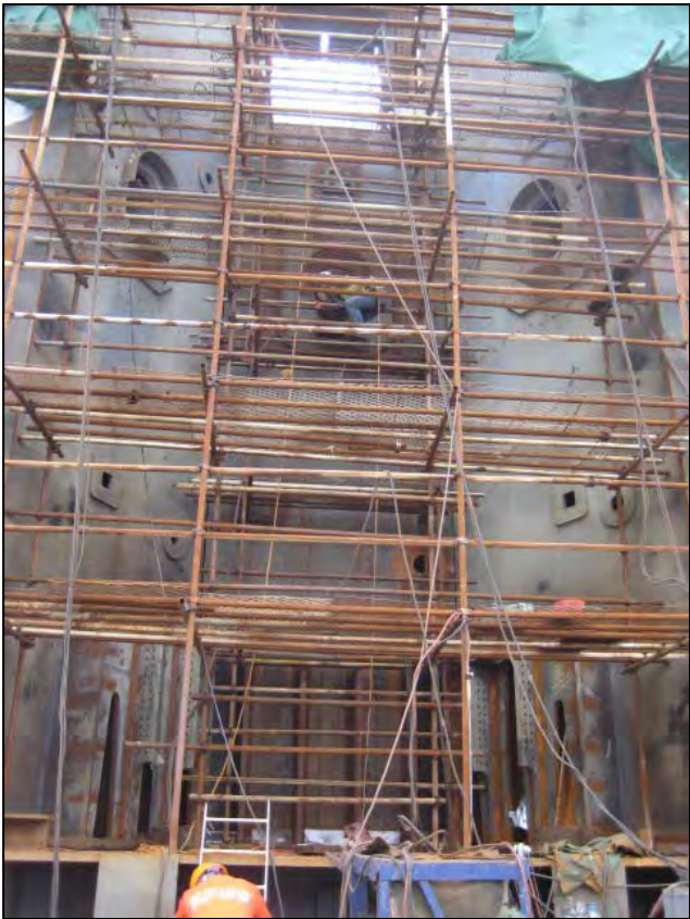
SAS Preassembly of Base Shear Plate
