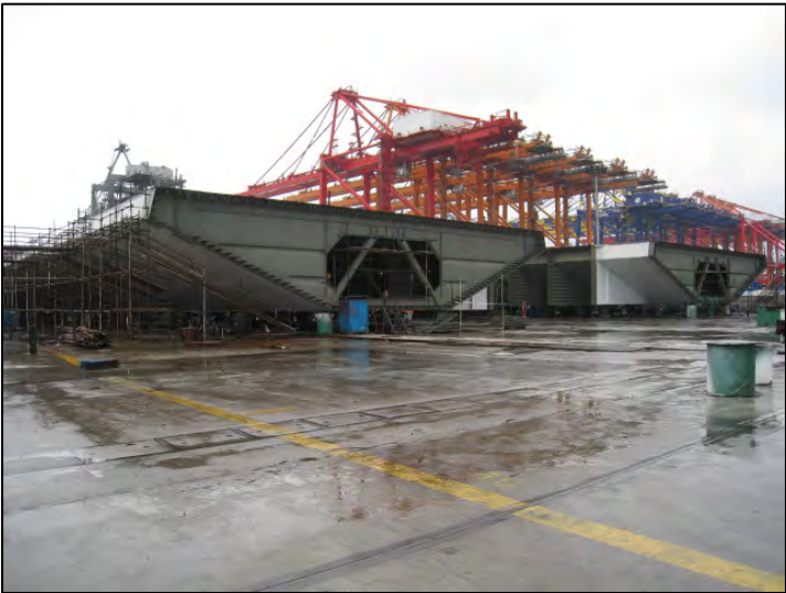
SAS Roadway Boxes 5 and 6 Being Prepared for Shipment
