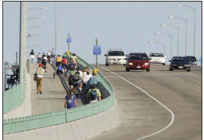
Benicia-Martinez Bridge Pedestrian/Bicycle Pathway Opened to The Public in August 2009
