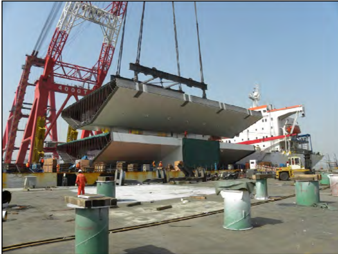
SAS - Roadway Boxes
