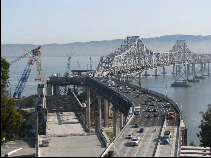
SFO Bay Bridge Detour Structure Completed over the Labor Day Weekend
