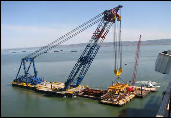
Shear-Leg Barge Crane Lifting Roadway Box Lift 1 East
