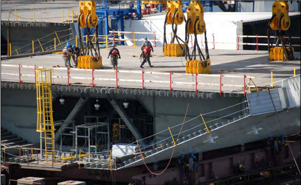
SAS - Positioning Roadway Box 4 West onto the Temporary Support Structures
