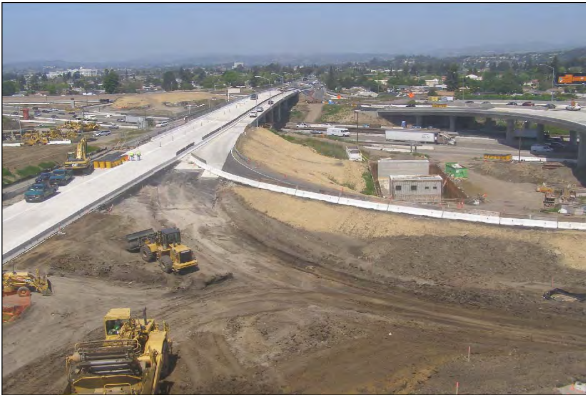
92/880 Site Preparation of New Route 92 and Interstate 880 Separator
