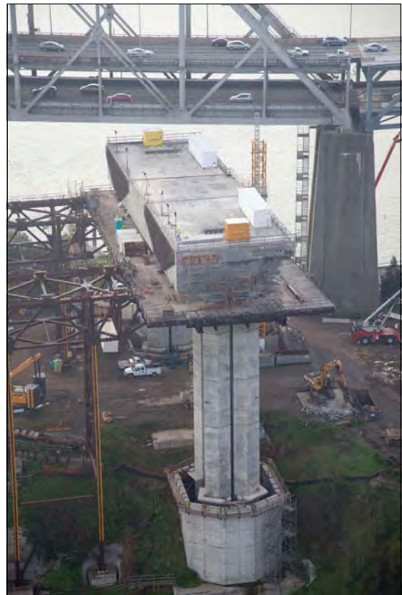
SAS Overview of W2 Cap Beam
