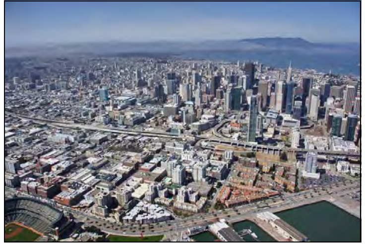
Overview of the Completed West Approach Replacement Structure
