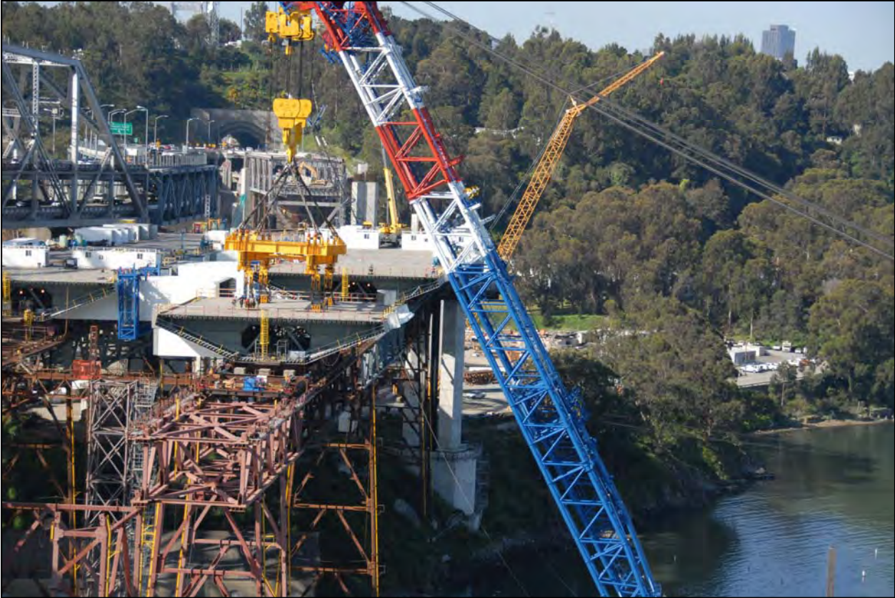
SAS Roadway Box Placement
