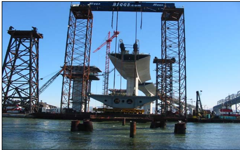
Skyway Orthotropic Box Girder
