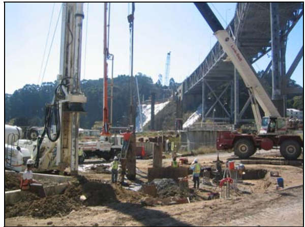
Drilling for CIDH piles for Bent 53
