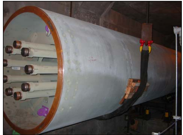
Hinge Pipe Beam on Temporary Support
