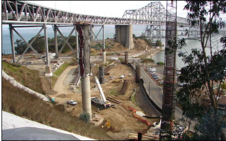
Viaduct portion of SSD
