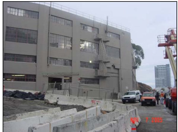
Harrison St. Off-ramp Demolition 6
