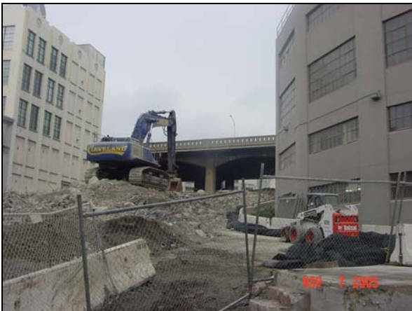
Harrison St. Off-ramp Demolition 5
