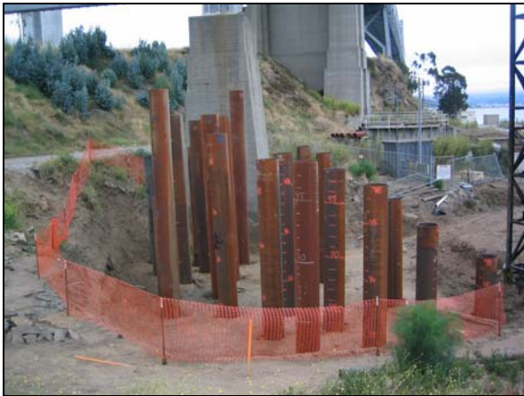
Piles for Bent No. 52
