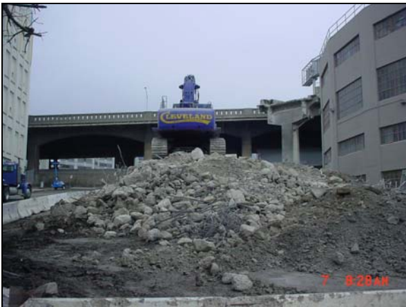
Harrison St. Off-ramp Demolition 3
