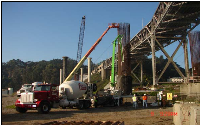
Construction of columns for the viaduct portion of SSD
