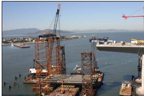
Aerial View of Skyway Construction
