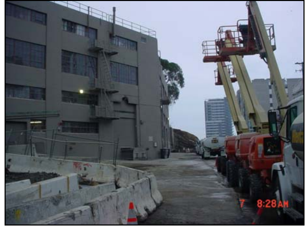
Harrison St. Off-ramp Demolition 2
