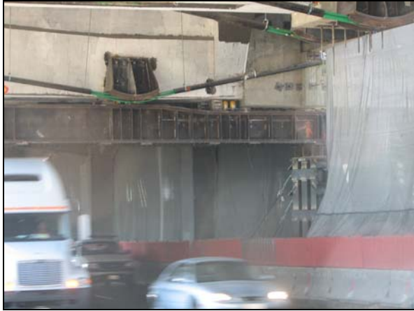
Temporary Support Frame (Super Bent at Bent #43) 1
