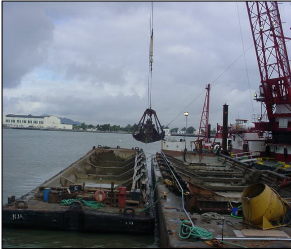
Drilling Operations for T1 Foundations
