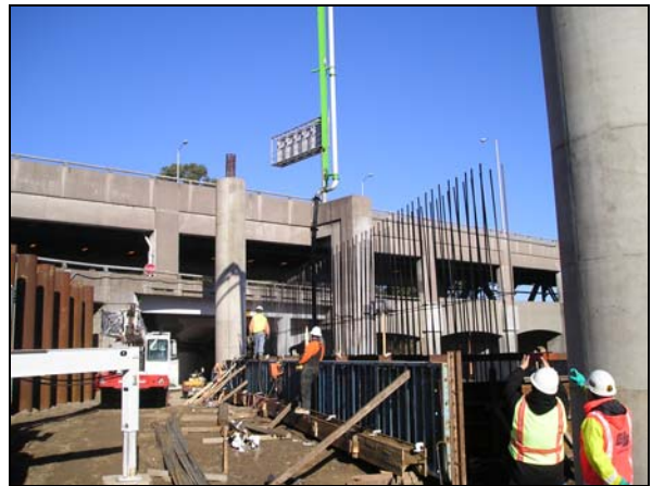
SoSoDet - Construction of Bent 48 grade beams along the former Southgate Road on Yerba Buena Island
