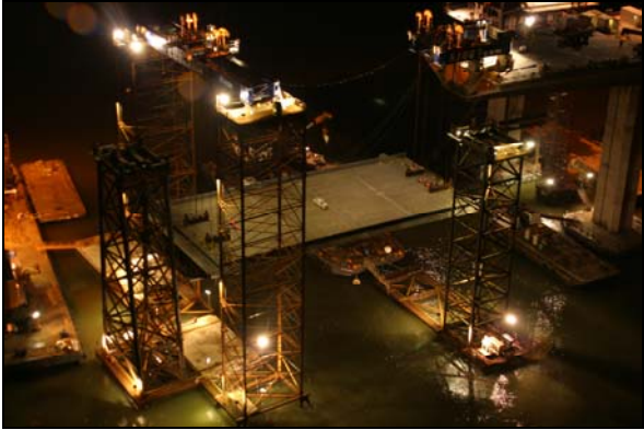
Skyway Orthotropic Box Girder
