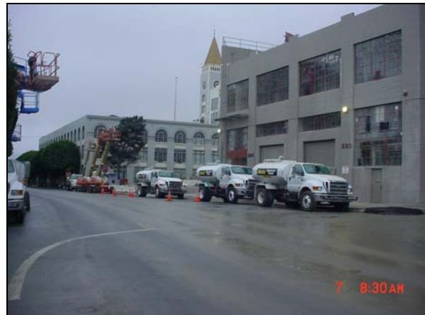
Harrison St. Off-ramp Demolition 4
