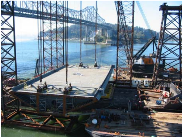
Skyway Orthotropic Box Girder
