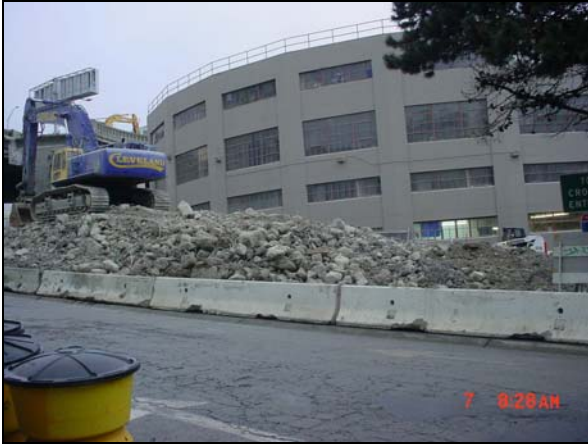
Harrison St. Off-ramp Demolition 1
