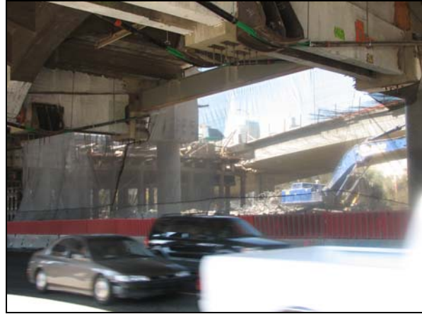
Temporary Support Frame (Super Bent at Bent #43) 2
