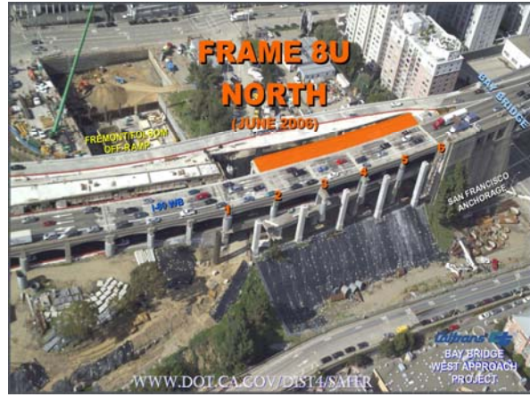
West Approach Frame 8U North
