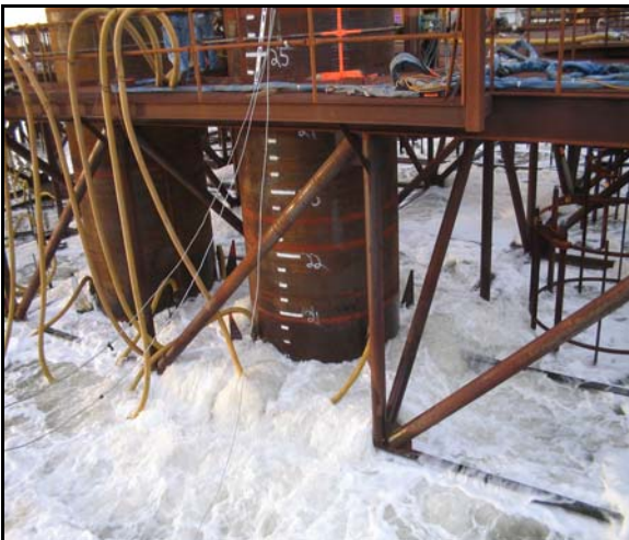
Bubble Curtain used for Installation of T1 Temporary Casings
