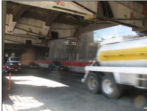
Temporary Support Frame (Super Bent at Bent #43) 3
