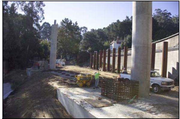
Footing and Pier Columns for Bent 48
