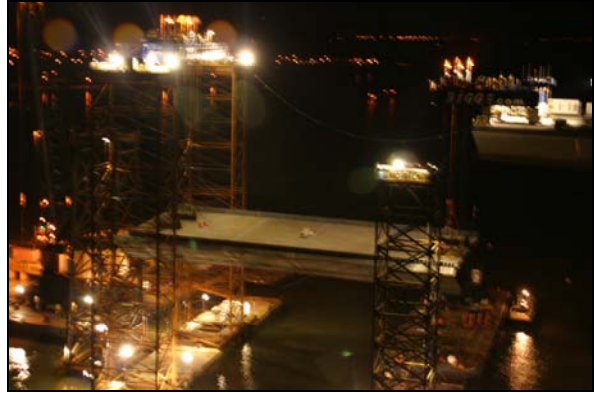
Skyway Orthotropic Box Girder
