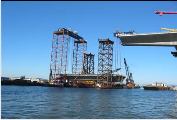
Skyway Orthotropic Box Girder
