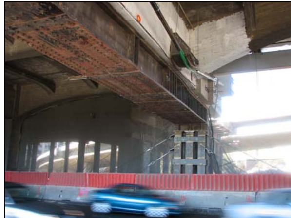
Temporary Support Frame (Super Bent at Bent #43) 4
