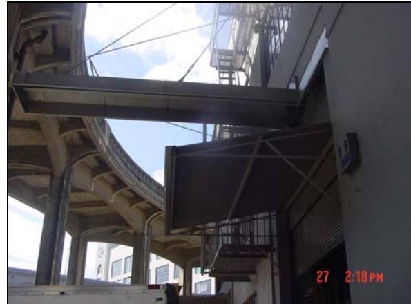
Harrison St. Off-ramp Pre-demolition 1
