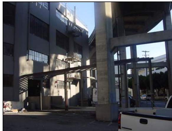
Harrison St. Off-ramp Pre-demolition 2
