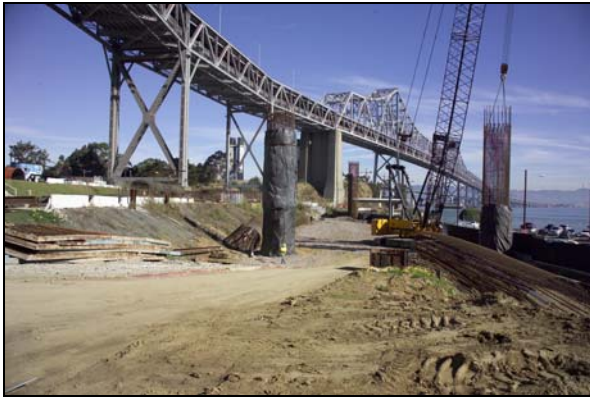
Pier Column Construction for Bents 50 and 51
