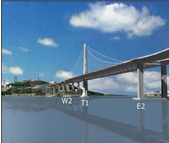
T1 = Foundation for the 530-foot steel tower E2 = Eastern Support of the suspension roadway W2 = Western Support of the suspension roadway
