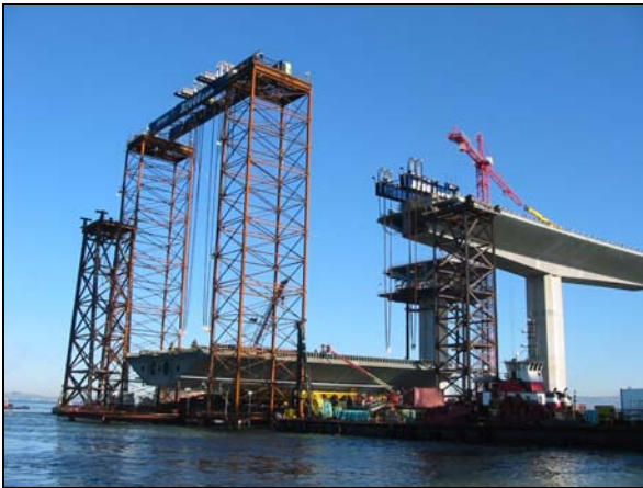
Skyway Orthotropic Box Girder
