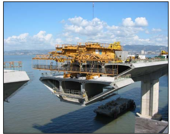
Lifting of Precast Segment for Skyway Deck
