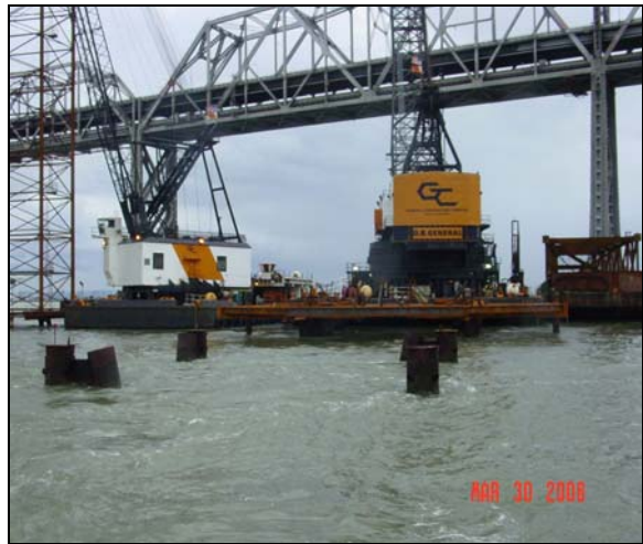
Installation of E2 Foundation Template
