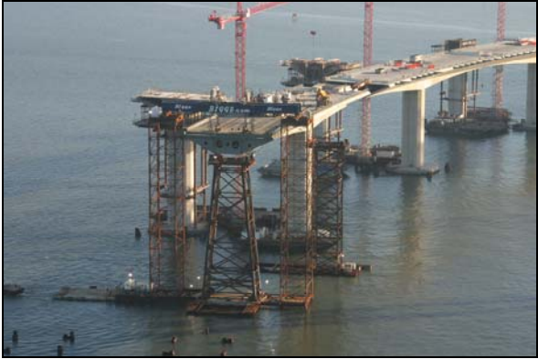
Aerial View of Skyway Construction
