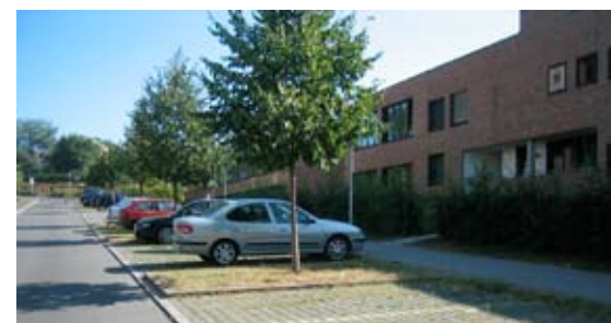
Previous pavers can be used for parking areas as well as pedestrian connections (GL-24).
