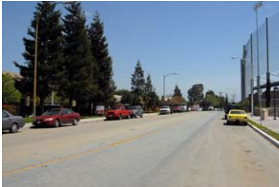
Campbell Avenue looking south.
