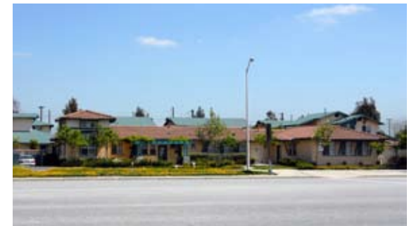
The Homesafe Family Shelter
