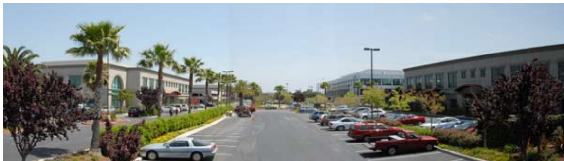
Low-rise office development built within the last ten years occupies frontage along El Camino Real and is within a three- to five-minute walk of the the station.
