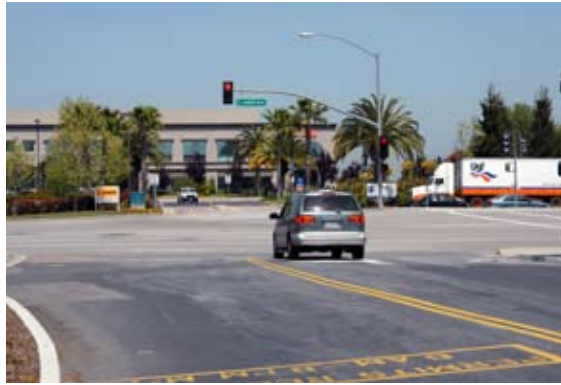
The Coleman Avenue/El Camino Real intersection will be improved with greater vehicle queuing on the east side—allowing for better access for planned residential development along Campbell Avenue.
