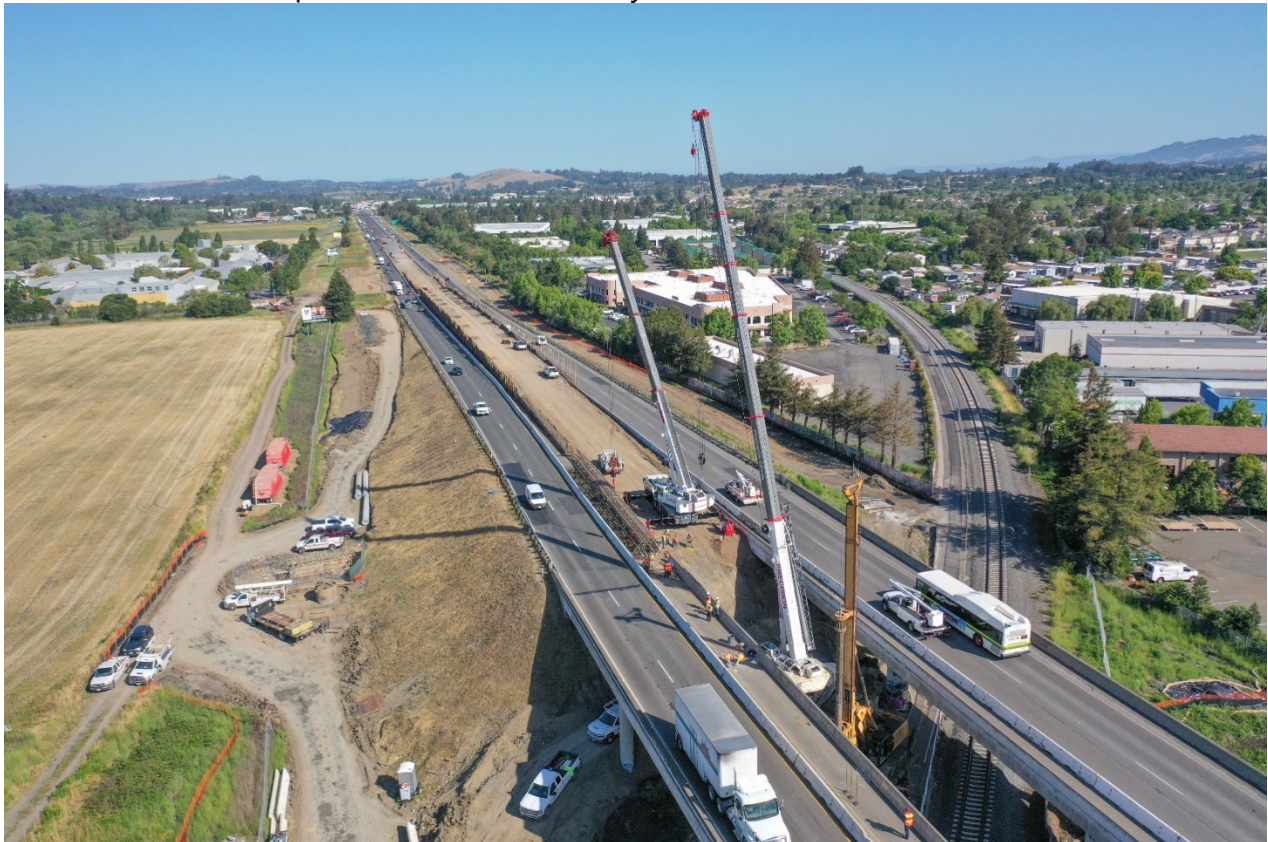
Petaluma Rail Overhead replacement, Highway 101 Under construction in 2020
