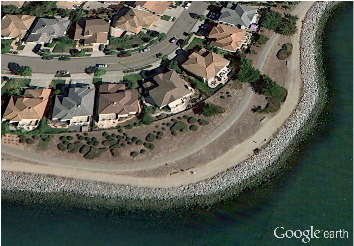
Revetment, Shoreline Park, Alameda
