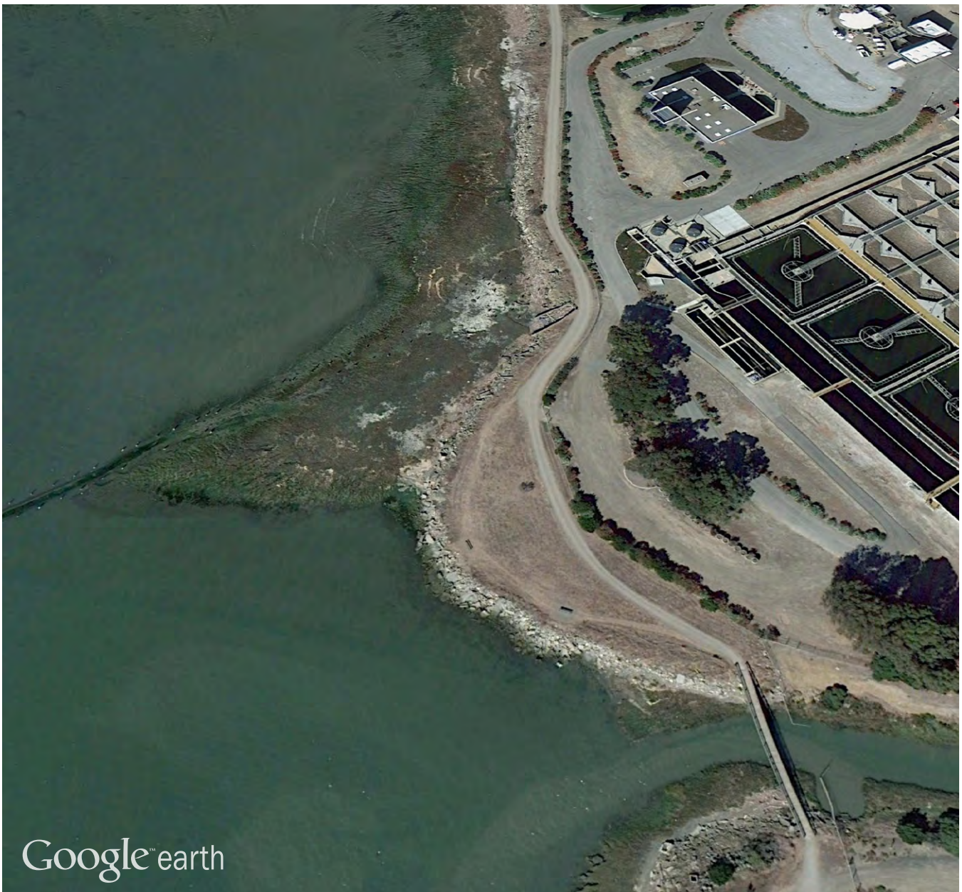
Example of a Revetment in the Pilot Project Area
