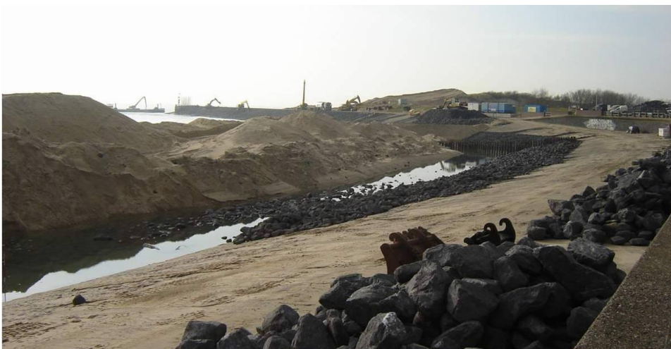
Figure 7.6 Raising Of Existing Levee
