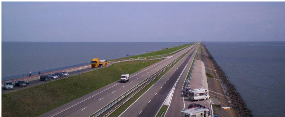
Figure 7.2 Freeway On Top Of A Levee
