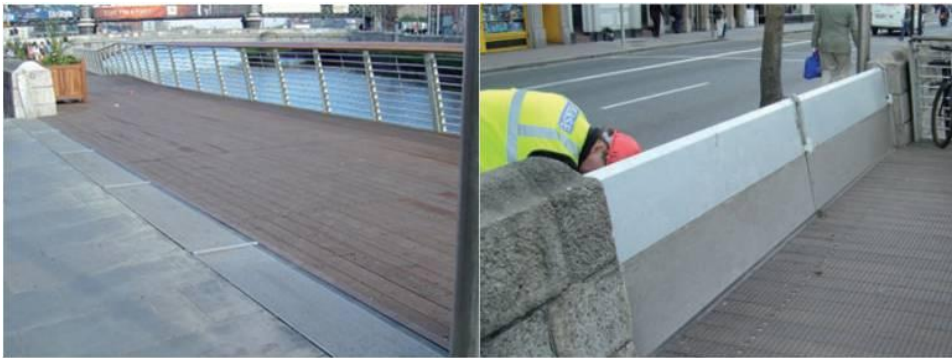
Figure 7.4 Demountable Floodwall Along Urban Waterfront
