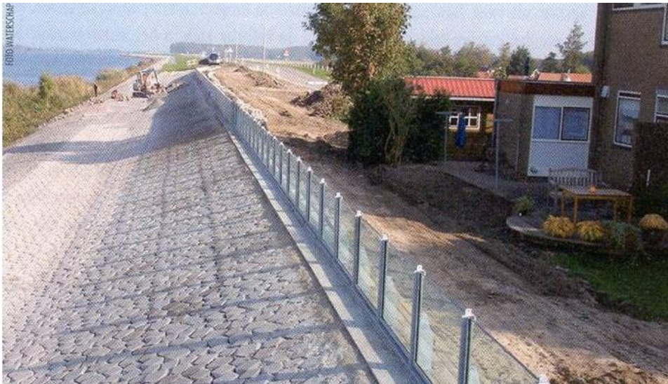
Figure 7.5 Glass Wave Overtopping Wall On A Levee
