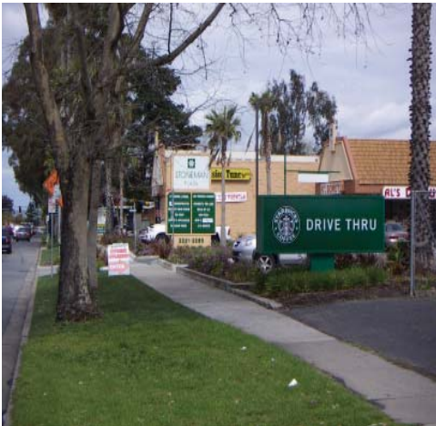
Large and inconsistent setbacks from the street contribute to a fragmented building edge along Railroad Avenue.
