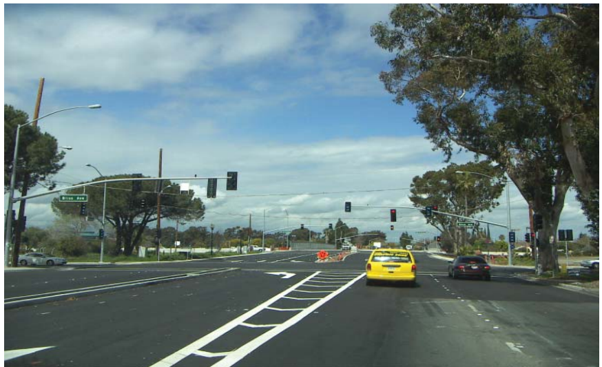
New traffic signals at the intersection of Railroad and Bliss Avenues help pedestrians cross the street, but visibility and pedestrian safety can be improved.
