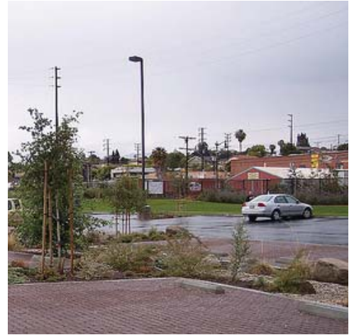
Permeable pavers in parking lots and other areas help improve drainage and can be an attractive screen for spaces.
