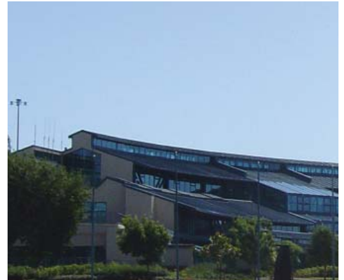
Pittsburg's City Hall is a major employer in the area, and a well-designed modern building that enhances the area.
