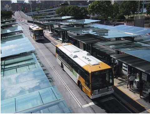
A bus access only lane provides a safe and comfortable environment for transferring from bus to eBART.
