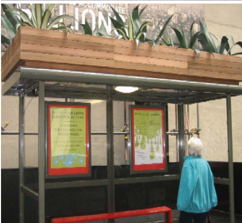
Bus shelters provide opportunities for artistic installations and public information kiosks.
