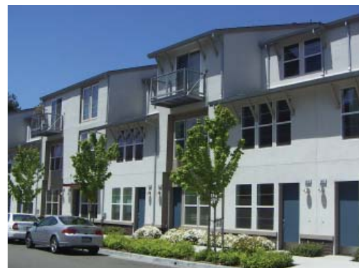
Upper-story balconies may also protrude from the building edge.
