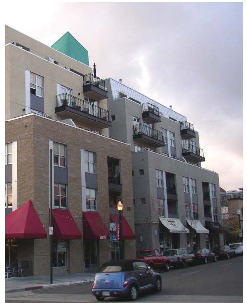
Upper-story setbacks mask a building's height and massing at the street level.
