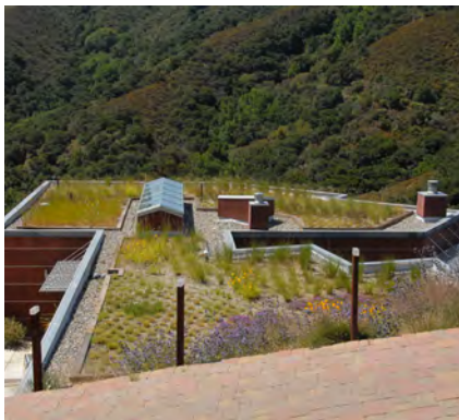
DG-42: Roof mounted photovoltaics are integrated architecturally (top). A green roof blends with nearby hills (bottom).
