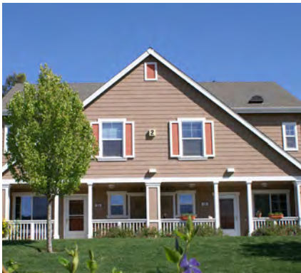
DG-11: Residential entrances can be accompanied by a covered porch, stoop, or veranda to shelter and clearly express the entrance.
