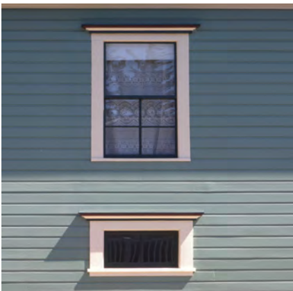
DG-20: Window trim adds to a building's visual interest and appearance.
