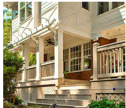
DG-17: These photos illustrate how knee bracing, columns and "exposed joists" can "visually support" other building features.
