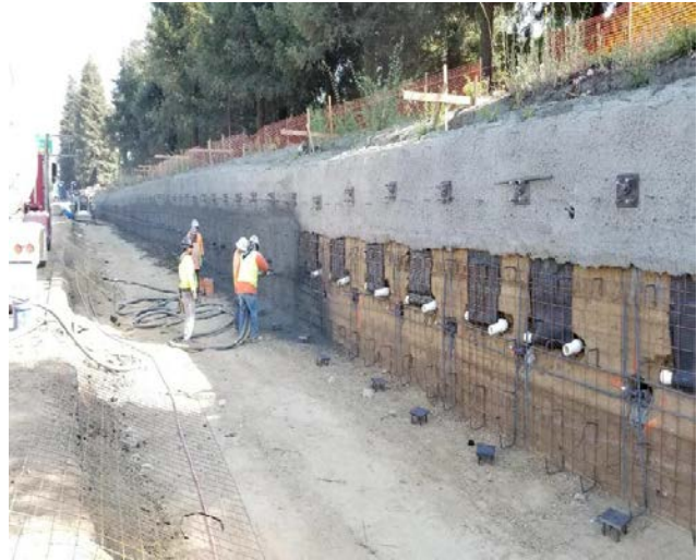
Shotcrete placement at soil nail wall, Hacienda Overcrossing
