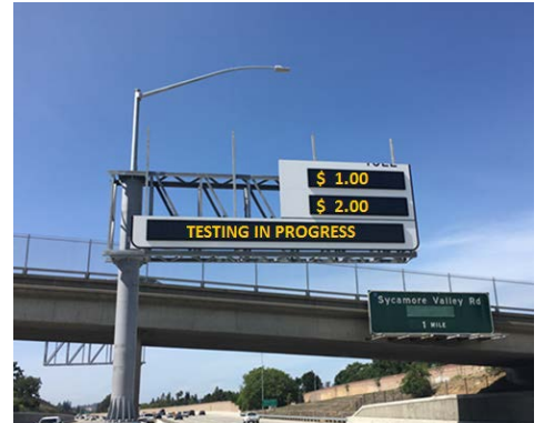
Mock-up of messages displayed on electronic signs for toll system testing during nighttime lane closures.
