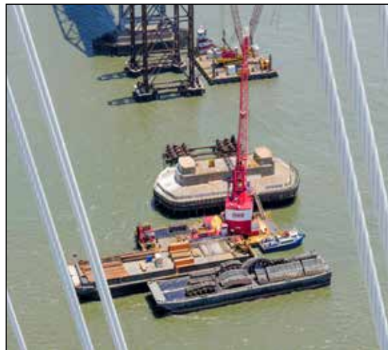
E3 Foundation Removal
