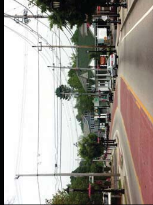
State highway shared center turn lane treatment: "Streetprint" colored and brick-textured asphalt topping (S.R. 114, Barrington, RI)
