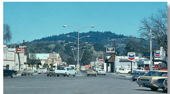
Exhibit H.3. Cloverdale Blvd Before Streetscape Improvements
