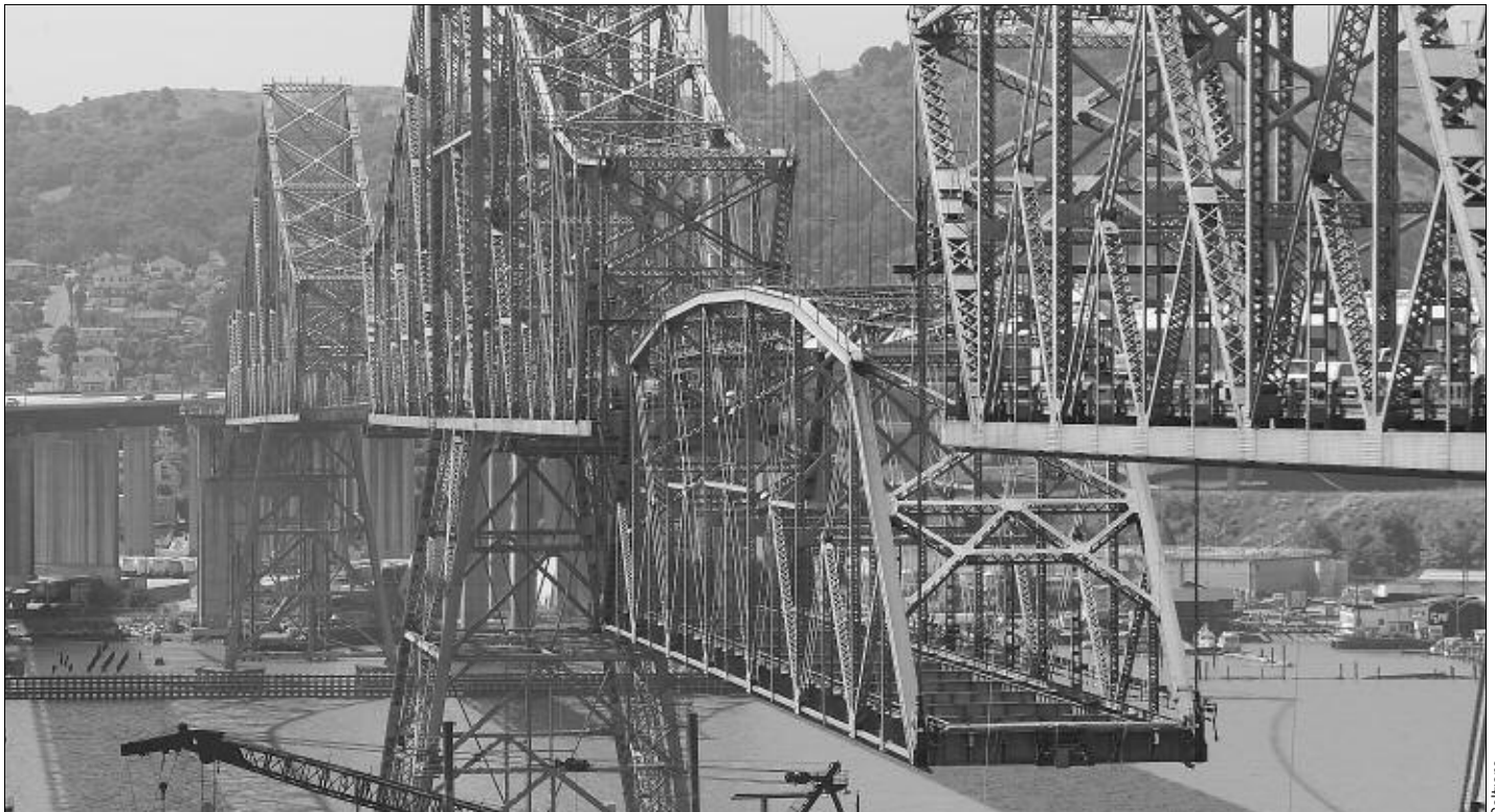
A section of the 1927 Carquinez Bridge is removed.
