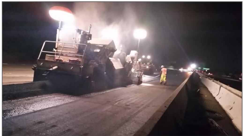
Construction crews grind and pave lanes closest to the median barrier.
