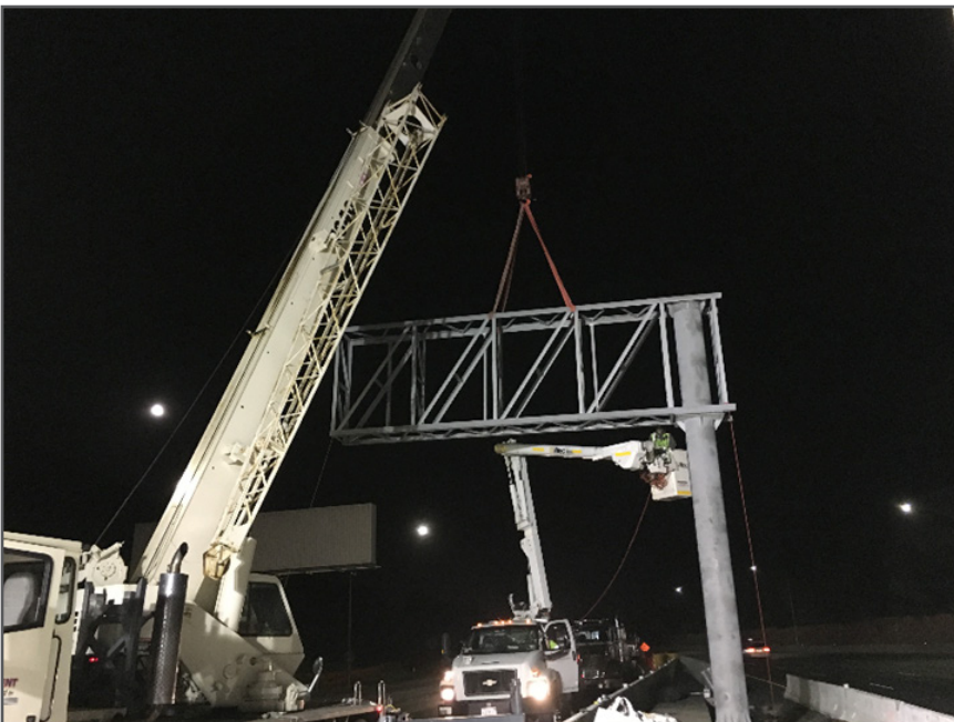
Construction crews install an overhead sign along I-680.
