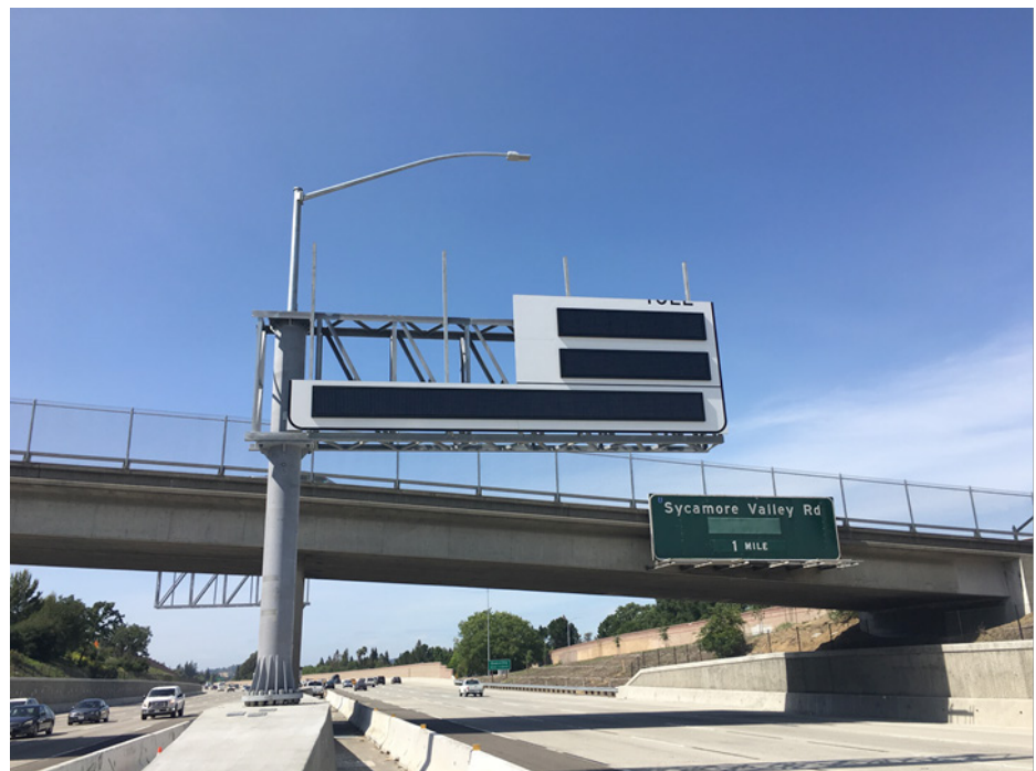
Partially installed pricing sign. (See additional construction photographs on pages 18-19)
