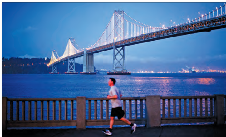
The north face of the West Span of the Bay Bridge has become the canvas for a nightly light show that dazzles locals and tourists alike.
