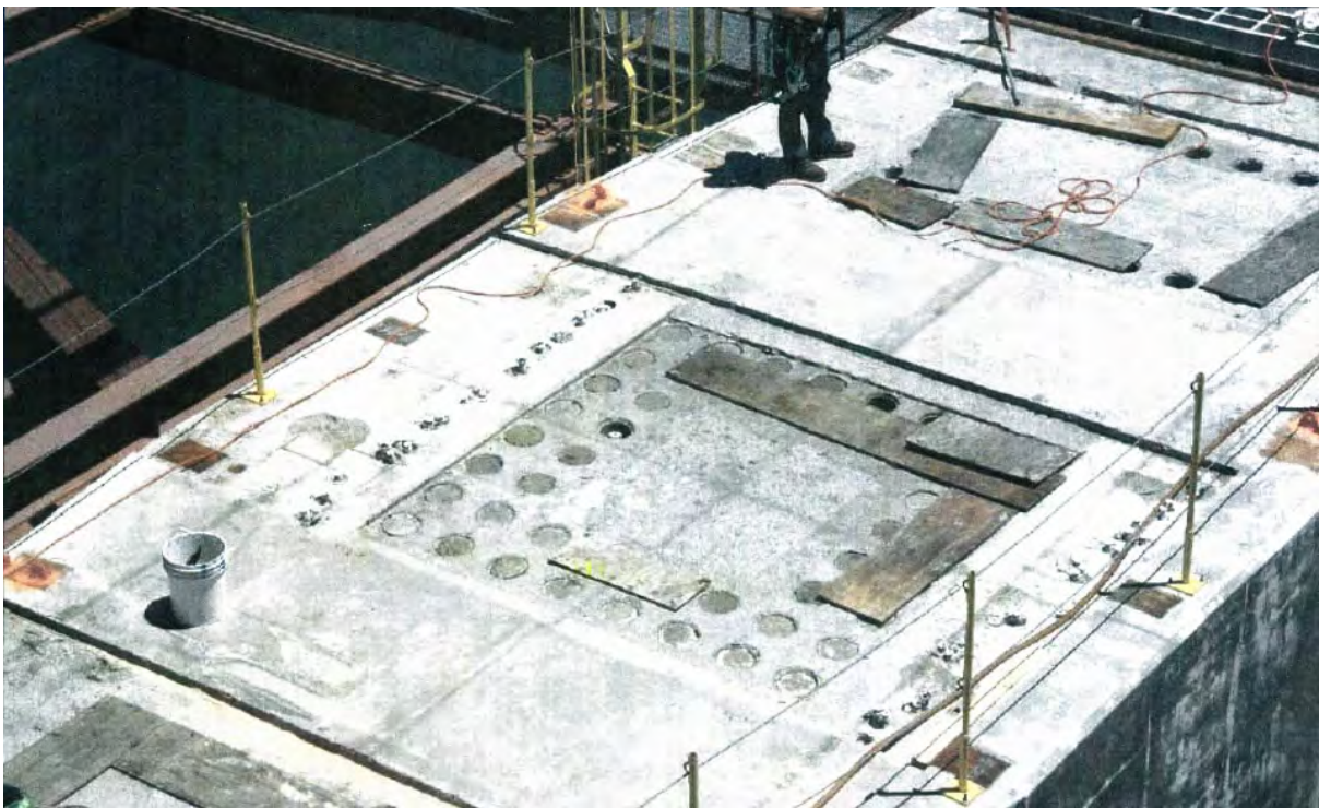
Figure 18 Pier E2 Cap Construction Photograph — Embedded rods are in holes
