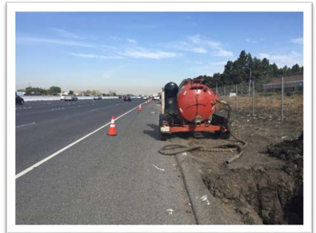
TOP: Rebar Cages for CIDH Pile Foundations BOTTOM: Directional Boring Equipment
