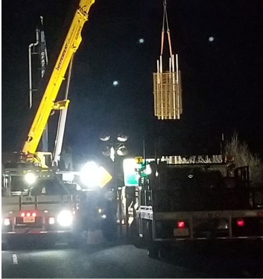
Setting reinforced steel cage for CIDH pile
