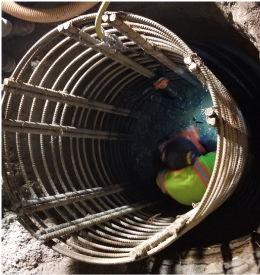
Preparing the top of the pile for sign-bridge pedestal
