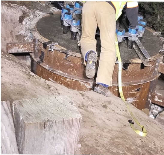
Finishing concrete on sign-bridge pedestal
