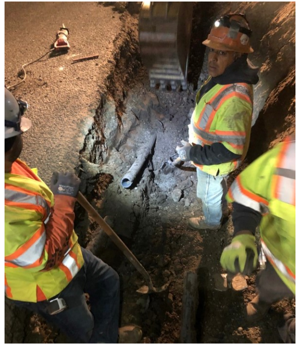
Installation of electrical conduit
