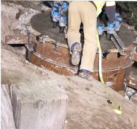
Finishing concrete on sign-bridge pedestal
