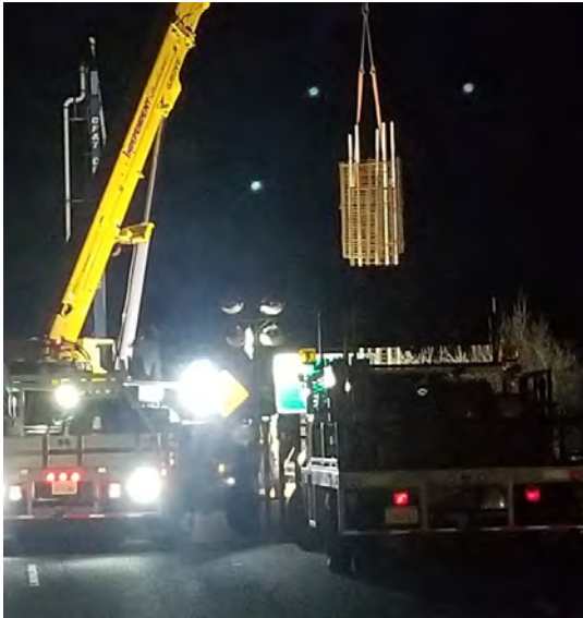
Setting reinforced steel cage for CIDH pile
