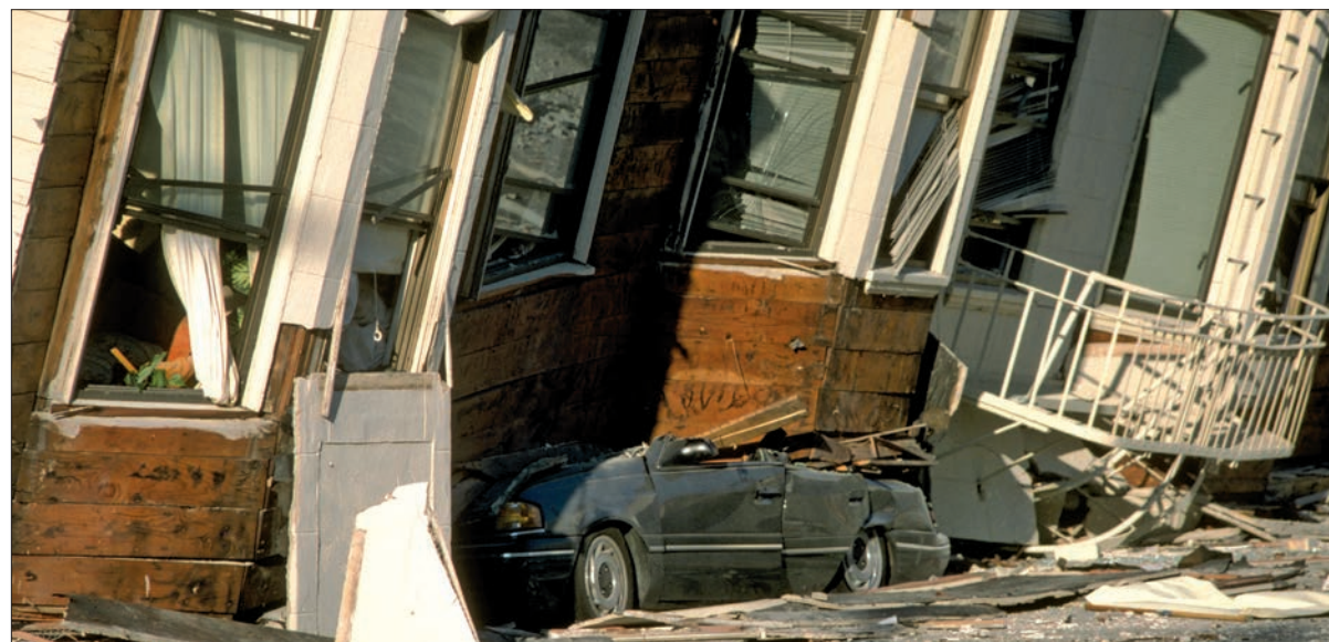
Damage from the 1989 Loma Prieta earthquake in San Francisco's Marina District
