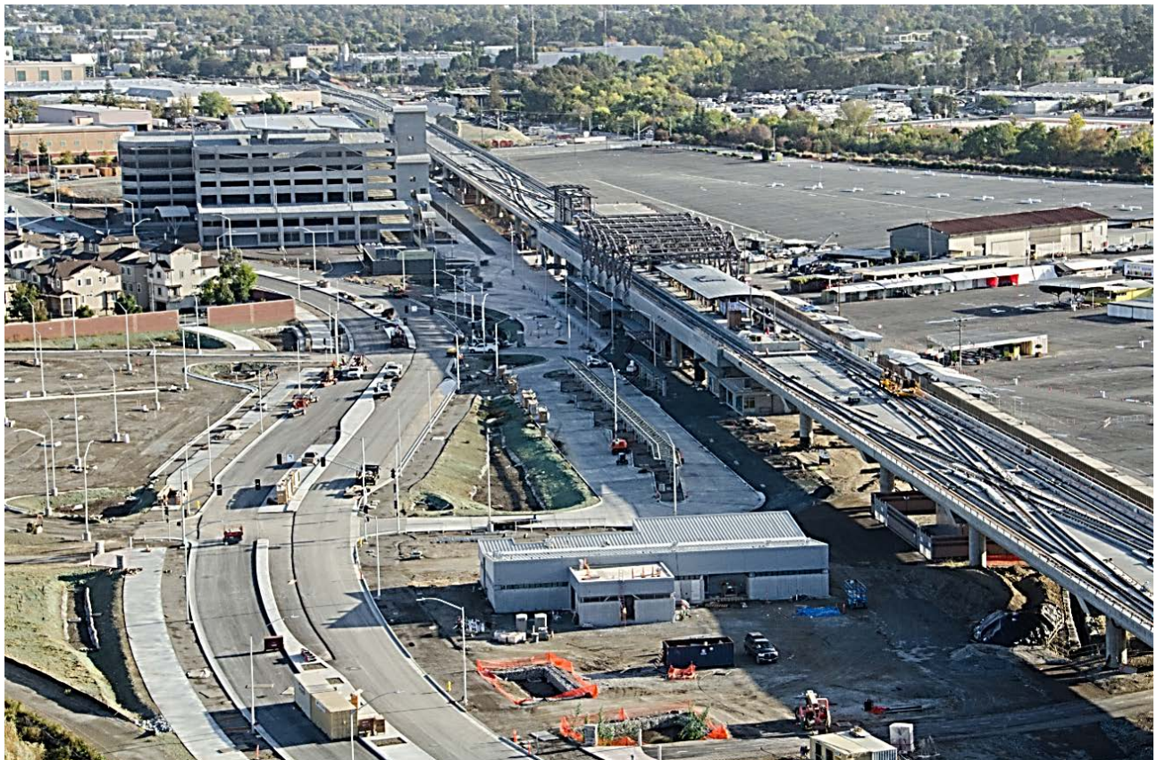
(VTA: BART to Warm Springs, Berryessa Extension)
