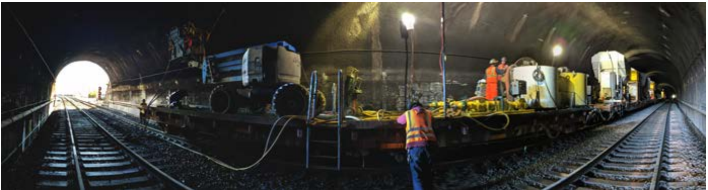
Construction of electrification infrastructure within rail tunnels in San Francisco (photo: Caltrain)
