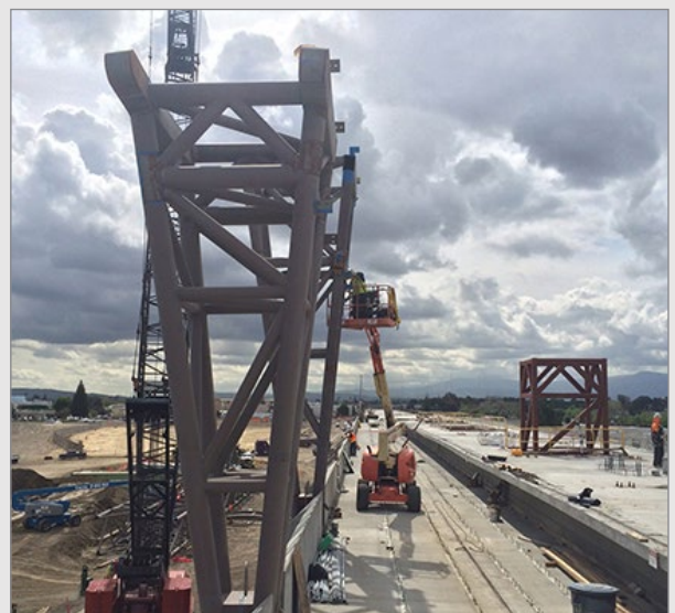
Construction of the new Berryessa BART Station. (Photo: Courtesy of VTA)
