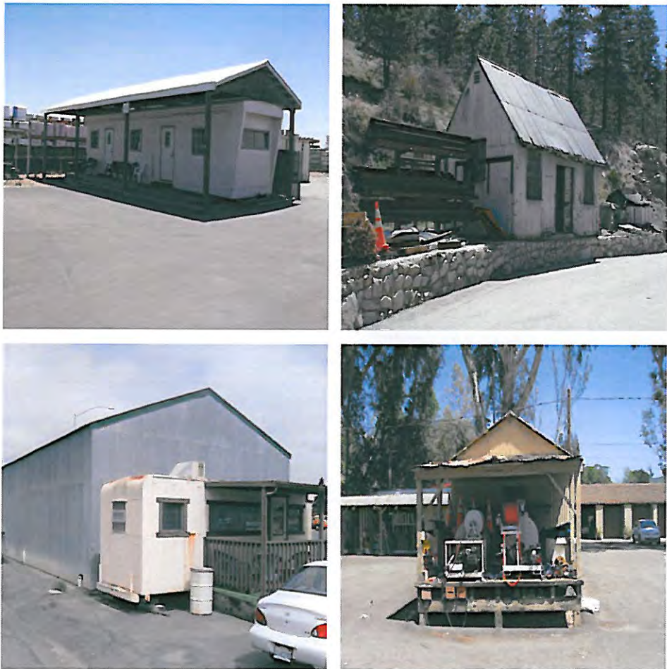
Maintenance facilities throughout the State are outdated and in need of modernization.
