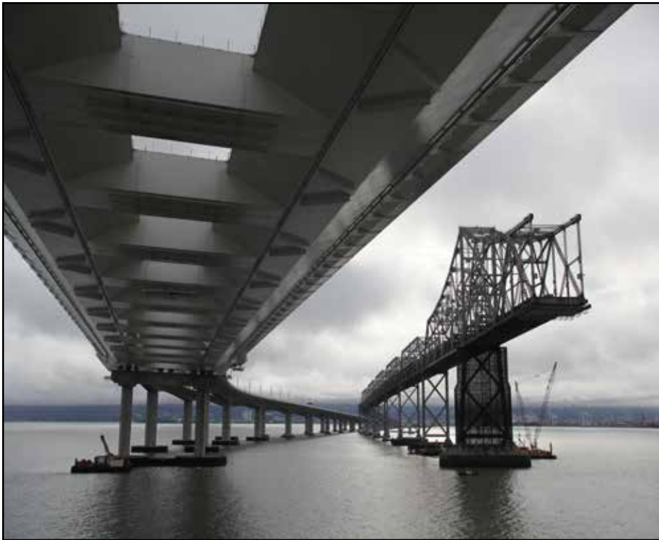
Underneath Cantilever Deck Removal in Progress Looking toward Oakland
