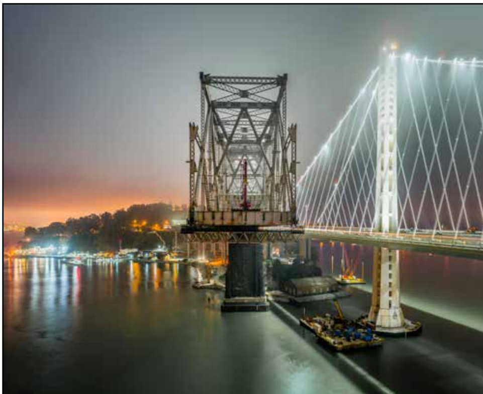
Demolition Progress of the Cantilever Section Looking toward Yerba Buena Island
