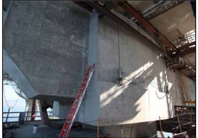
A View of the west Face of Pier E2W with S1 Shear Key Hold-Down Retrofit Complete
