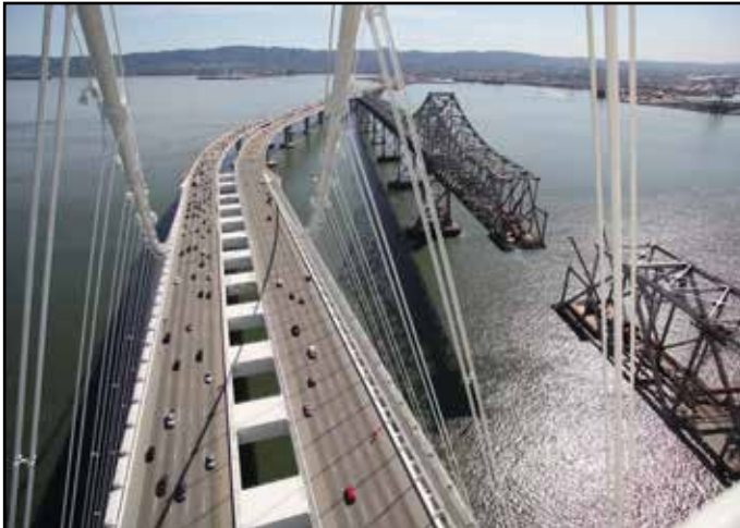
Self-Anchored Suspension Bridge and Demolition of Old Bridge
