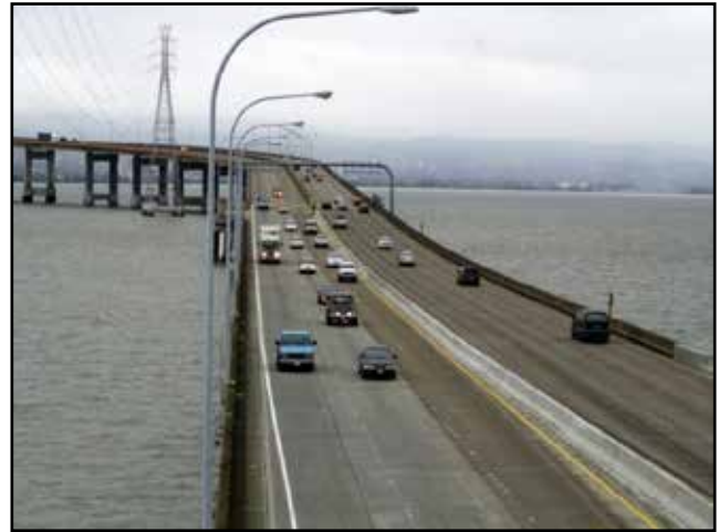
High-Rise Section of San Mateo-Hayward Bridge
