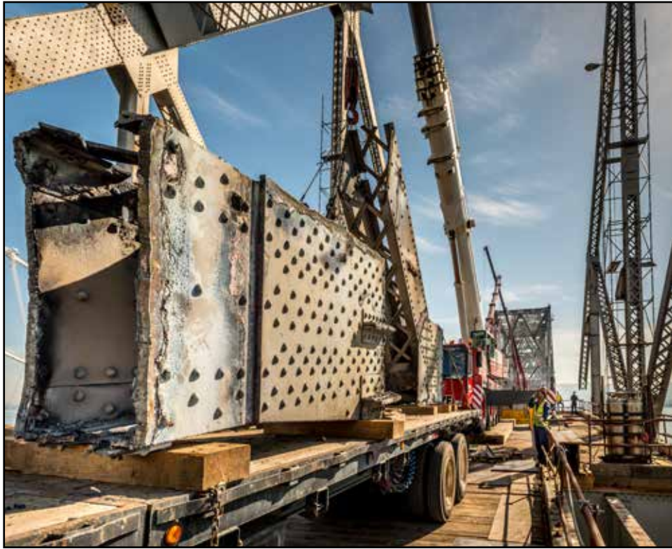
Removing Truss Member from the Cantilever Section
