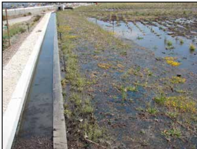
Stormwater Retention Basin
