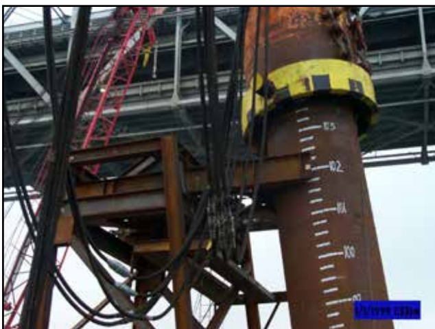
Battered Pile Installation Demonstration
