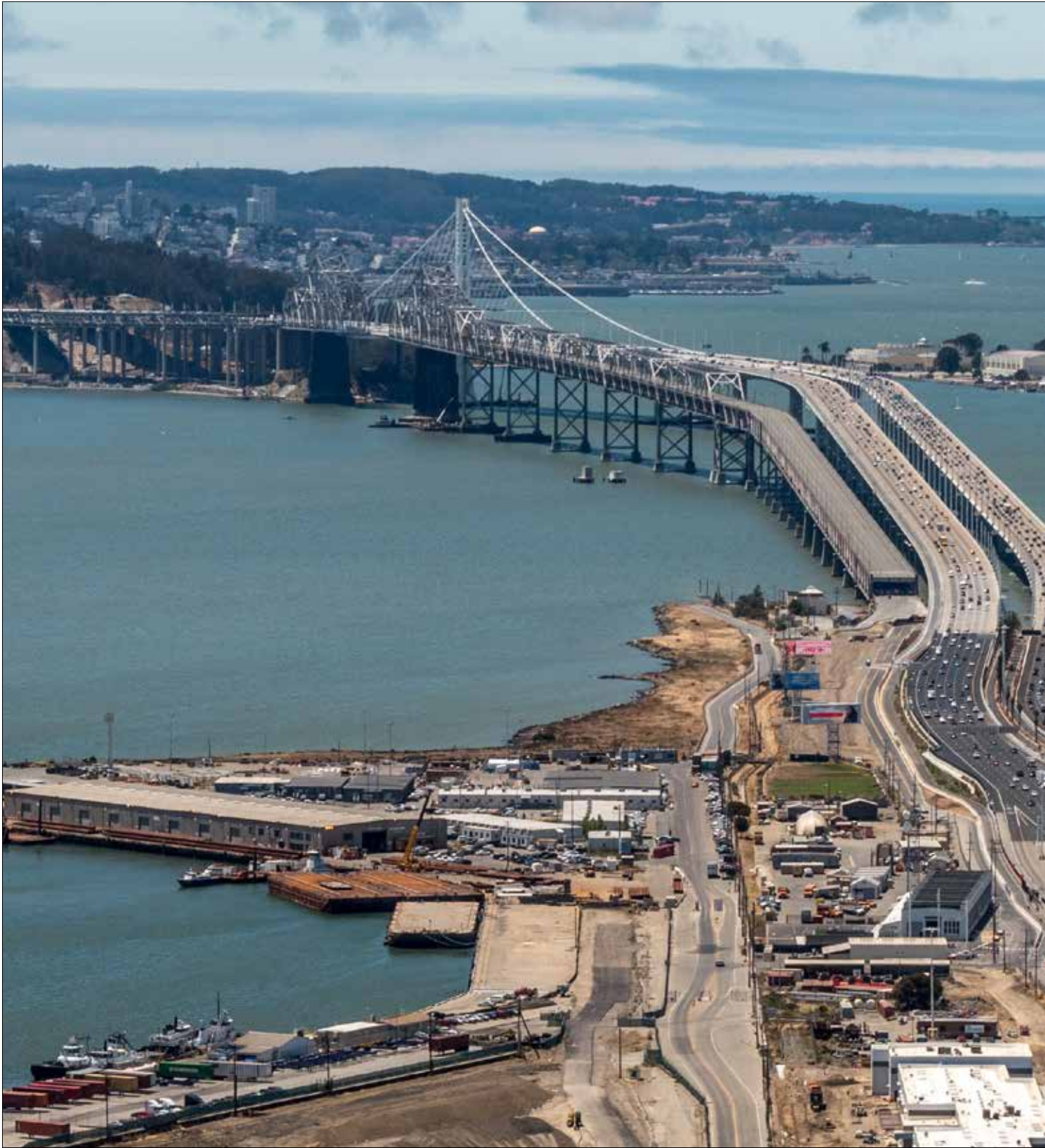
Aerial View of Oakland Touchdown Construction Progress
