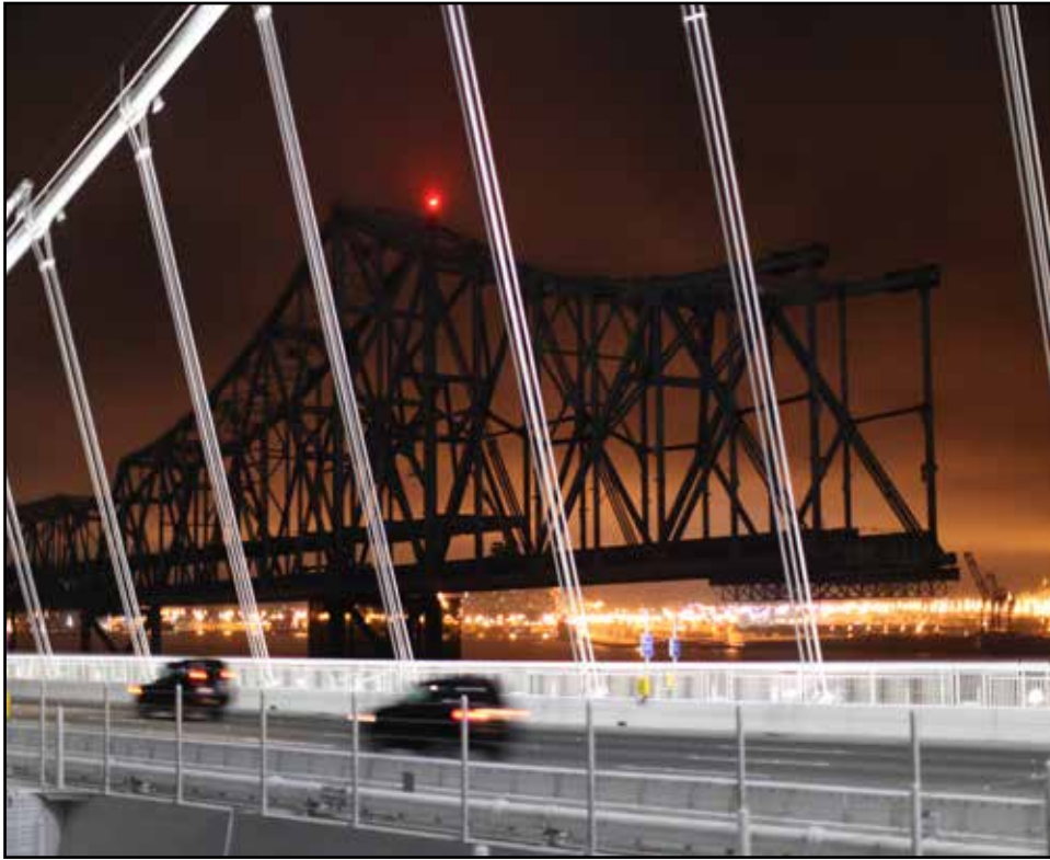
Contractors Have Removed over 200 Feet of the Original East Span
