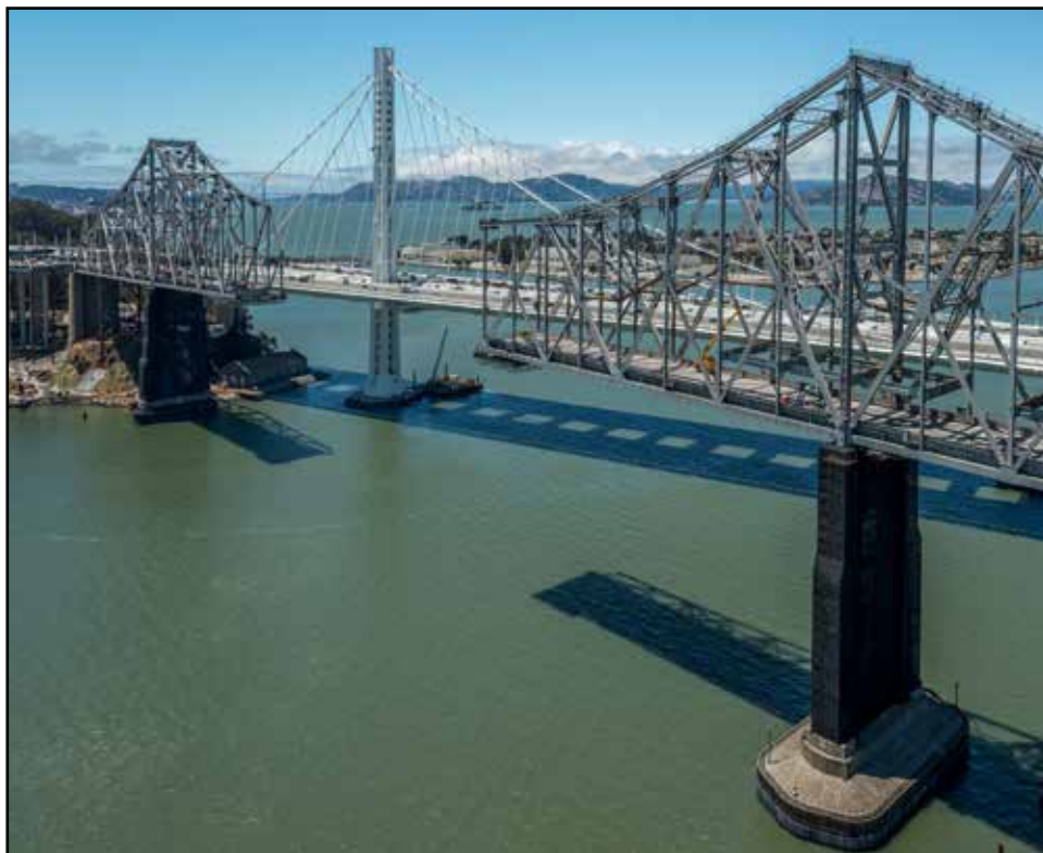
Demolition Progress of the Cantilever Section
