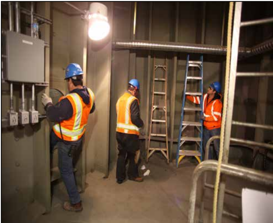
Tower Interior Cleaning
