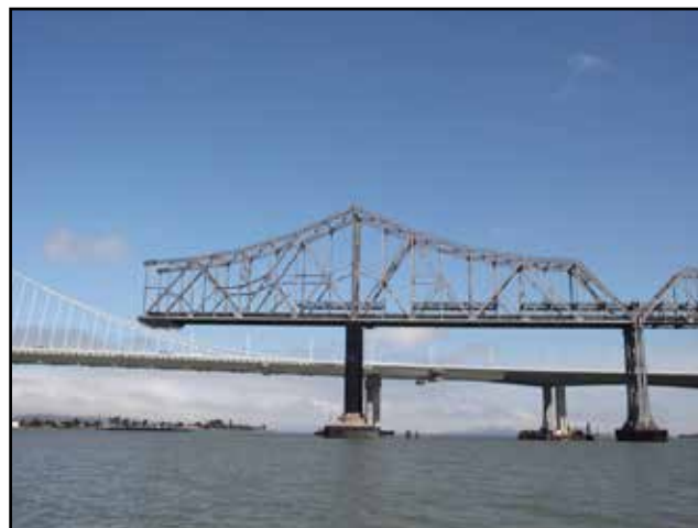
The existing East Span Cantilever Section of the San Francisco-Oakland Bay Bridge Being Dismantled
