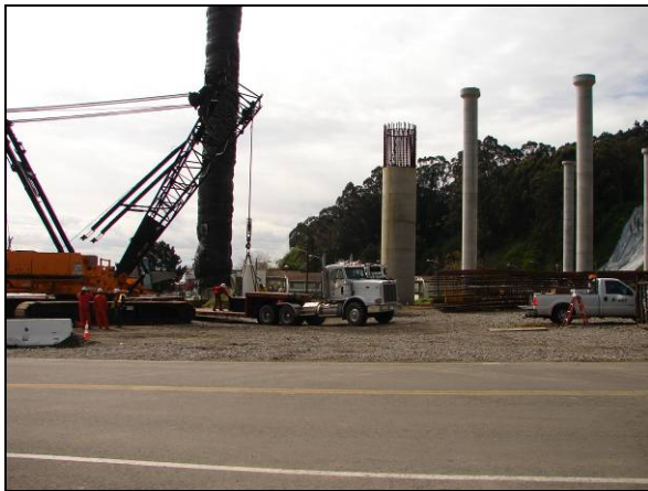
Demobilization of the SSD construction equipment 2
