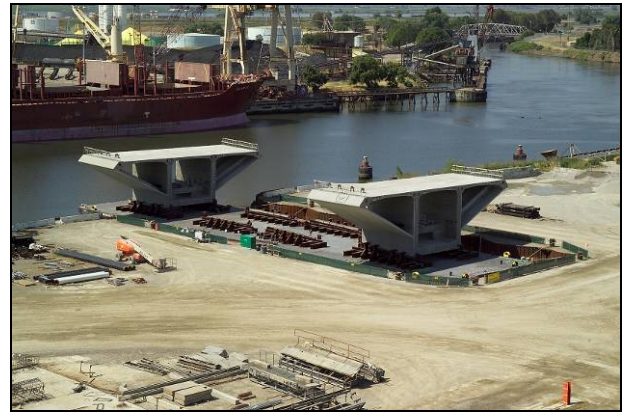
Precast deck segments at Stockton casting yard
