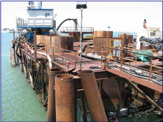
Pile driving at T1
