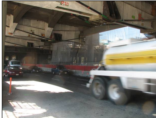
Temporary Support Frame (Super Bent at Bent #43) 3
