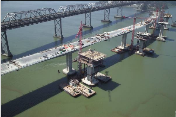
Pier Table 6W Nearing Completion
