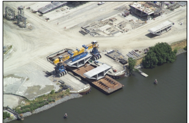
Precast deck segments ready for transport
