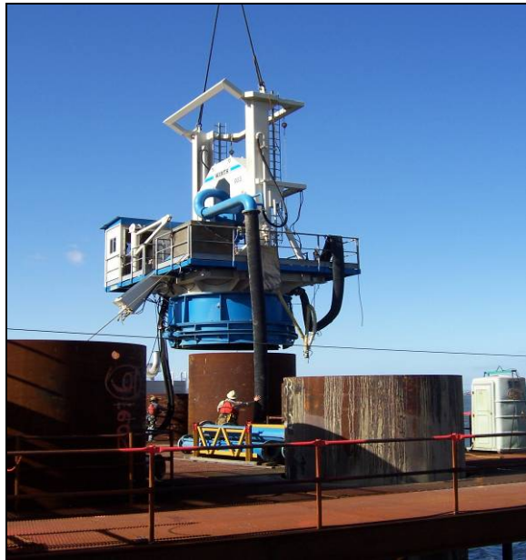
T1 Foundation –drilling for CIDH Piles
