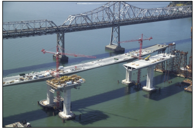
Aerial view of Skyway construction
