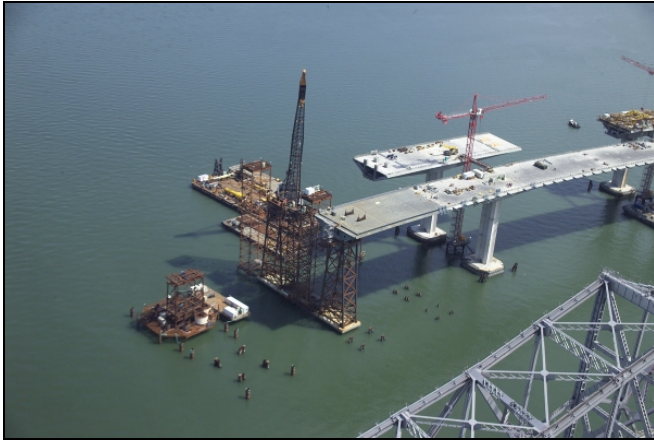
Western end of Skyway with adjacent E2 Foundation construction
