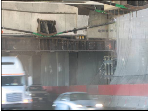
Temporary Support Frame (Super Bent at Bent #43) 1
