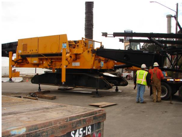
Demobilization of the SSD construction equipment 4
