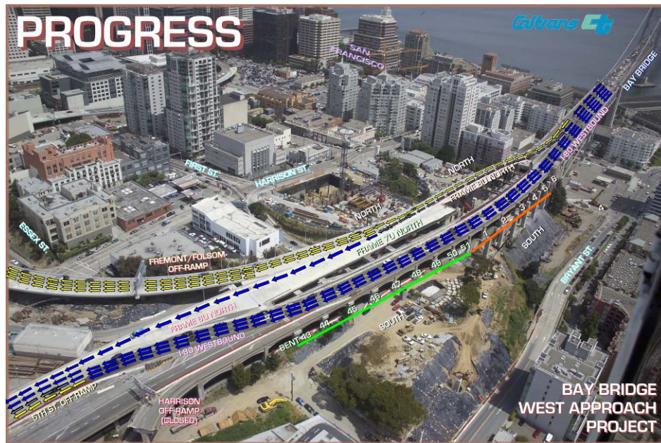
West Approach Project
