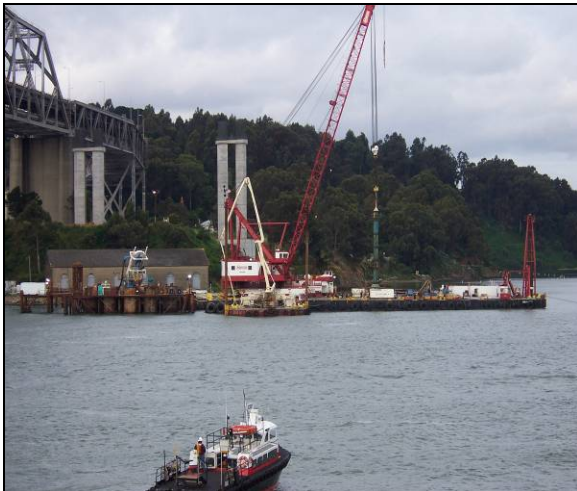
T1 Foundation-Drilling Operations for CIDH Piles
