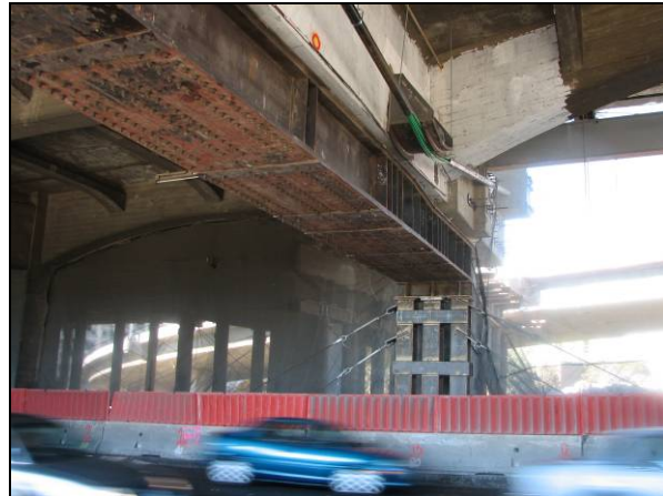
Temporary Support Frame (Super Bent at Bent #43) 4
