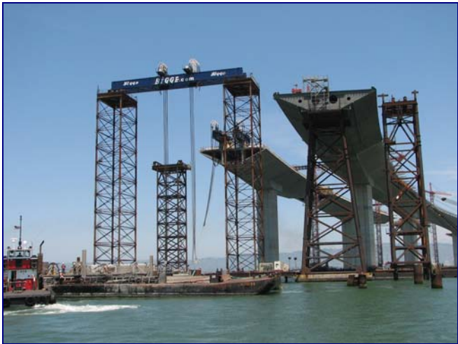
Temporary support for the orthotropic box girder - west
