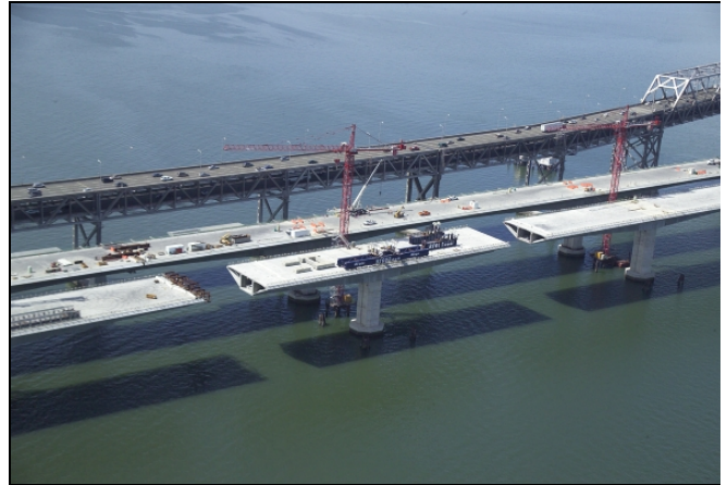
Deck segment at Pier 10 awaiting hinge pipe beam installation
