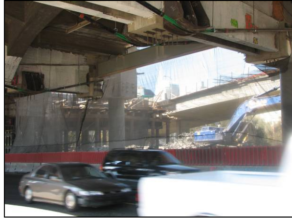
Temporary Support Frame (Super Bent at Bent #43) 2
