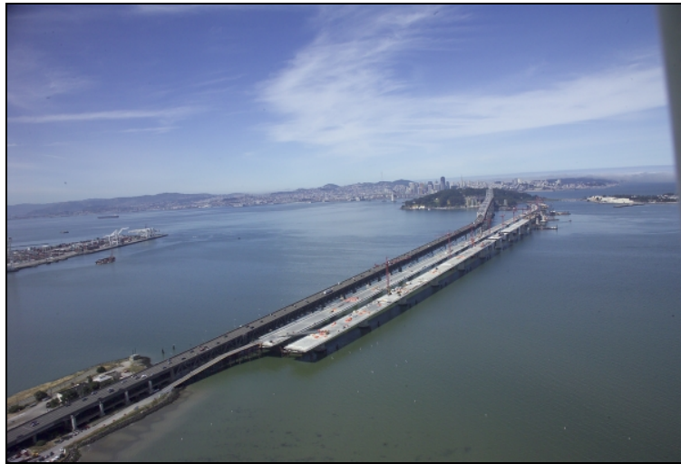
Aerial view of Skyway construction
