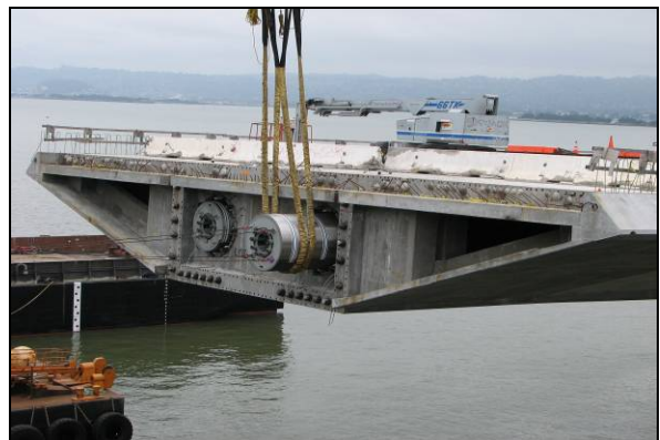
Skyway-5-5-06-Install of hinge pipe beams at Hinge DW
