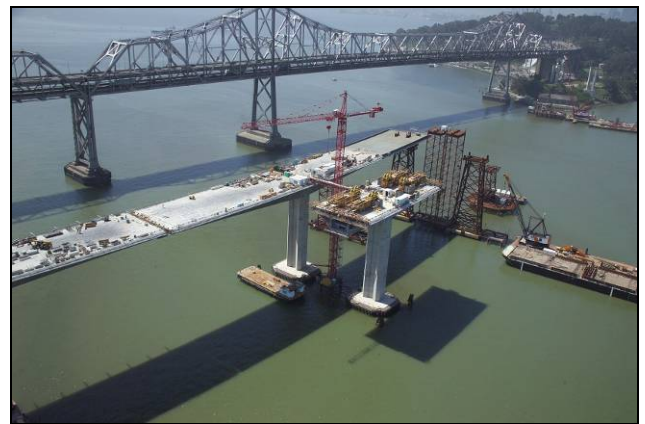
Aerial view of the western end of the Skyway contract
