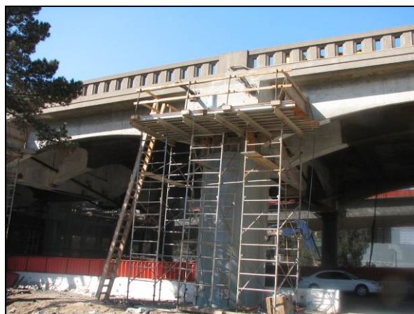
Demolition of Frame 7U North & 8U North over First St. On-ramp 1
