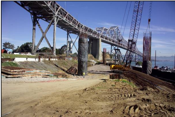
Pier Column Construction for Bents 50 and 51
