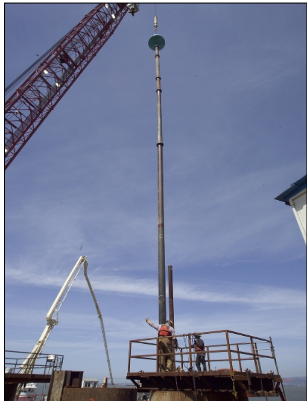
T1 Foundation-drilling operations for CIDH Piles
