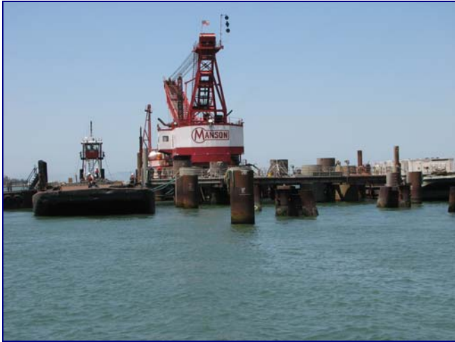
Pile driving at E2
