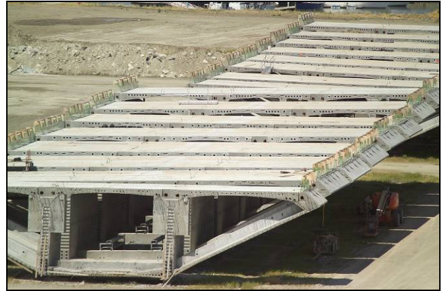
Precast deck segments at Stockton casting yard
