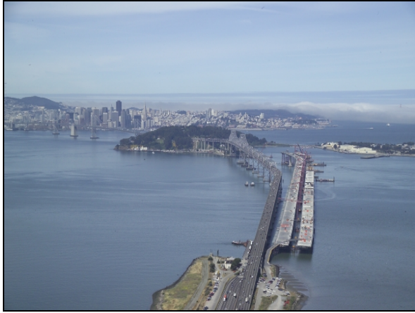
Aerial view of Bay Bridge East Span and new Skyway
