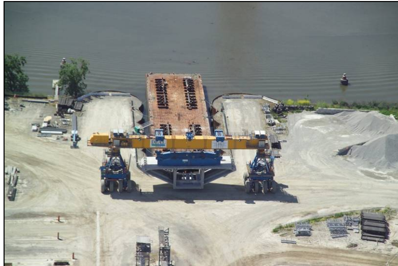
Precast segment Skyway deck ready for transport
