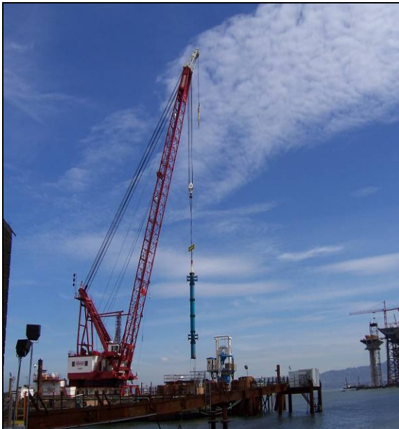
T1 Foundation-drilling Operations for CIDH Piles
