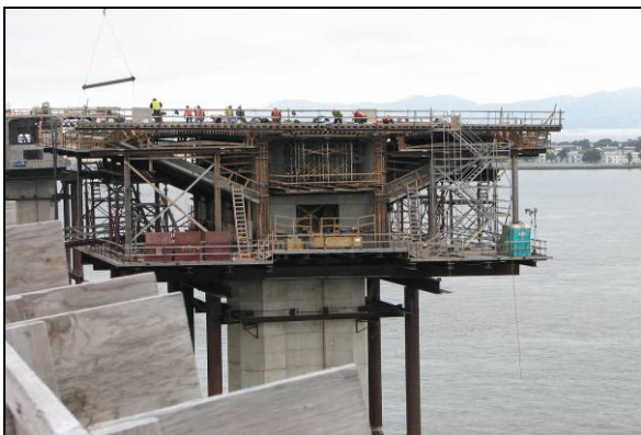
Construction of last remaining Skyway pier table (4W)
