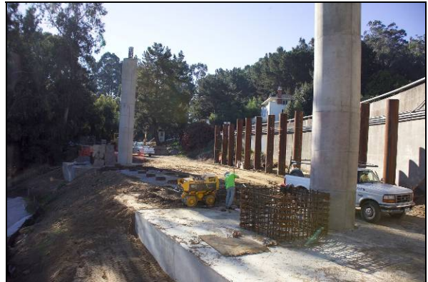
Footing and Pier Columns for Bent 48
