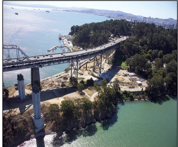
View of the completed W2 pier columns at the YBI, which will be the western support of the SAS structure
