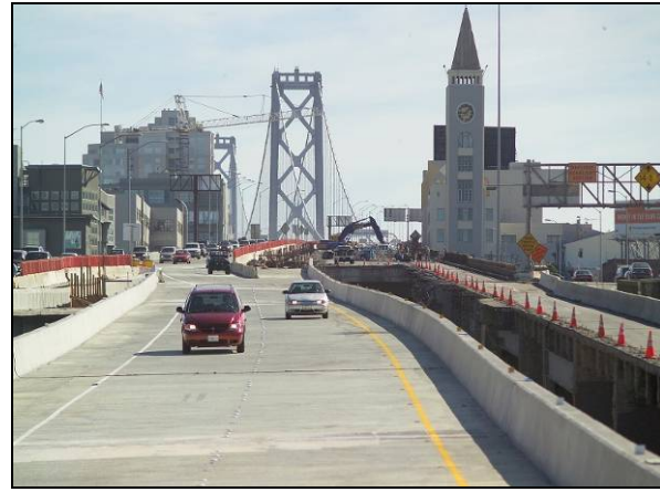
West Approach Project
