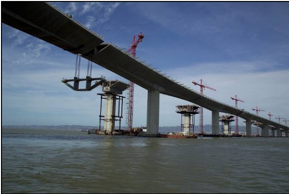
Installation of final precast segment deck for EB Skyway6
