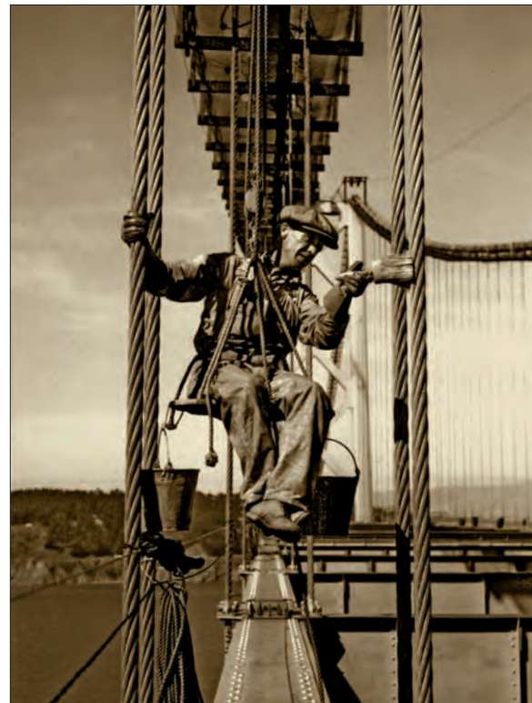
San Francisco-Oakland Bay Bridge
